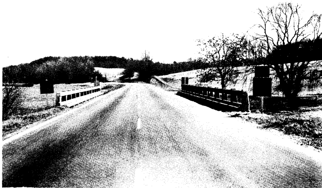
Figure 2. View of bridge #3 in Table IV showing excellent alignment and sight distance characteristics but the restricted roadway width and exposed ends of the rigid concrete railing constitute a potential hazard.
