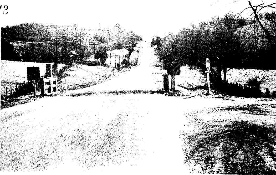
Figure 4. A narrow roadway with bridge located within a passing opportunity section of a two lane highway. An intersection is located to the right adjacent to the structures. (Bridge #1 of Table IV.)
