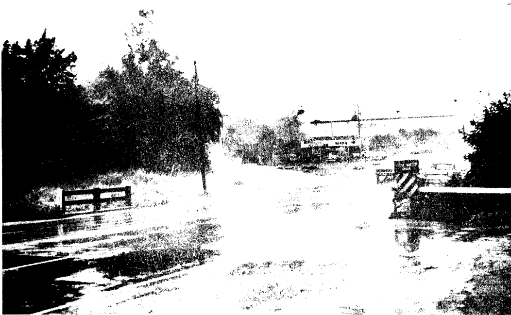
Figure 13. A narrow roadway width bridge located adjacent to an intersection (center) and business entrance (right foreground). A temporary wooden rail replaces the knocked out concrete rail on the right side of the bridge. (Bridge #24, Table IV.)
