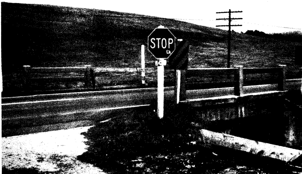
Figure 8. The same structure as shown in Figures 4 through 7. Here the south rail has been rebuilt; the east end of the north rail knocked out. (Date of accident — November 1970.)
