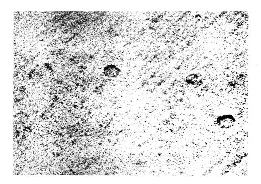
Figure 5. Close view of blisters in epoxy overlay with sand aggregate. Largest blister has a diameter of approximately 1".
