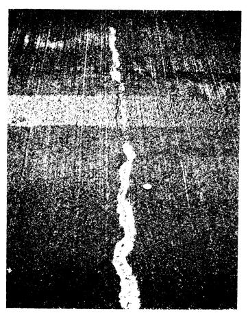
Figure 7. Typical separation of the overlay with a thin layer of concrete attached, adjacent to a reflective crack in the grit strips on the Occoquan Creek bridge.
