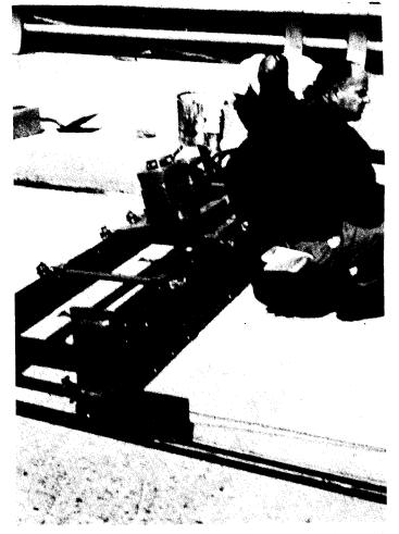
Figure 10. Screed used to finish the top surface of the Guardkote 250 mortar overlay.
