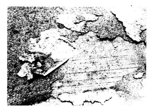
Figure 4. Area of delamination in the Shell MRAX strip with aluminum oxide grit on the Ramp C bridge.
