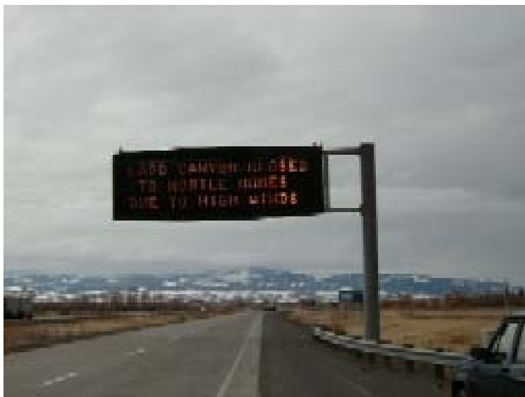
Figure 5.4: Variable message sign
