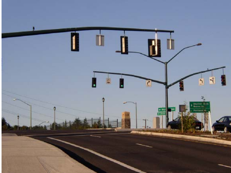
Figure 5.3: Signal mast arm with support pole in Portland, OR
