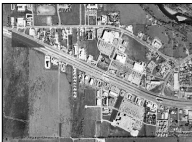
SH 71 Bastrop – after improvement
