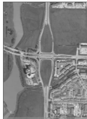
Preston Rd. - Legacy Pkwy. Grade Separation, Plano
