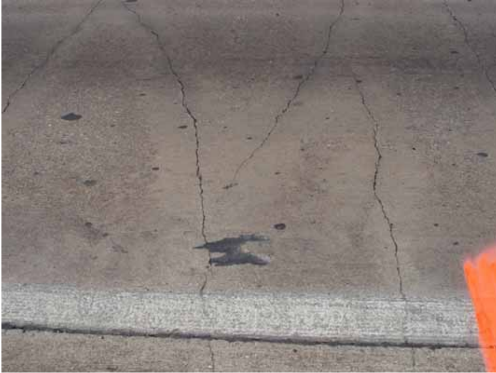
Figure 6.34: Non-milled, old concrete pavement texture on IH-35 in Waco
