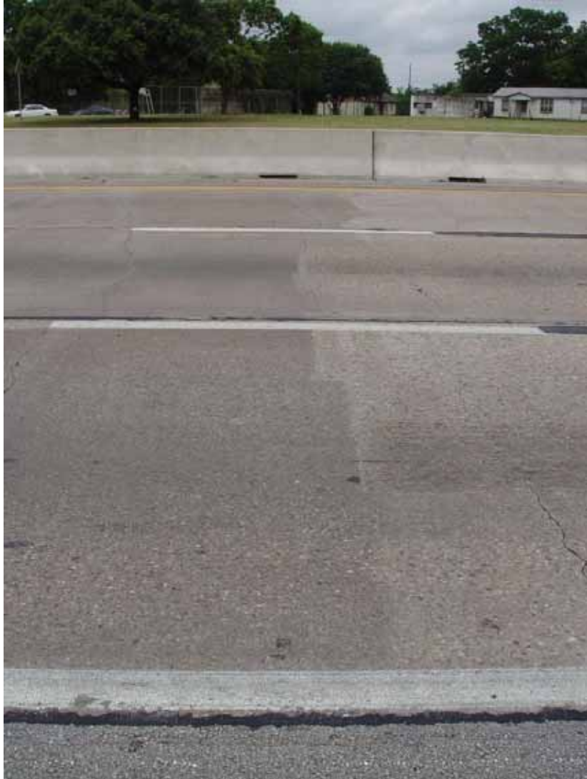
Figure 6.29: Beginning of IH-35 northbound diamond-ground section in Waco
