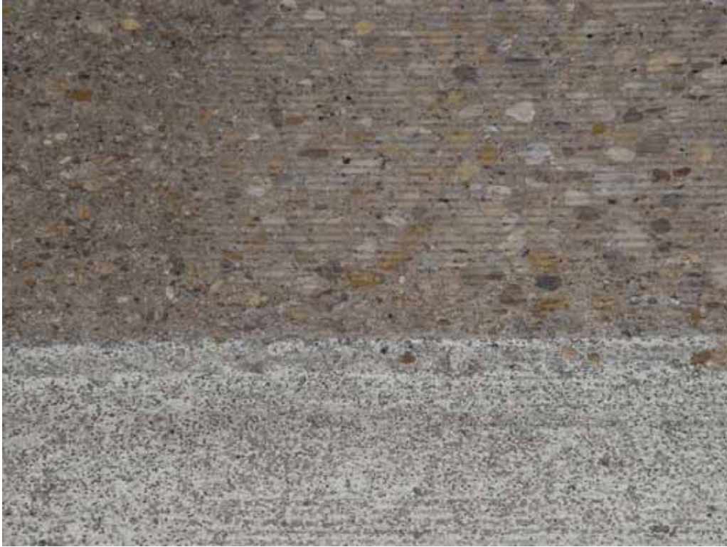
Figure 6.30: Texture of the diamond-ground section on IH-35 in Waco
