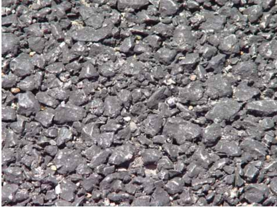
Figure 6.5: Texture of the new PFC overlay on IH-30 in Dallas
