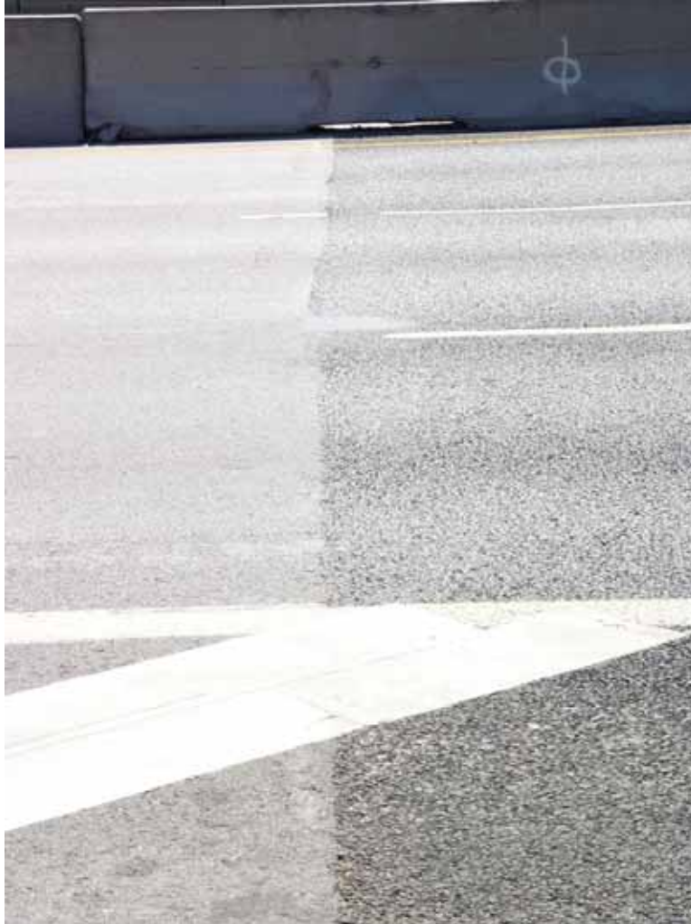
Figure 6.6: Westbound transition to new PFC overlay on IH-30 in Dallas
