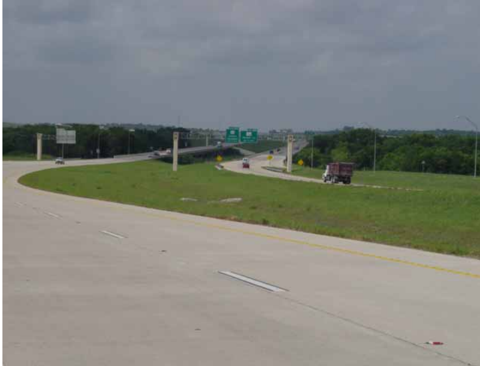
Figure 6.12: View of SH 130
