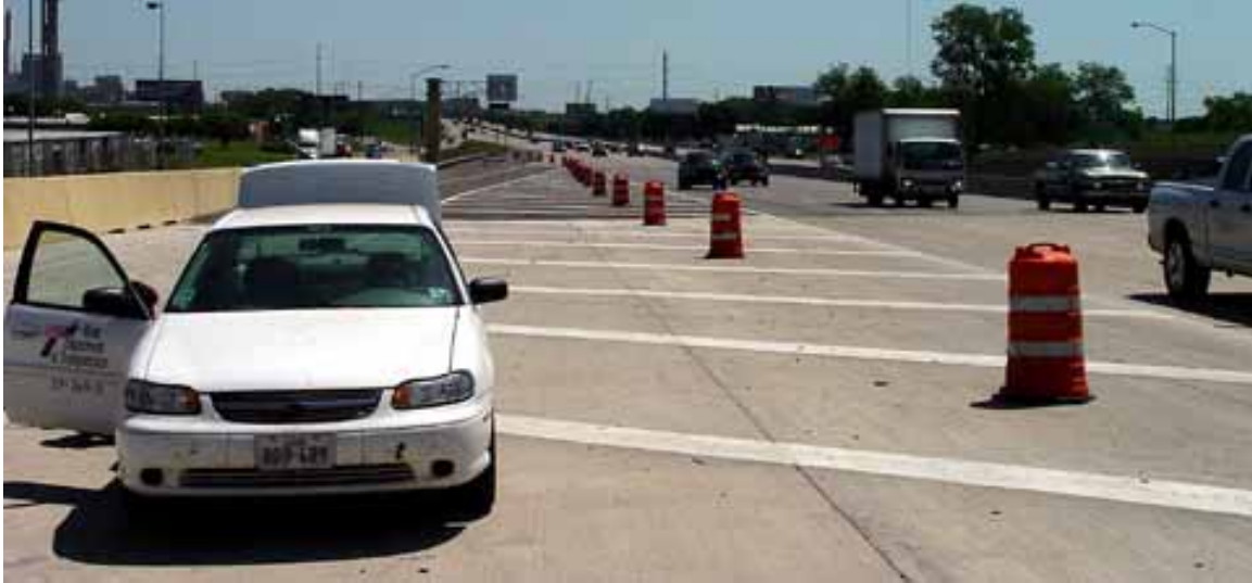
Figure 6.2: Beginning of IH-30 CRCP westbound section
