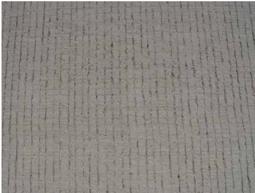
Figure 6.13: Uniformly transversely tined CRCP on SH 130 in Austin
