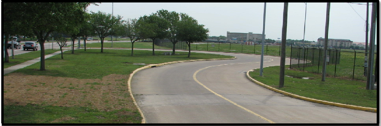
Figure 28. Facility Access Road That Allows Trucks to Straighten Before Approaching Intersection With Street.
