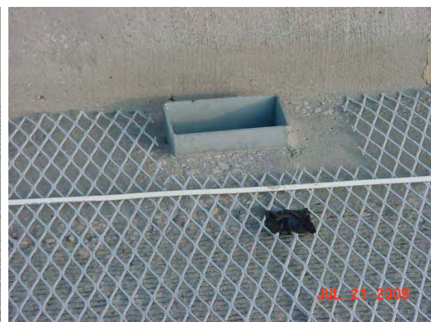
Figure 2 &3: Anode electrically connected to each other with metal clamps at each corner of 4' x 8' sheet. (Black patch is insulation around clamps to keep out concrete during placement.). White anode lead wire is connected to sheet in two locations. Anode was cut to fit around steel deck drains so it won't short out to the rebar.
