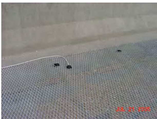
Figure 2 &3: Anode electrically connected to each other with metal clamps at each corner of 4' x 8' sheet. (Black patch is insulation around clamps to keep out concrete during placement.). White anode lead wire is connected to sheet in two locations. Anode was cut to fit around steel deck drains so it won't short out to the rebar.
