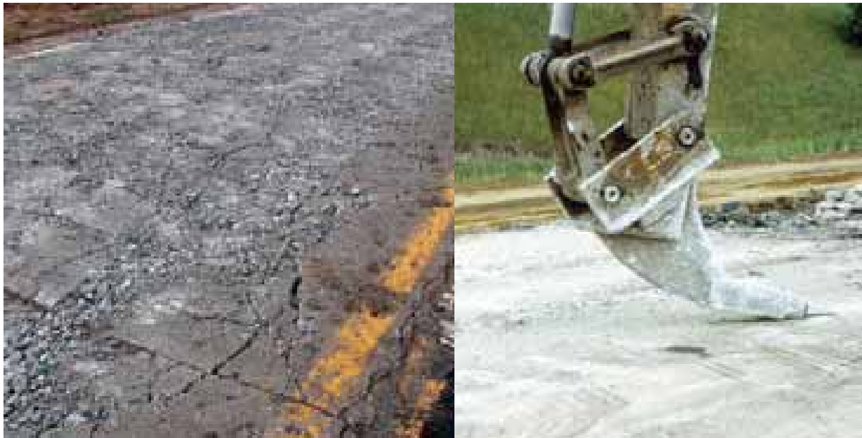
Figure 2-2. Typical concrete pavement break pattern before removal (left) and Rhino horn attachment for use in separating concrete for removal (right) after (ACPA 2009).
