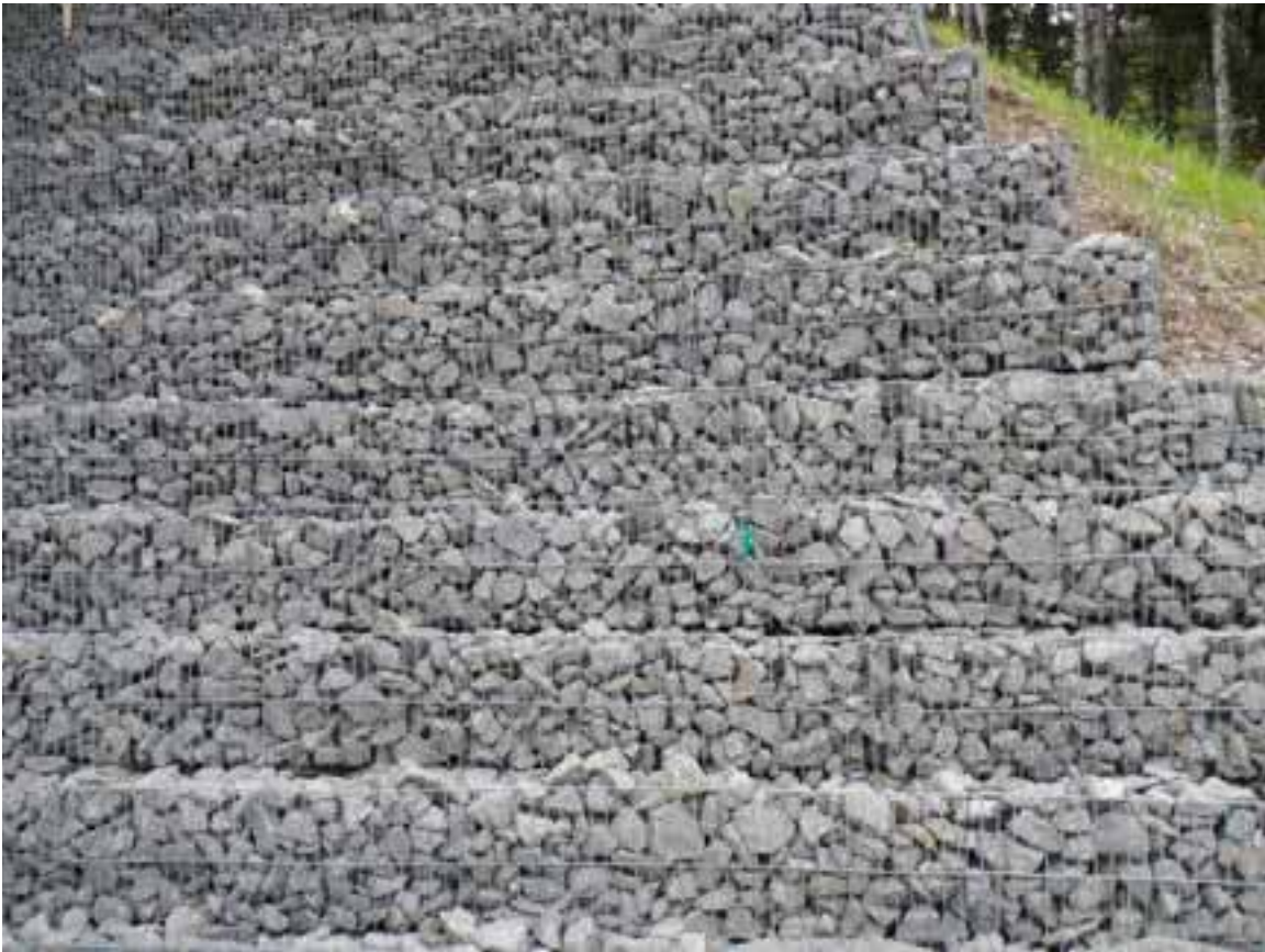
Figure 2-11. Wire gabion retaining wall structure.
