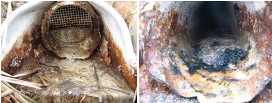
Figure 5-2. I-69 east of Flint; (left) partially plugged rodent screen; (right) blast furnace slag sludge behind screen.
