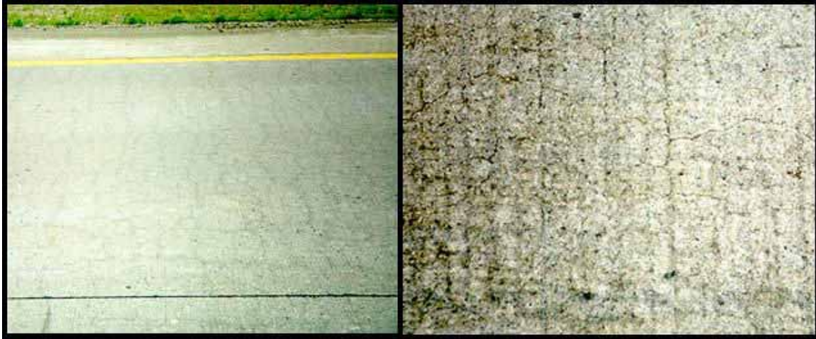
Figure 2-16. Concrete pavement containing RCA as aggregate on I-94 WB, West of Kalamazoo.
