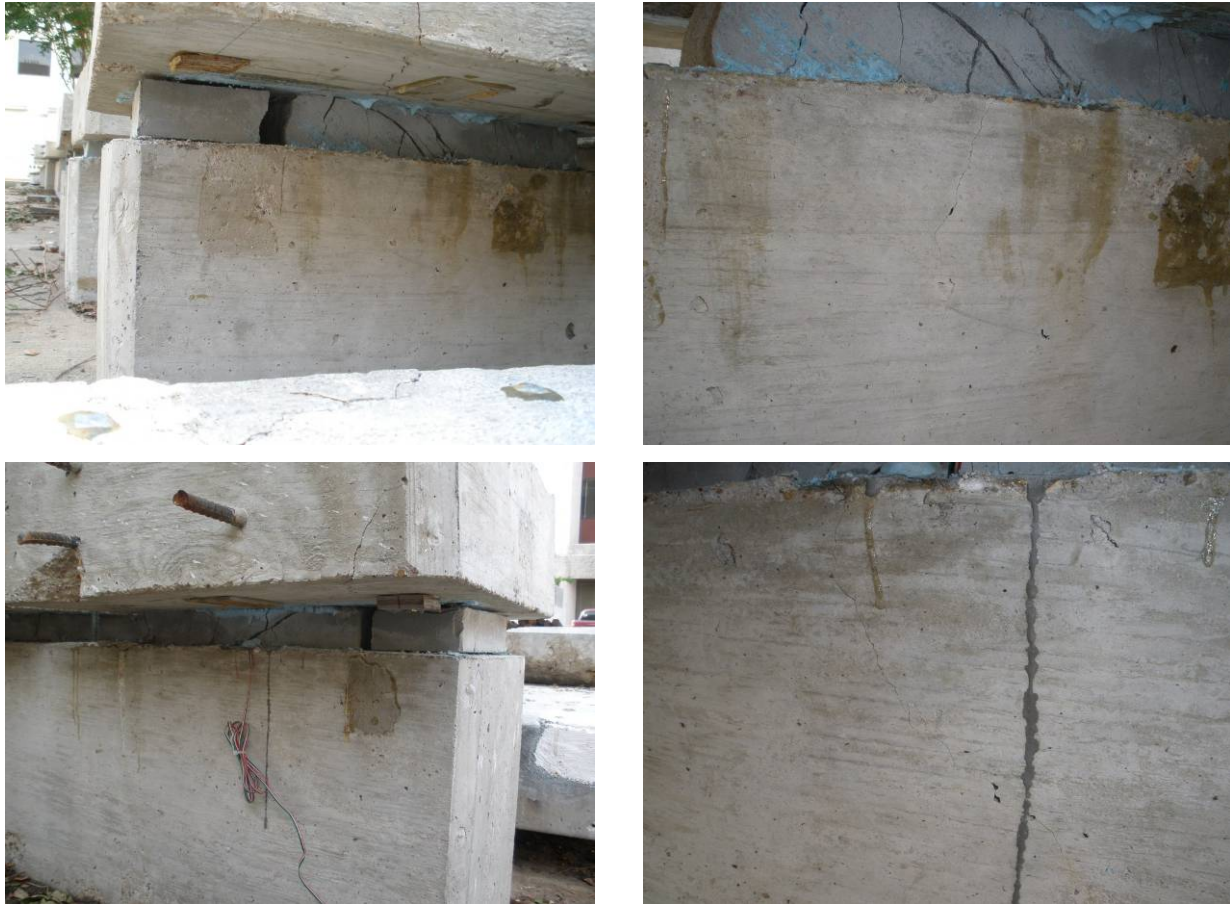
Figure 3-33. Photographs of 2_TR_2.0_B after Testing.
