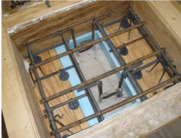
Figure 3-9. Photograph of Typical Reinforcing Layout of a CIP Shear Test Deck Specimen.
