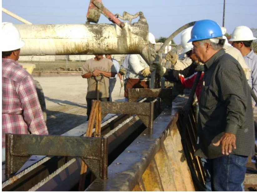
Fig. 7.5. Casting of PSFC I-Beam
