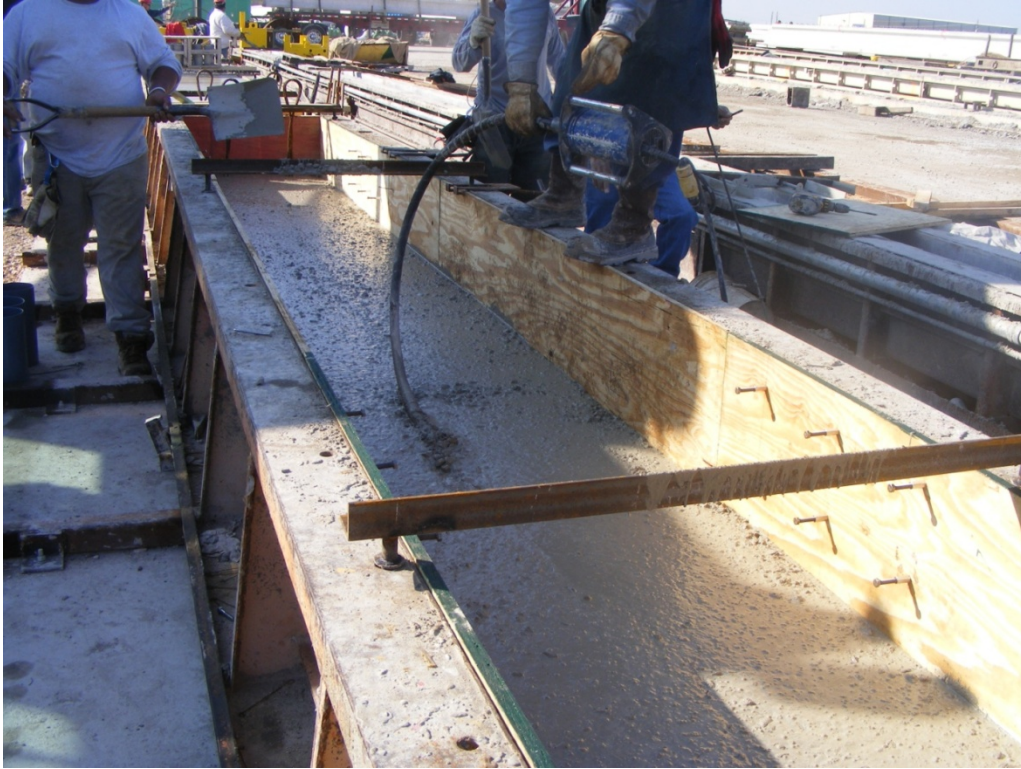
Fig. 8.4 First-Stage Concrete Compaction using Spud Vibrators in PSFC Box-Beams
