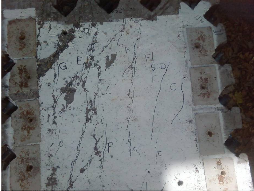
Fig. 6.2 Crack Pattern in PSFC Panel TAF-2
