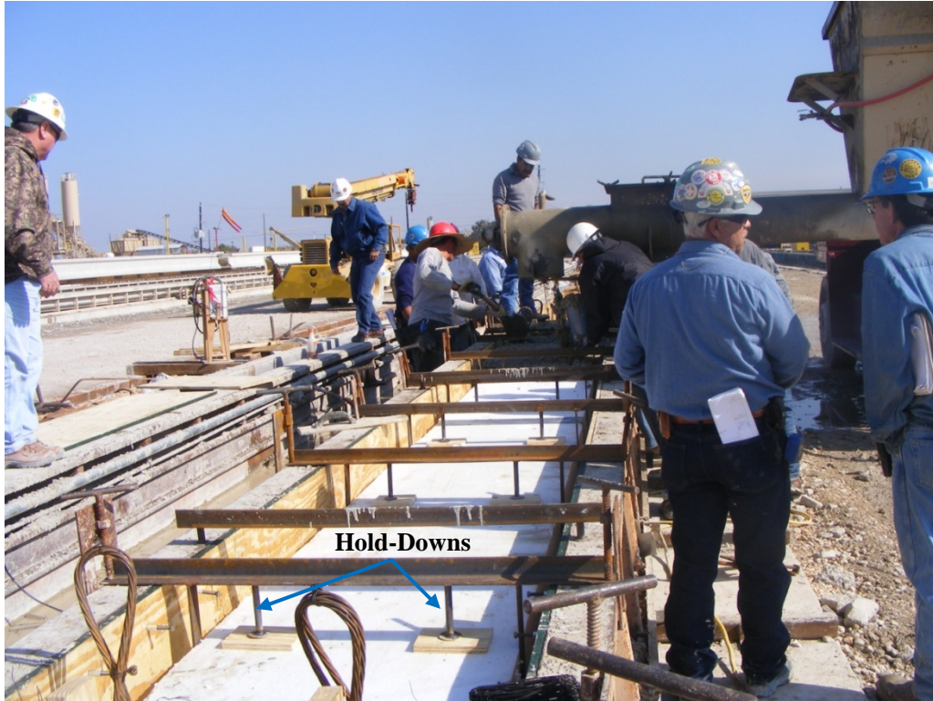
Fig. 8.5 Placement of Styrofoam after First-Stage of Concrete Casting in PSFC Box-Beams
