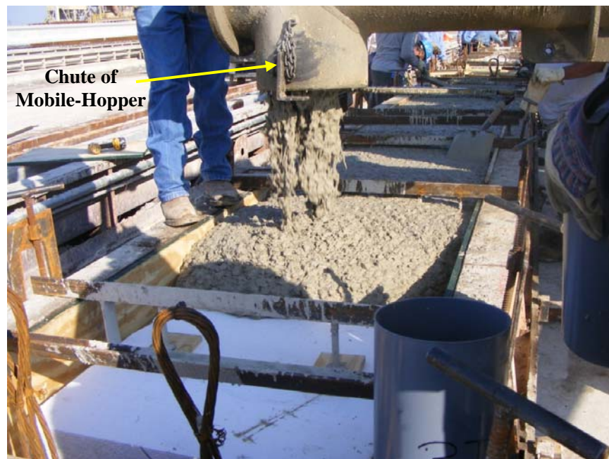
Fig. 8.3 Casting of PSFC Box-Beams
