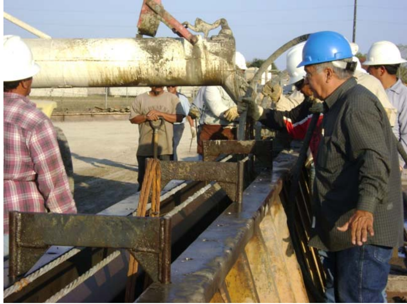
Fig. 7.5. Casting of PSFC I-Beam
