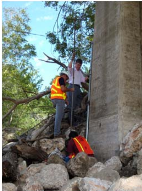
Figure E-13. Installation of the TBS Using a Hand-Auger.
