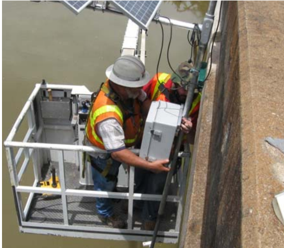
Figure 5-11. Mount the Master Station.
