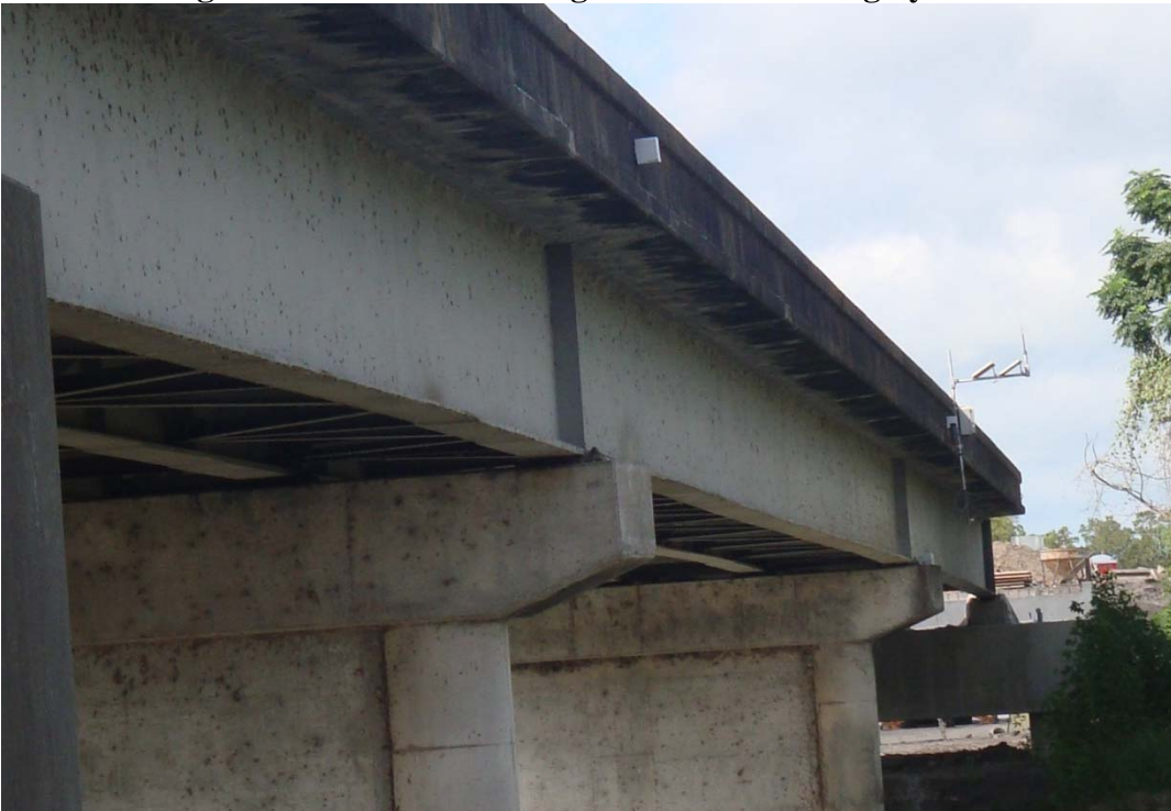
Figure 5-29. Modified Bridge Scour Monitoring System.
