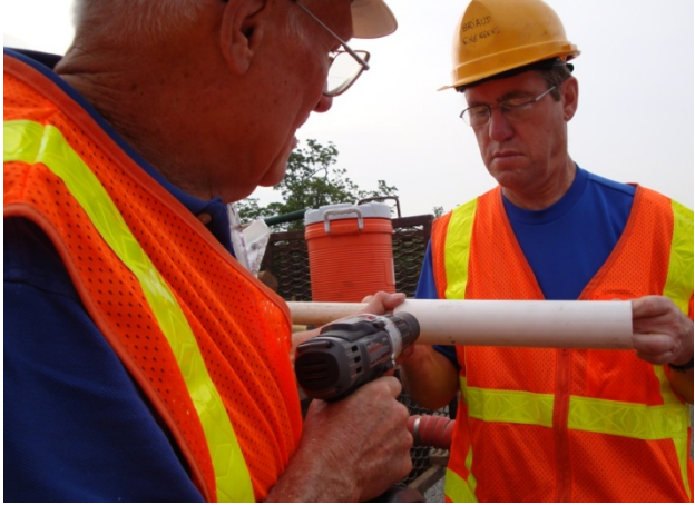
Figure D-22. PVC Pipe as an Extension of the Float-Out Device.
