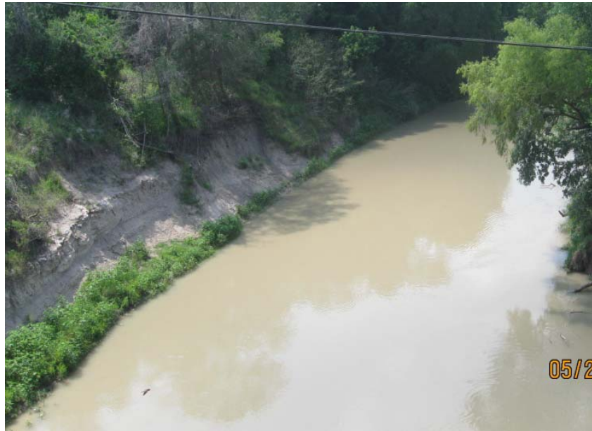
Figure E-9. Northern Bank of San Antonio River (Downstream of the Bridge).
