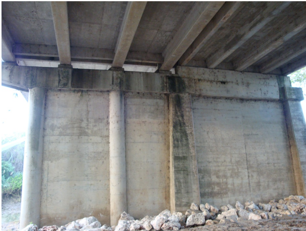
Figure 6-5. Compound Web-Wall on the Main Bridge Span (P1).
