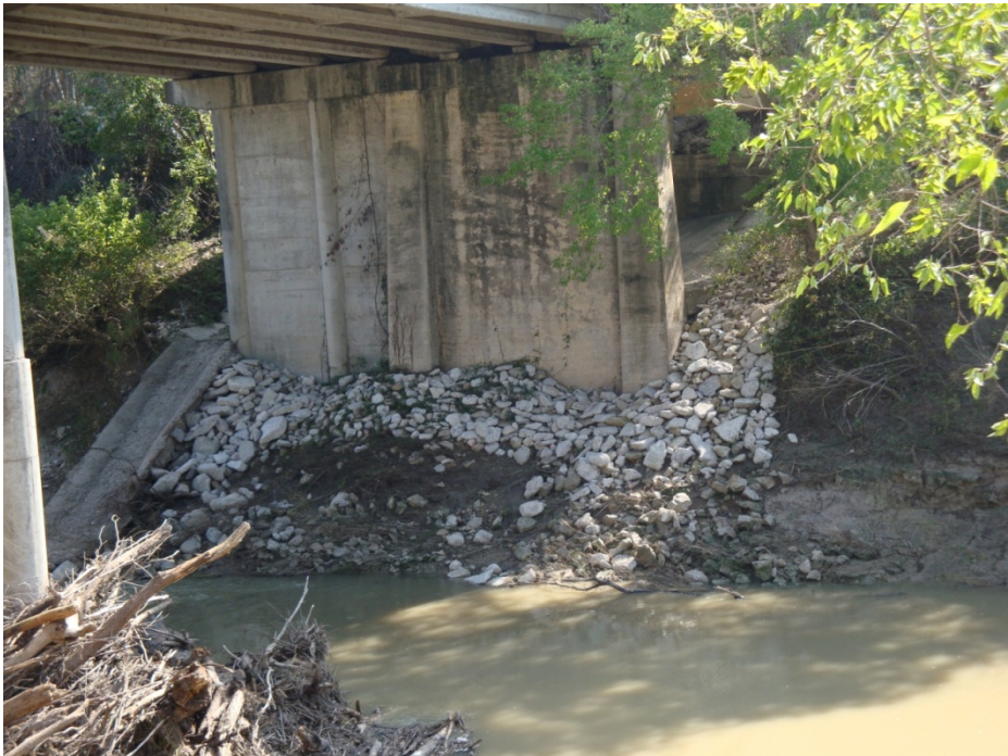
Figure E-8. Silty Clay at Pier P3.
