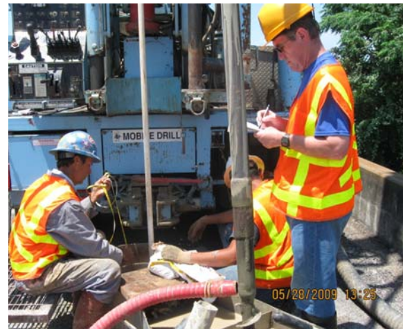
Figure 5-18. Refilling the Drilled Hole.
