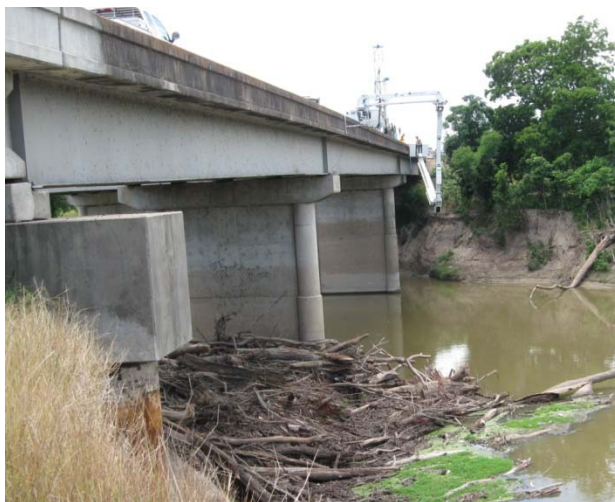
Figure D-7. Working on a Snooper Truck (SB1 is front pier with debris).
