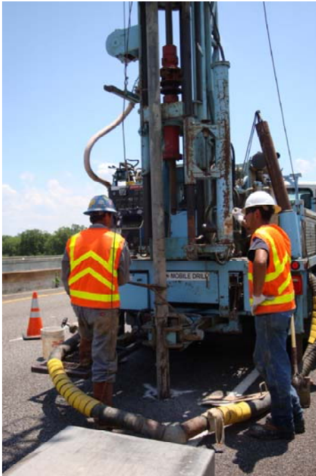
Figure 5-19. Installation of TBS.
