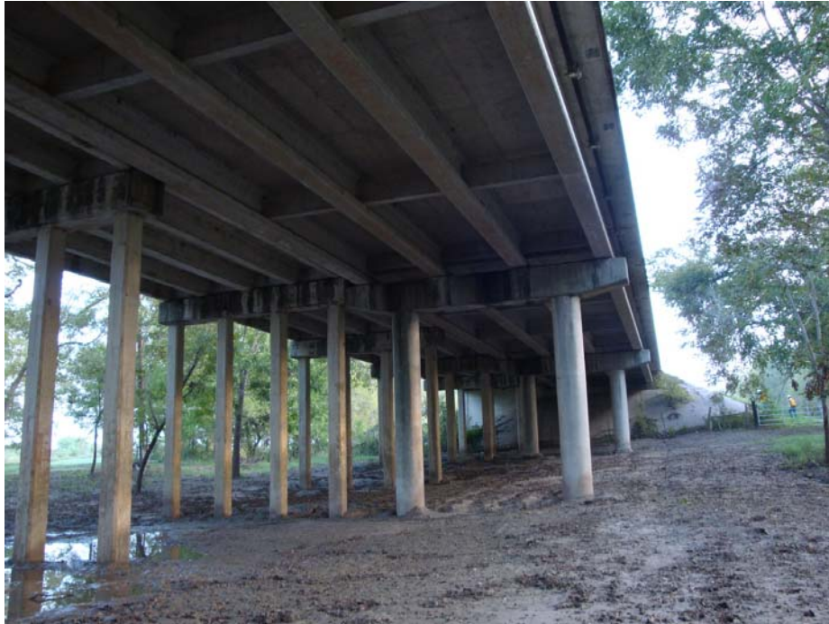
Figure 6-6. Eastern Line of the SH80 over San Antonio River Bridge.
