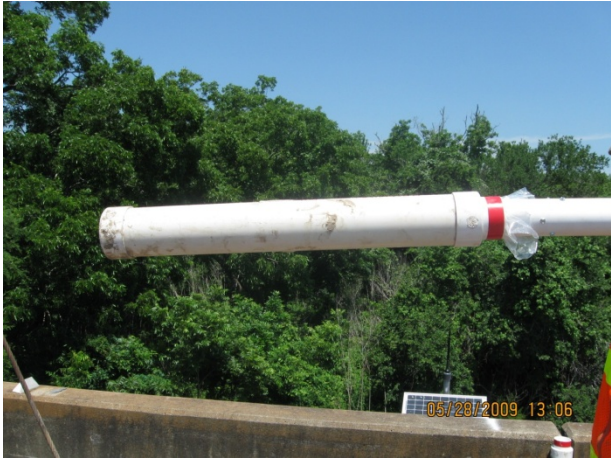
Figure D-24. Float-Out Device Mounted in the PVC Pipe.
