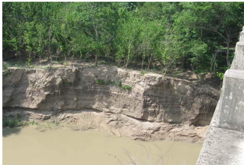
Figure E-10. Southern Bank of San Antonio River (Downstream of the Bridge).
