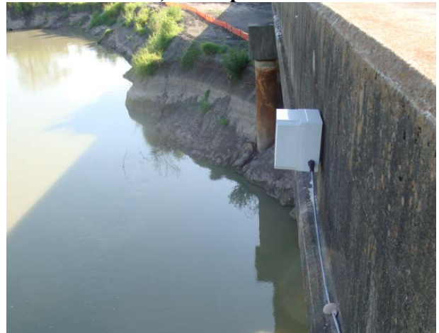
Figure 5-27. Single-Axis Tiltmeter (Tiltmeter2) on the Deck (Near Pier SB1).
