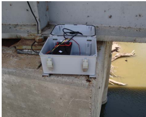
Figure 5-13. Wireless Accelerometer on Top of Pier SB1.
