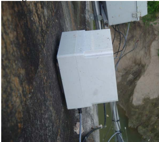
Figure 5-26. Single-Axis Tiltmeter (Tiltmeter1) on the Deck (Near Pier SB2).
