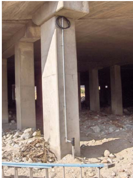
Figure C-4. Magnetic Sliding Collar Installation (Caltrans).
