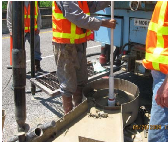
Figure 5-17. Lower the Float-Out Device.
