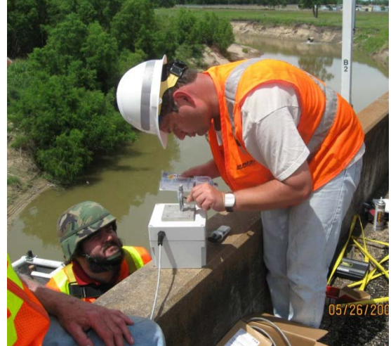
Figure D-10. Applying Glue to the Tiltmeter Enclosure.
