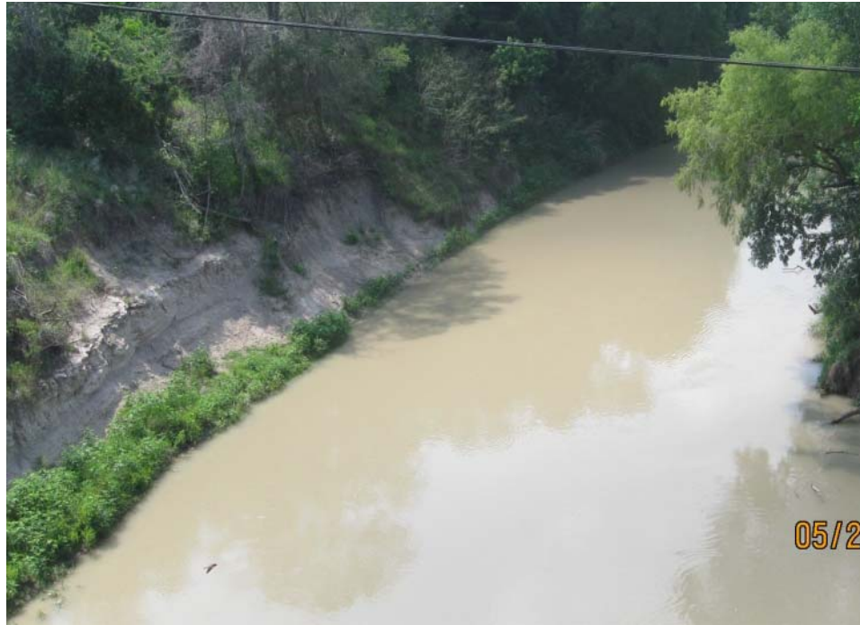
Figure 6-9. Northern Riverbank of San Antonio River (Downstream).
