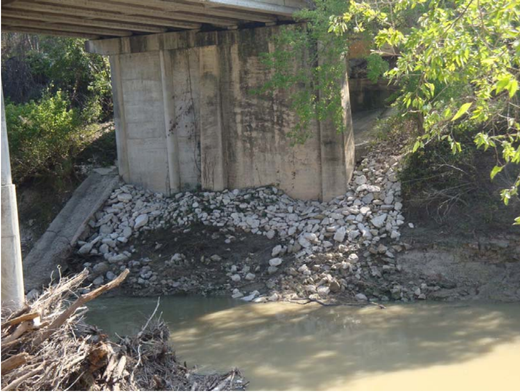
Figure 6-8. Silty Clay beneath Pier P3.
