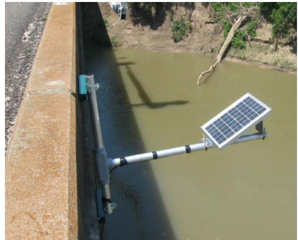
Figure D-5. Solar Panel on the Pier SB1 (with Debris).
