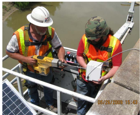
Figure D-8. Drilling a Hole in the Tiltmeter Enclosure to Install the Bolt.
