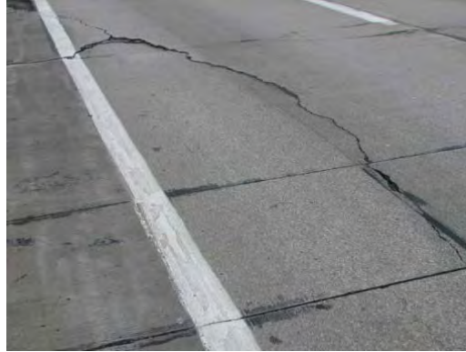
Surface cracking
