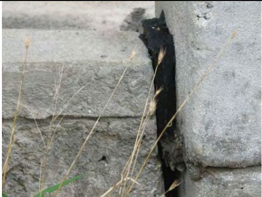
BAS movement from the abutment
