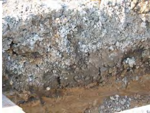
Approach slab base
