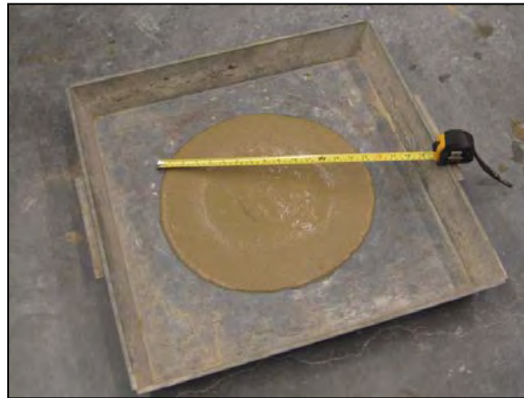
Figure 5-2: Measurement of CLSM flow
