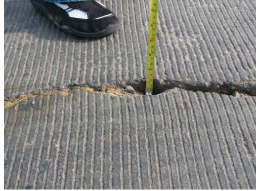
Surface cracking
