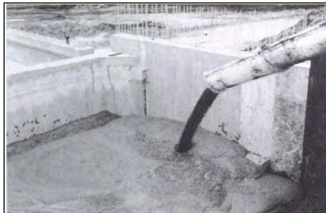
Figure 5-1: Placement of CLSM behind bridge abutment [33]
