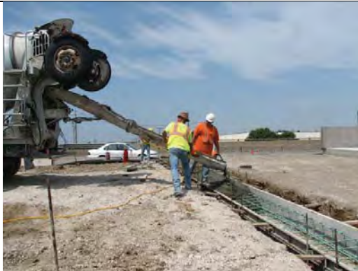
Pouring of Sleeper slab
