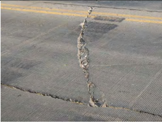
Surface cracking
