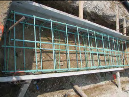
Sleeper slab reinforcement
