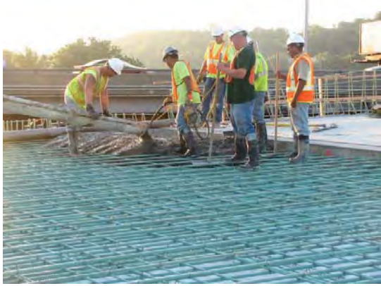
Pouring of Concrete in BAS
