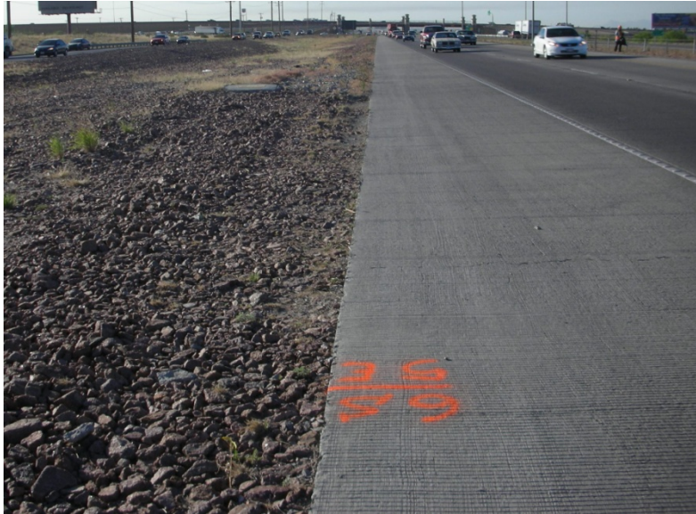
Figure 4-3. Sample Unit Limits Marked on Roadway Shoulder.
