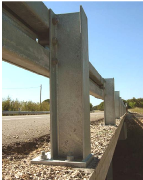
Figure 3.2 Texas Type T101 bridge rail (9)
