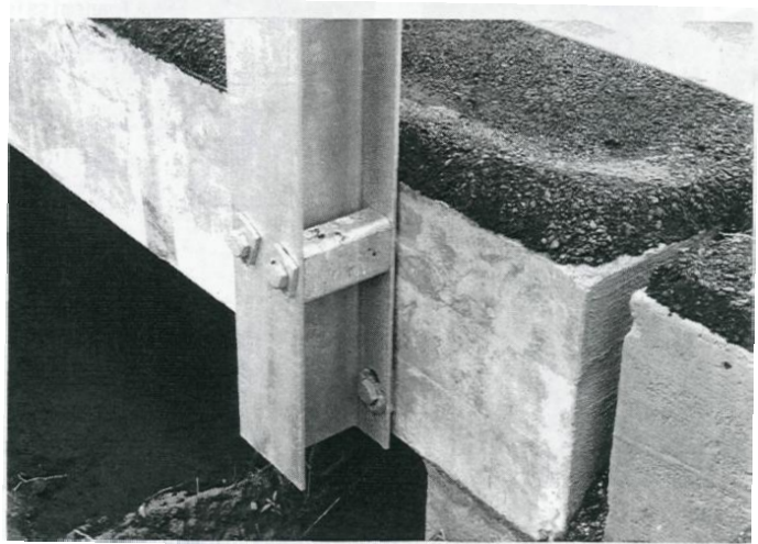
Figure 3.6 Oregon side-mounted bridge rail installation (8)
