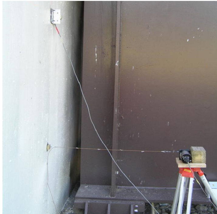
Figure 5.6. Abutment horizontal translation and rotation monitoring
