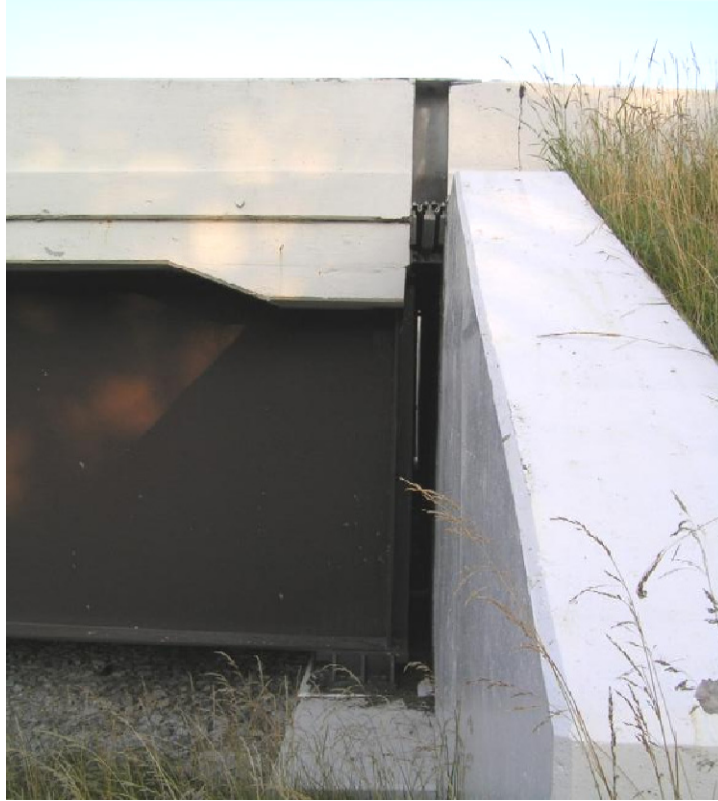
Figure 5.51. Girder bearing at abutment
