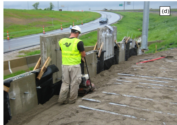
d. compaction of backfill next to the wall
