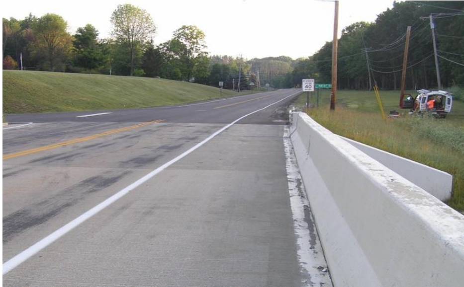
Figure 5.53. New asphalt pavement up to approach slab
