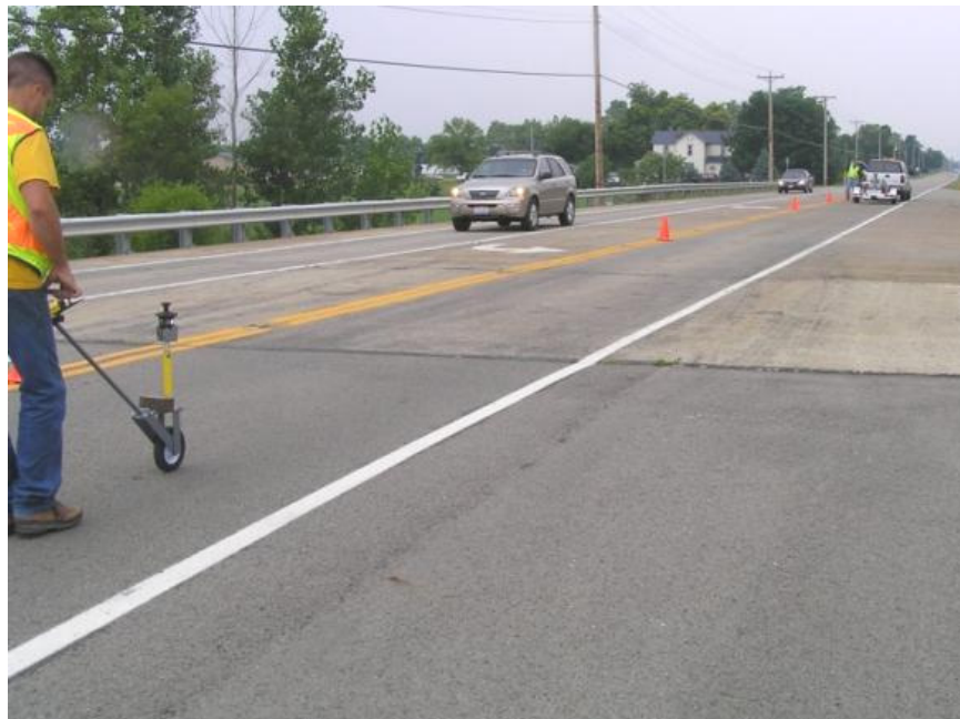
Figure 5.38. Condition of LIC 40-12.53 bridge surface
