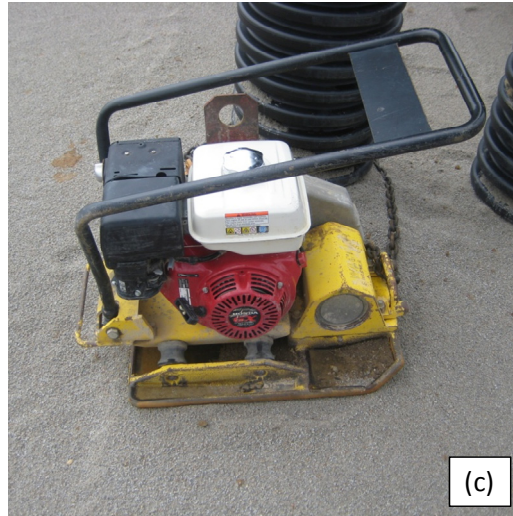
c. Vibratory plate compactor used for compaction of wall backfill
