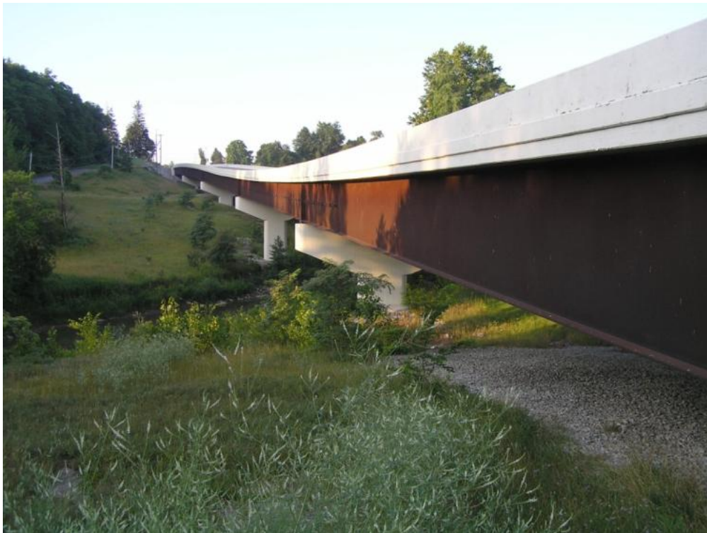
Figure 5.50. Five spans of ERI 60-2.39
