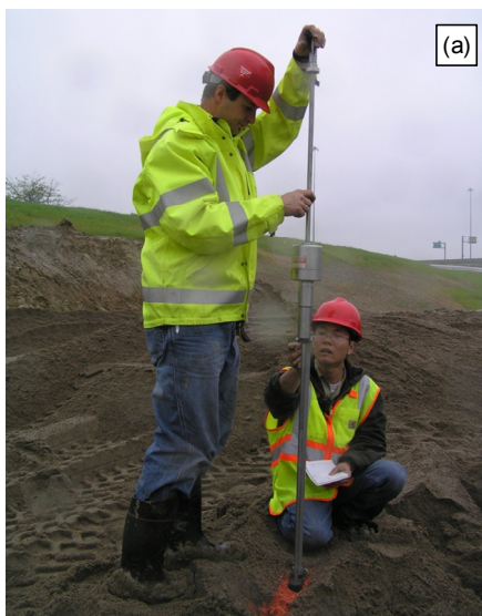
a. Dynamic cone penetrometer (DCP)
