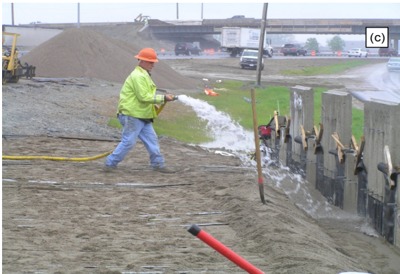
c. watering of backfill prior to compaction
