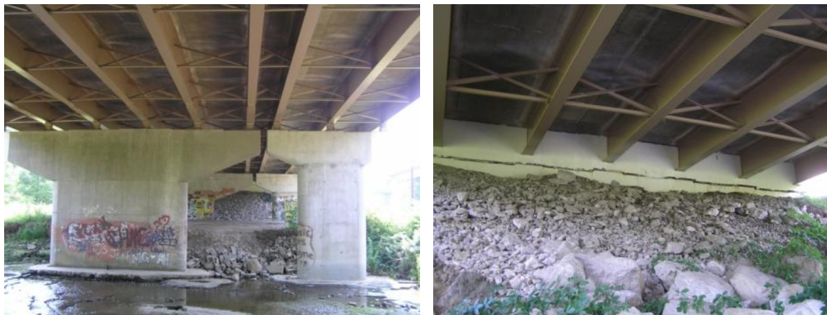
a. Widened bridge
