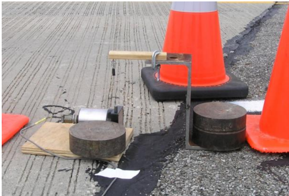
Figure 5.5. Displacement transducer at approach-pavement joint
