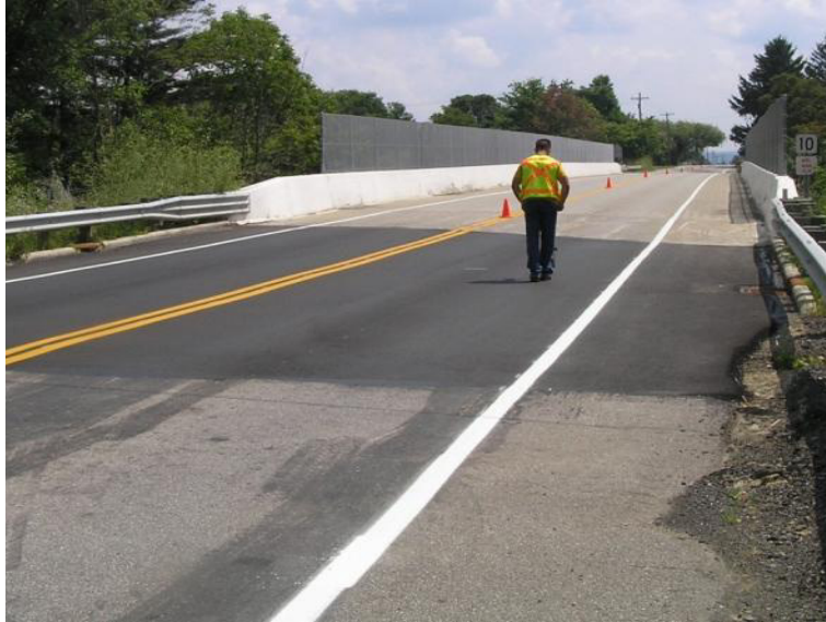
Figure 5.22. RIC 430-9.98 newly placed asphalt wedge and mud-jacked slab
