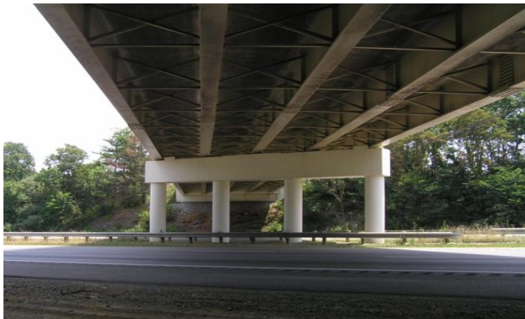
Figure 5.20. RIC 430-9.98 crossing over I-71
