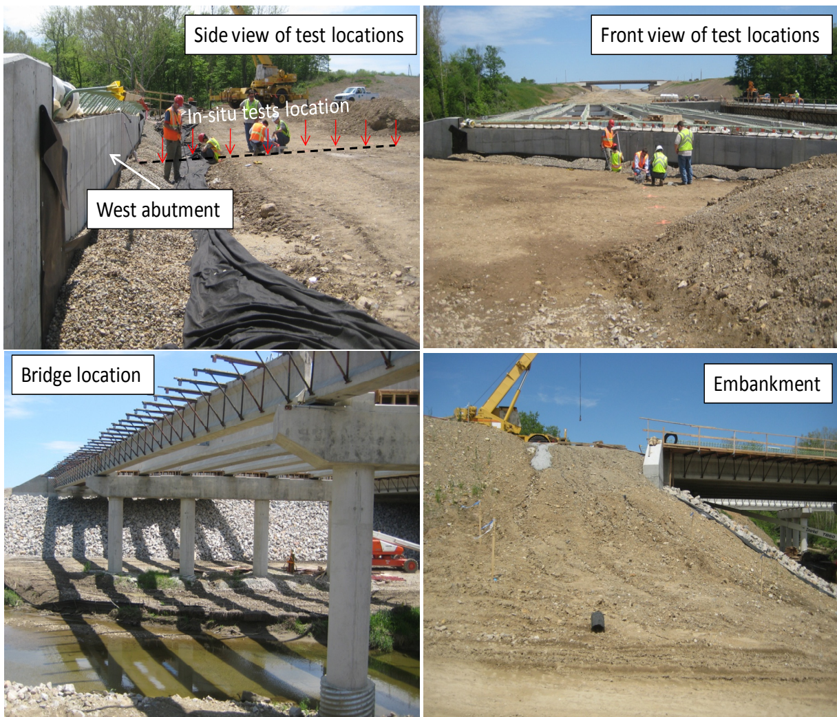
Figure 6.35. Bridge #5 (LIC-37-1225L) at Licking 161 over Moots Run
