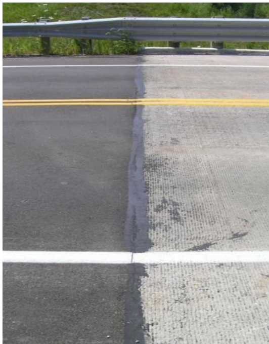
a. Pavement to approach joint
