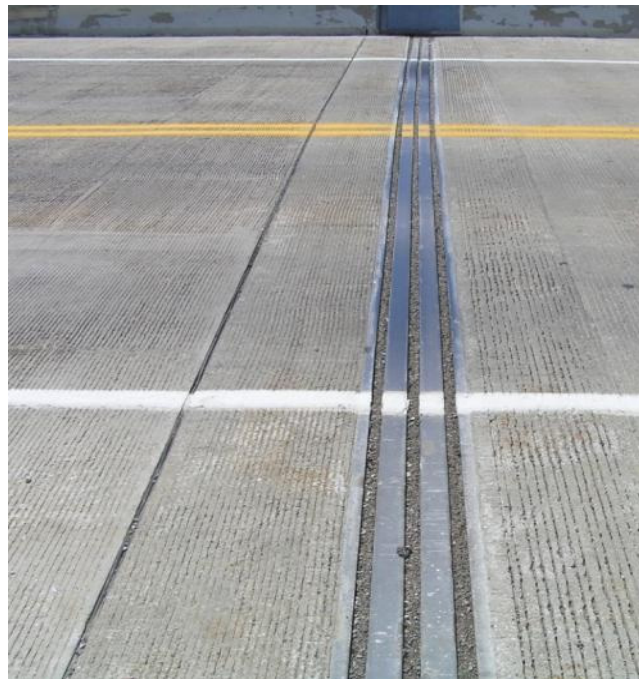
b. Approach to bridge joint
