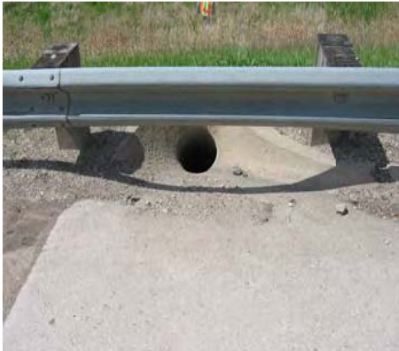
Figure 4.11. Effective surface drain detail (White et al., 2005).
