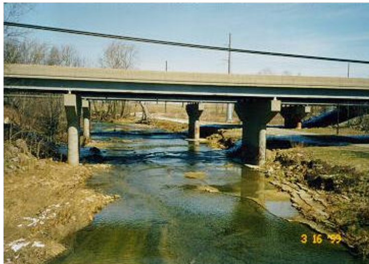
Figure 5.30. Profile of PRE 70-12.49 prior to widening
