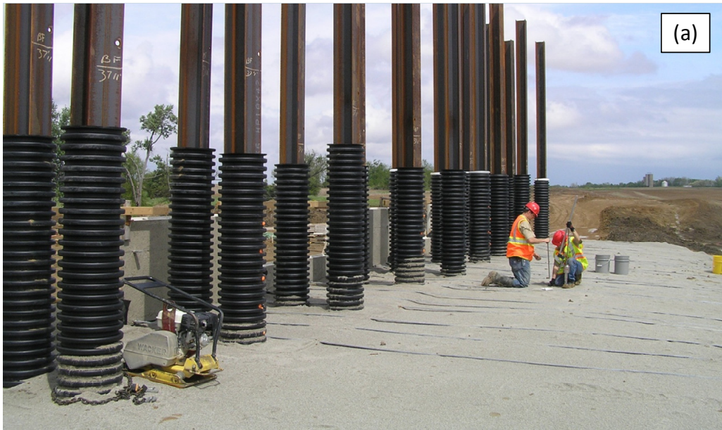
a. Overview of the south MSE wall
