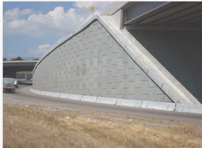
Figure 1. An MSE wall along US-89 in Davis County
