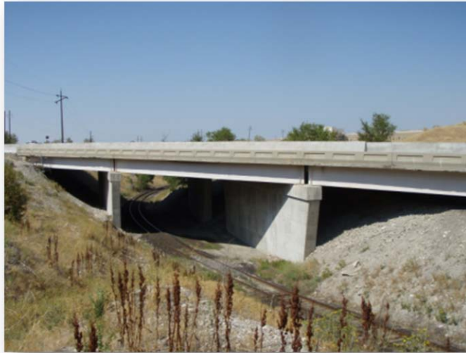
Figure 2. Bridge “C 371 2” over the Kennecott Railroad spur
