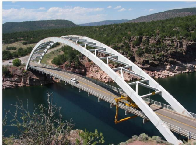
Figure 1. Cart Creek Bridge (OC 372)
