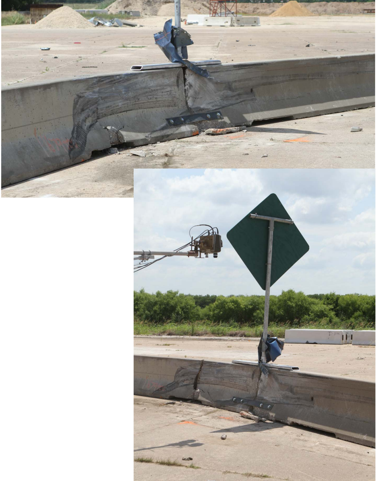
Figure 9. Installation after Test No. 461430-1.
