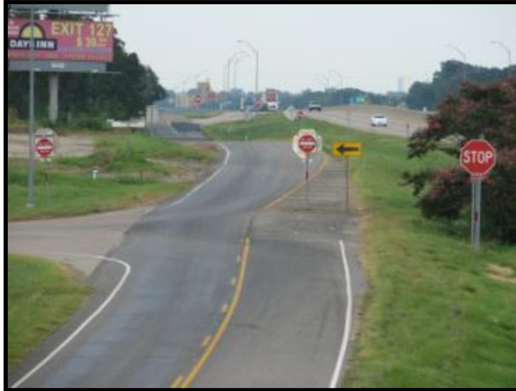
Figure 3-8. Example of a Transition Intersection Unit Type.
