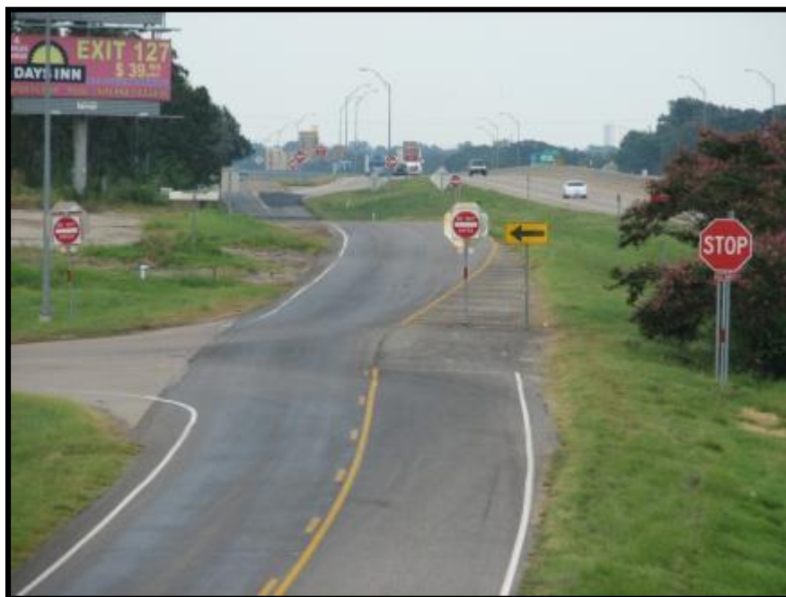
Figure A-13. Transition Intersection from One-Way to Two-Way Operation Showing “Do Not Enter” Signing (Sulphur Springs).
