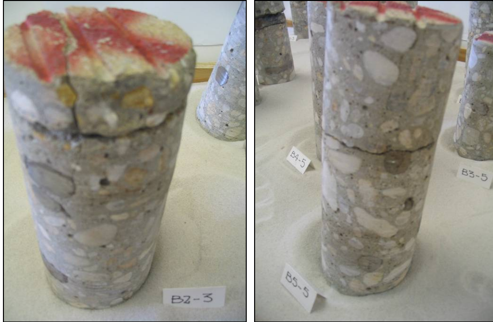
Figure 1-4: Cores from the US 331 deck with vertical and horizontal cracks
