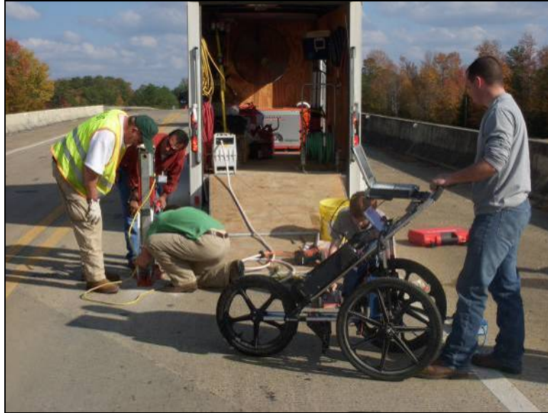
Figure 3-24: View of the bridge deck on SR 216 over L&N RR
