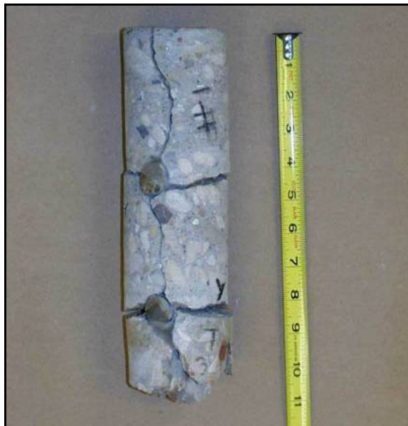
Figure 1-6: Core from CRC pavement in Texas with vertical and horizontal cracks (Courtesy of Dr. Moon Won)
