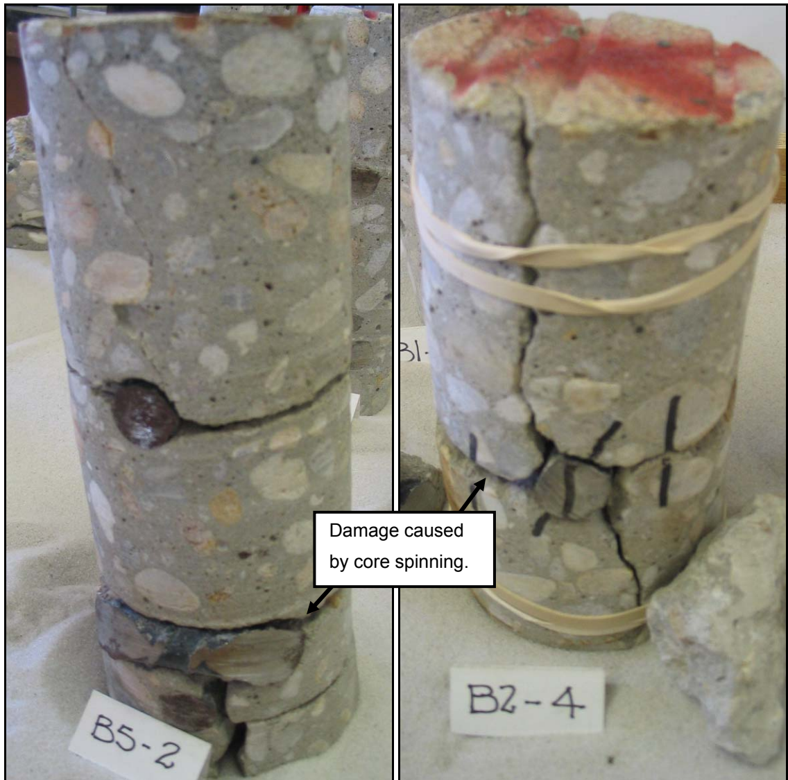
Figure 3-8: Cores from the US 331 deck with vertical and horizontal cracks
