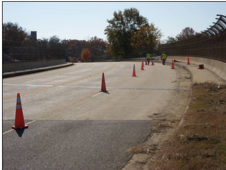
Figure 3-19: View of the bridge deck on SR 49 over SCL RR in Lineville
