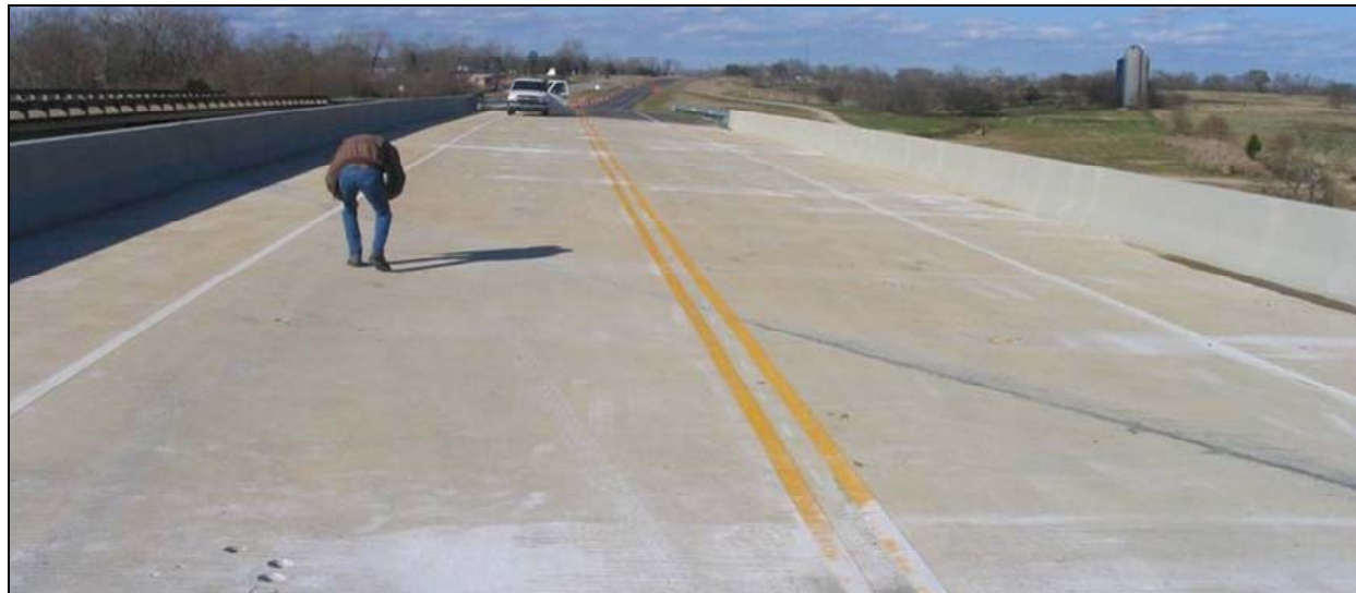
Figure 1-3: View of the northbound lanes of the US 331 bridge deck
