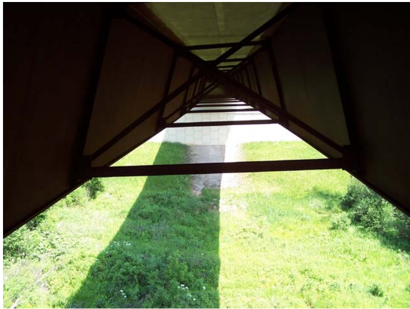
Figure 3.3: View Between Bridge Girders
