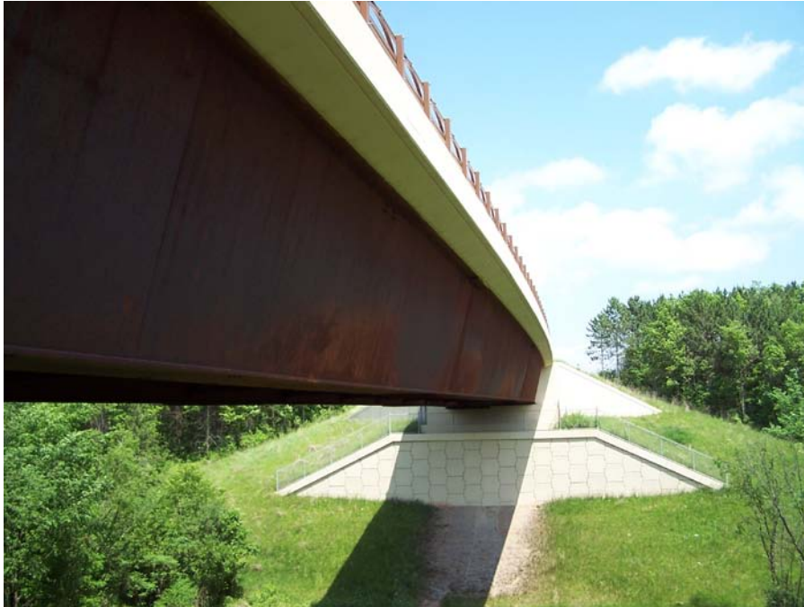
Figure 3.10: East Face of Bridge
