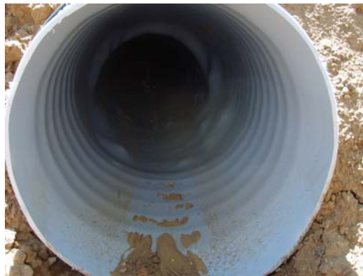
Figure 16. Inlet of fold-and-form rehabilitated culvert
