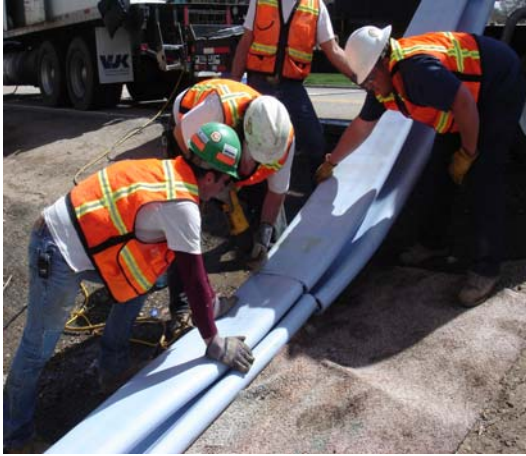
Figure 15A. Cutting liner
