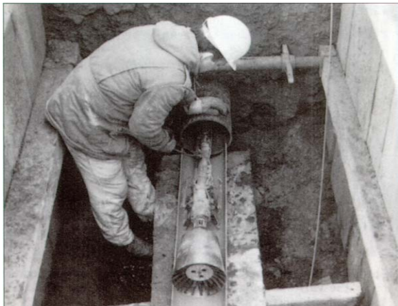
Figure 19A. Lining machine for non-man entry culverts (www.dot.ca)
