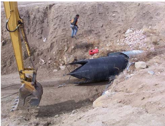
Figure 5A. Cutting out nose cone
