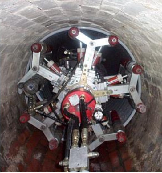
Figure 11A. Full-bore expanding machine ( www.dot.ca.gov )
