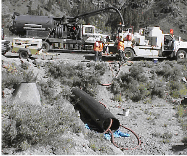
Figure 18. Steam being introduced into a 30 inch HDPE liner (www.htliners.com)
