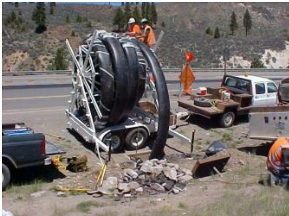
Figure 17A. Liner on a spool
