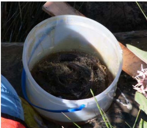
Figure 6A. Oakum being soaked in urethane sealant
