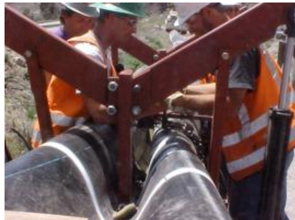
Figure 17B. On-site deforming equipment
