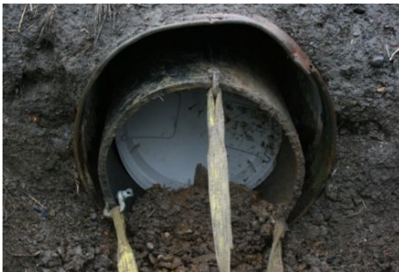
Figure 4. Optional cleaning device for culverts
