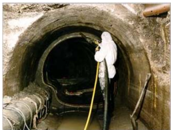
Figure 19B. Large diameter cement-mortar lining (www.cflhd.gov)
