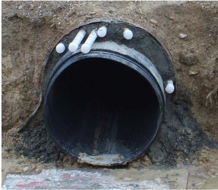
Figure 3. Inlet of segmental-lined culvert
