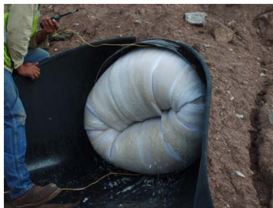
Figure 13. Outlet end of inverted liner
