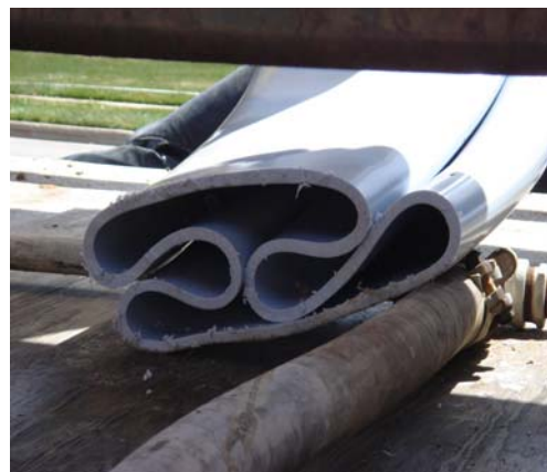
Figure 14B. H-shape liner (15- to 30-inch)
