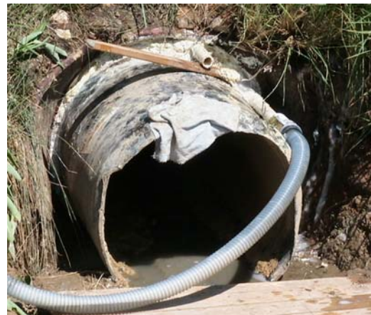
Figure 6B. Inlet sealed with Oakum
