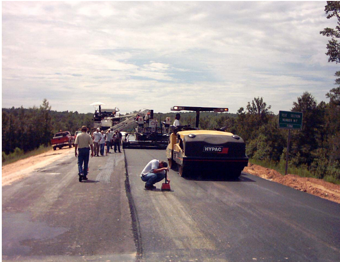
Figure 2.2 Construction of Test Sections.
