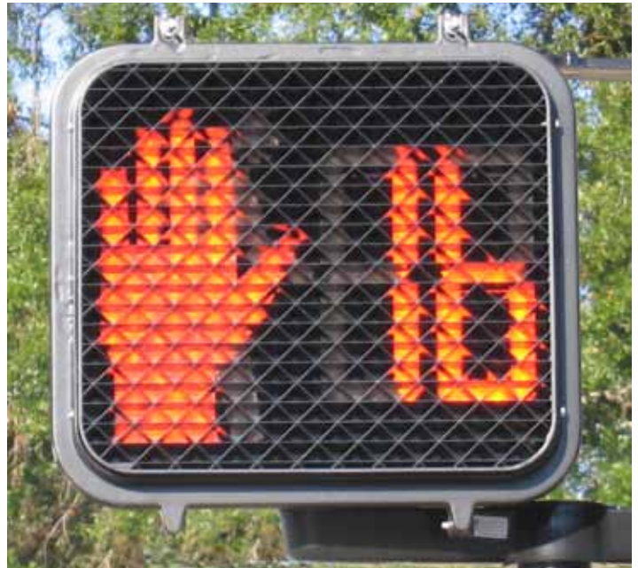
A countdown pedestrian crosswalk signal at the TERL facility.
