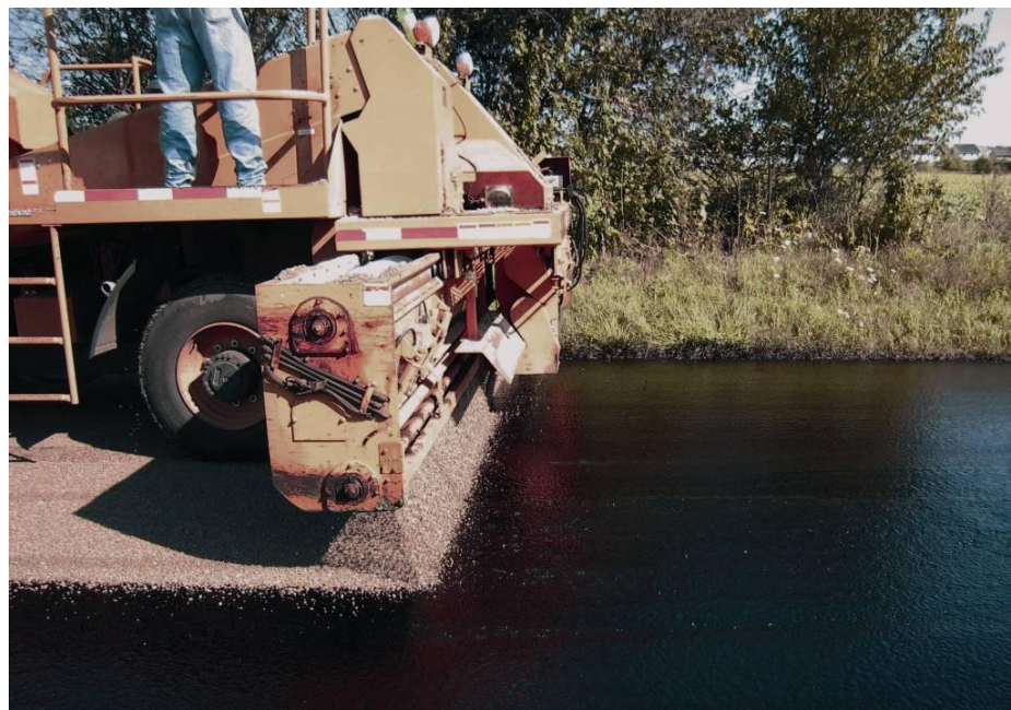
A chip spreader applies cover aggregate during a seal coat or “chip seal” operation on 74 th Street in Cedar Rapids, Iowa, during a road maintenance effort Photo: Dr. Charles Jahren, Iowa State University/CCEE
