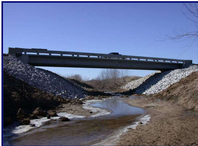
A UHPC prestressed bridge constructed on Little Soap Road in Wapello County, Iowa
