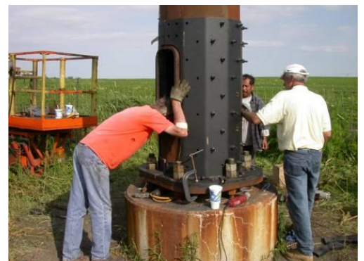
A bolted reinforcing jacket was placed on a tower in the I-35 & US 18 Interchange near Clear Lake
