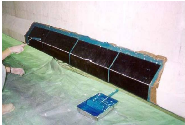
A transverse CFRP jacket being installed on a beam Photo: Iowa State University/InTrans
