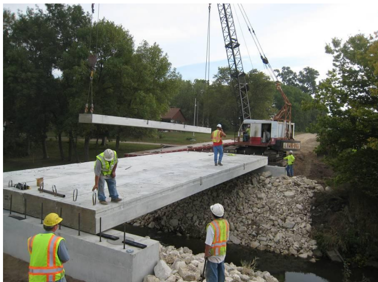
Beam placement during accelerated construction of Buena Vista IBRD bridge Photo: Dr. F. Wayne Klaiber, Iowa State University/CCEE
