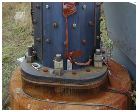
Bolted Reinforcing Jacket
