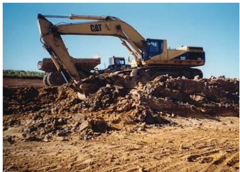
Soil mixing operation through layered soils, Des Moines, Iowa Photo: Vern Schaefer, Iowa State University/CCEE
