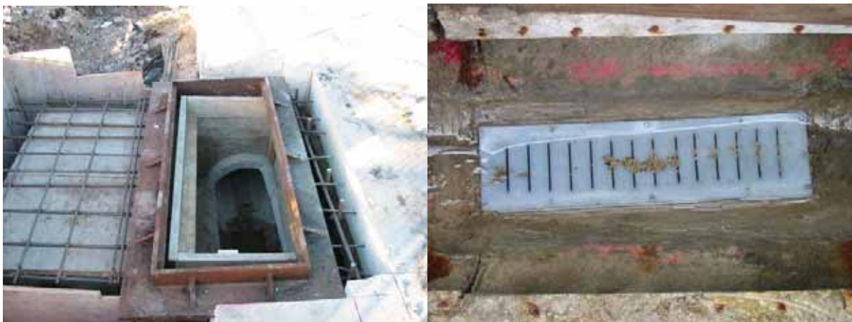
Figure 6. Manhole constructed for water-quality sampling of the highway runoff; bedload sample.
