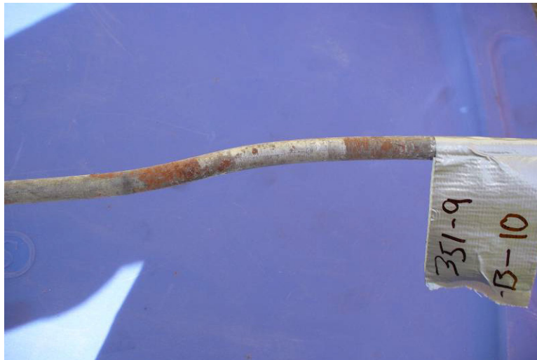
Figure 17 Damage and subsequent corrosion of coupon R-351-9-B-10 near panel face of two-stage MSE wall
