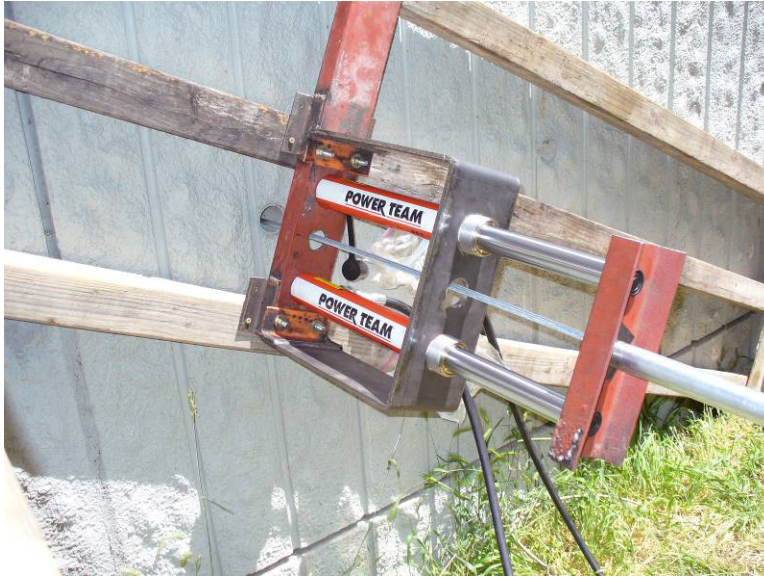
Figure 6 Alternate setup of equipment for coupon extraction
