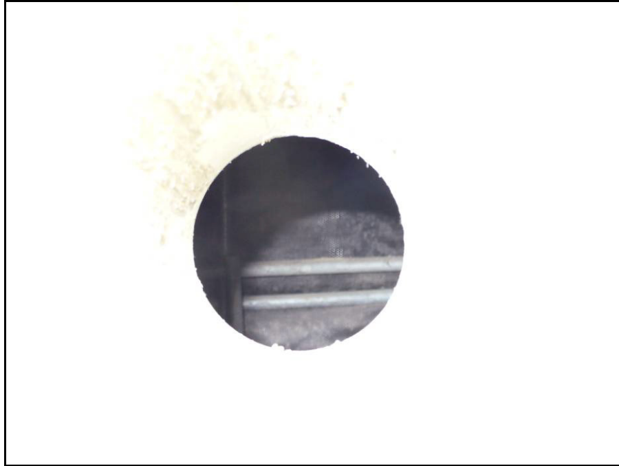
Figure 8 Typical view of welded wire mesh through coupon access hole in two-stage MSE wall
