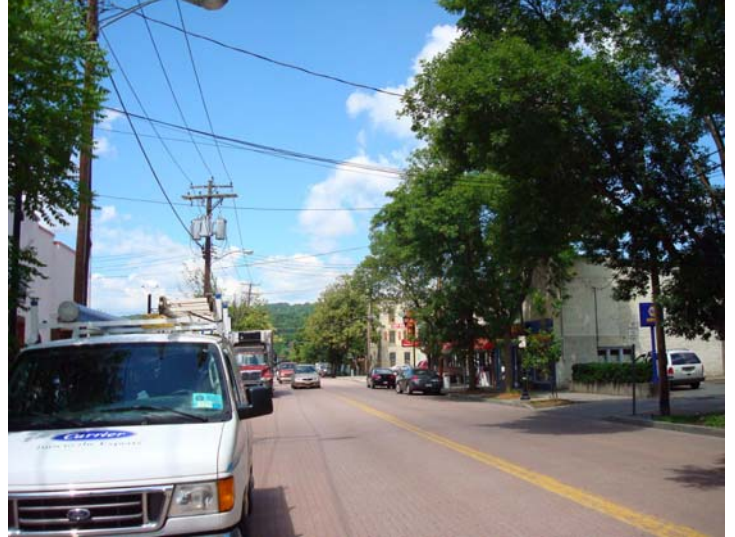
Figure 4-4. Example of utility infrastructure in Ithaca, NY
