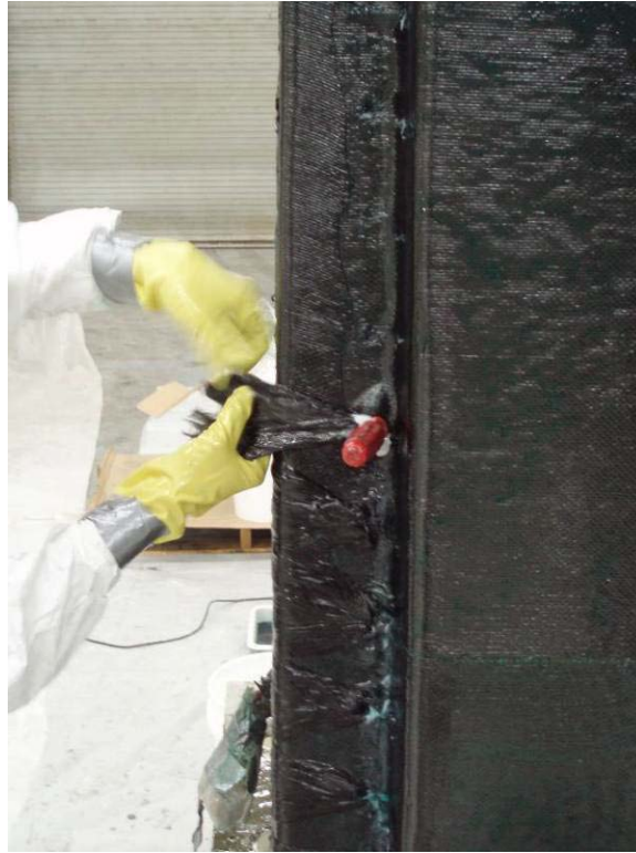
Figure 12 – FRP Anchor Installation
