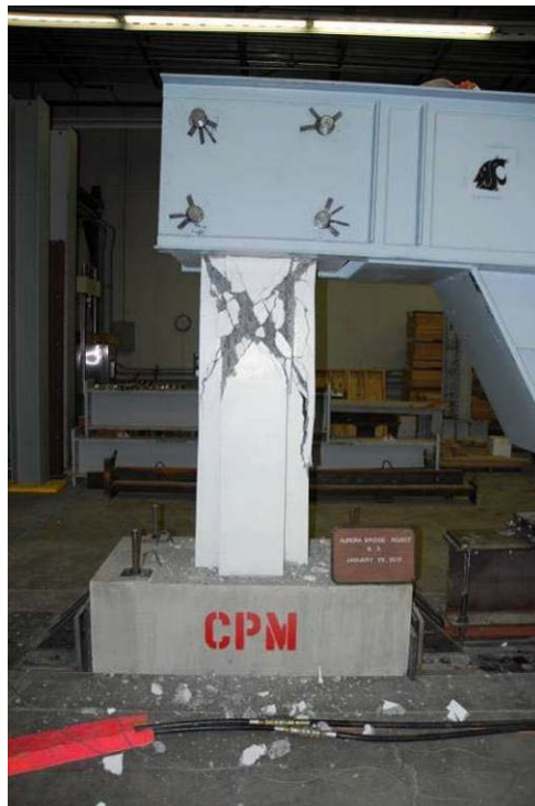
Figure 23 – Column 5 Shear Cracking Near the End of Testing
