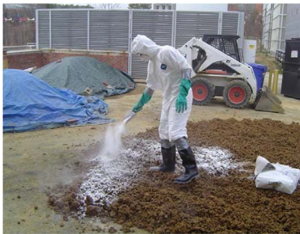
Figure 55. Spreading of Hydrated Lime on Coastal Plain Subgrade
