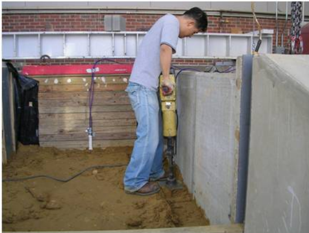
Figure 56. Initial Soil Compaction using Vibratory Plate Compactor
