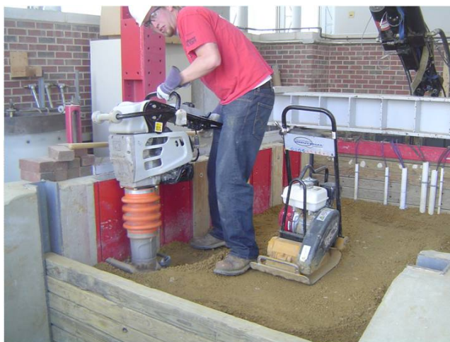
Figure 58. Additional compaction on LSS using Jumping-Jack Rammer
