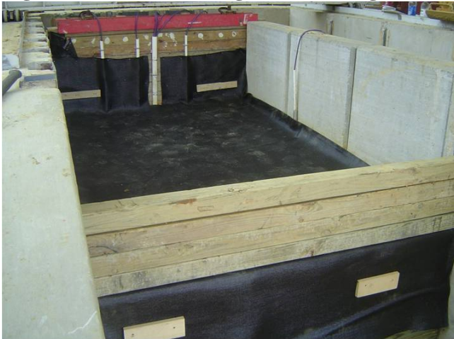
Figure 60. Installed Geotextile A before granular layer placement
