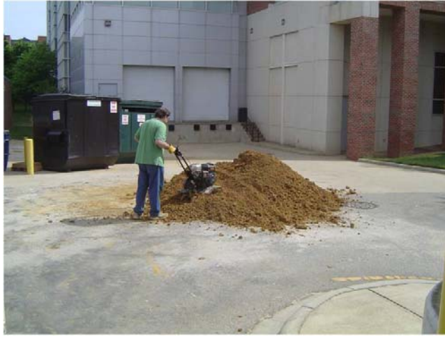
Figure 54. Soil Preparation with Front-Tine Tiller
