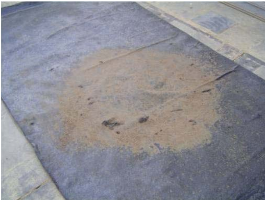
Figure 94. Fabric Stained by Subgrade Fines - Post 13" ABC with Geotextile B (14) Test
