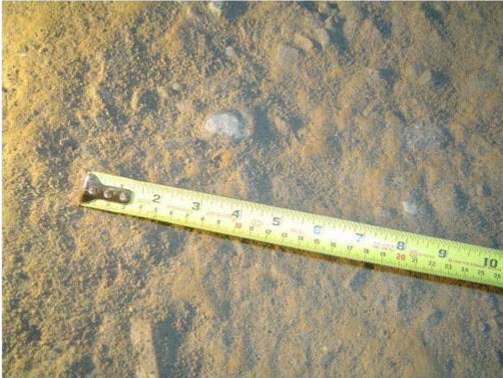
Figure 88. Intrusion of ABC into Coastal Plain Subgrade Surface - Post 14" ABC (5) Test
