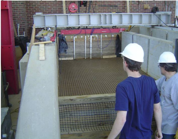
Figure 59. Installed Geogrid B before granular layer placement
