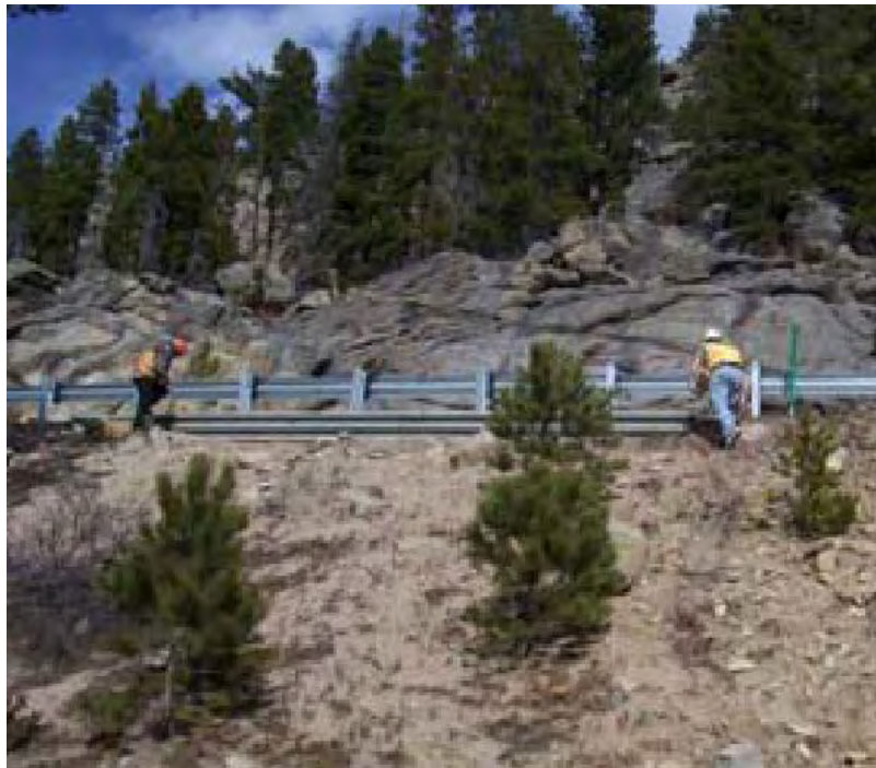
Figure 6. Guardrail stabilization system along SH-72.
