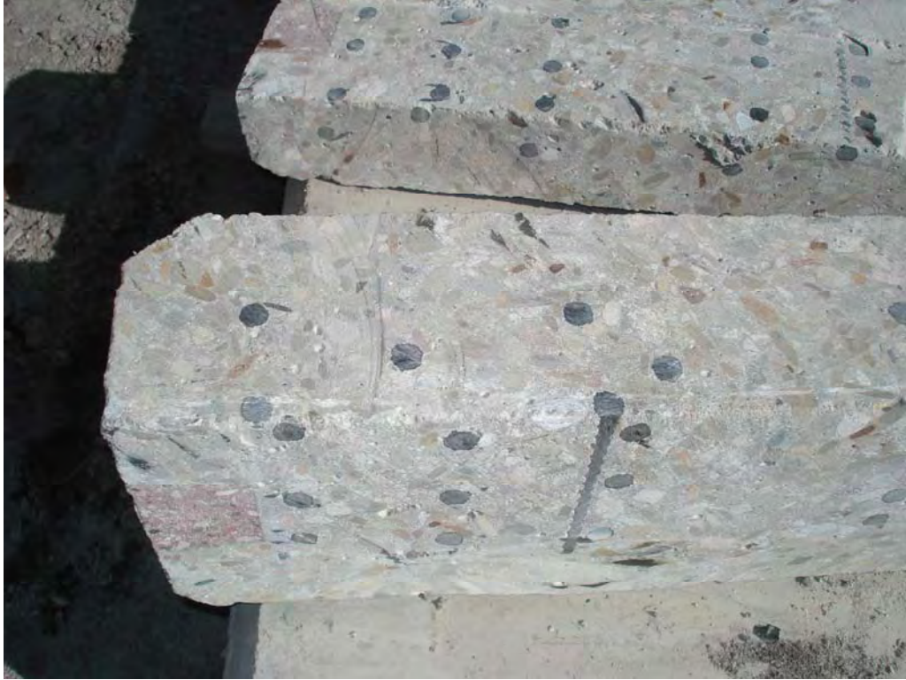
Figure 8: Normal Concrete Bonding
