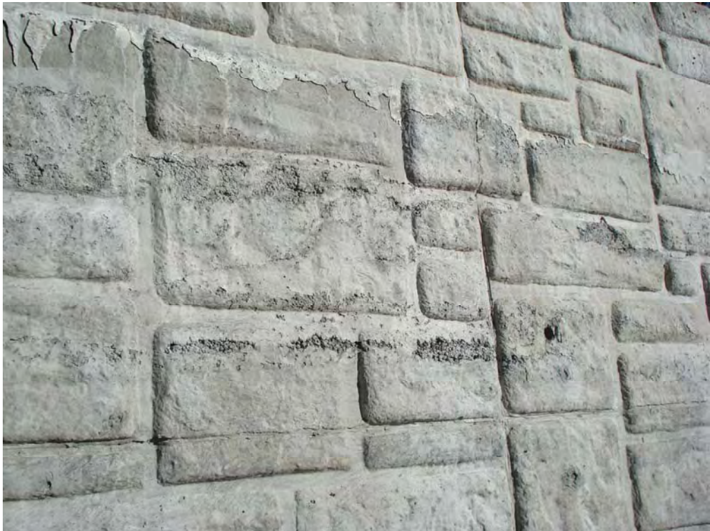
Figure 18: Southern Abutment Finish 2
