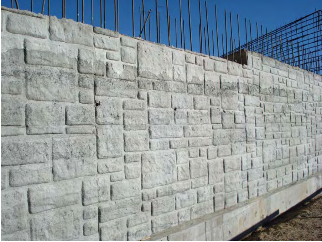
Figure 16: Exposed Face Southern Abutment
