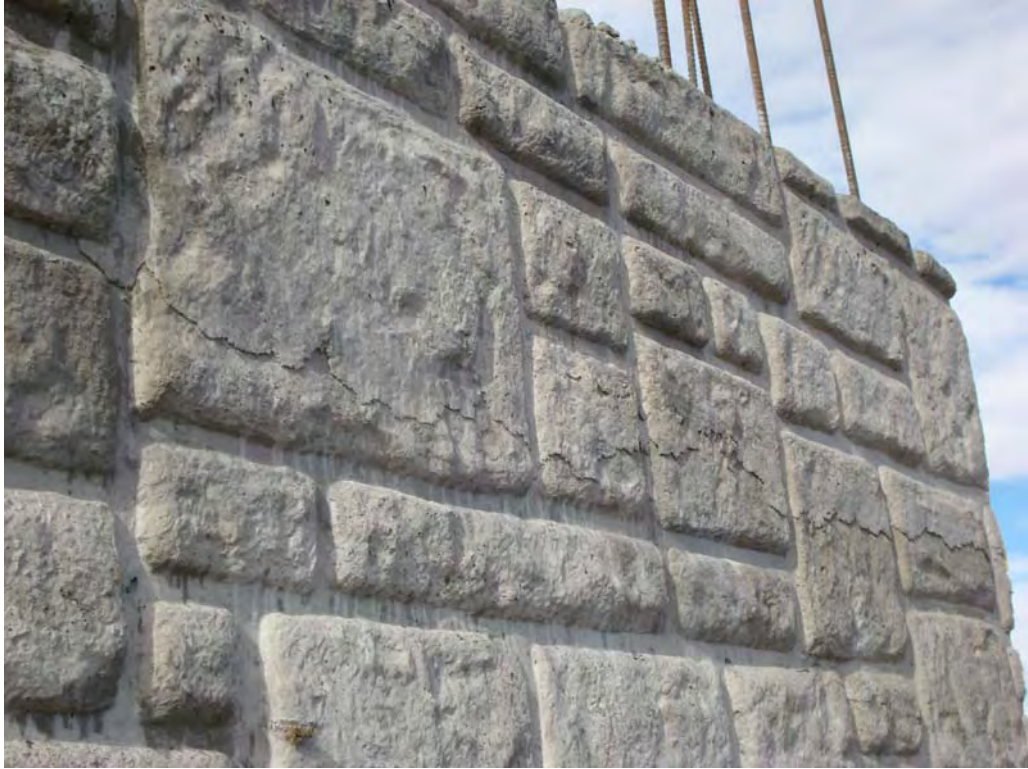
Figure 20: Northern Abutment Exposed Face
