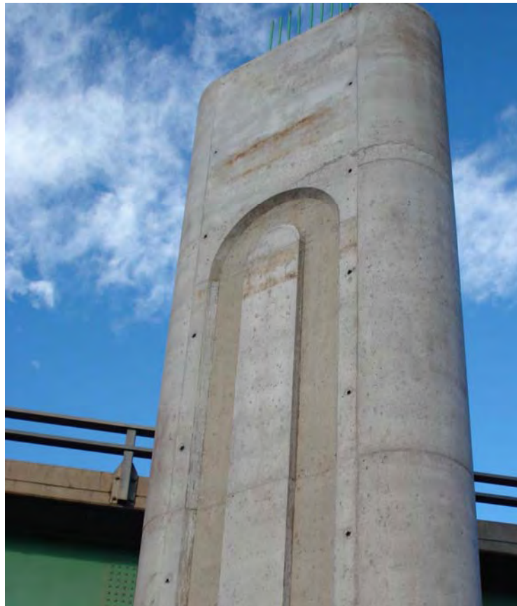
Figure 23: Visible Placement Separations
