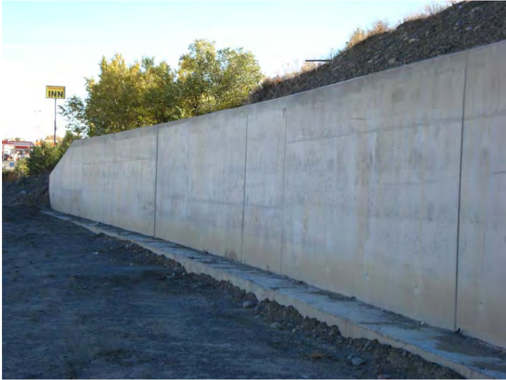
Figure 12: Second Retaining Wall Placement
