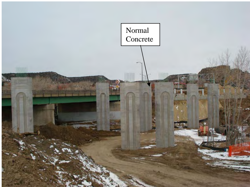
Figure 21: Northbound Bridge Piers
