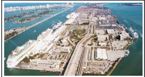
Port of Miami Tunnel, Florida (DBFO with availability payments). Expected to open in 2014, the tunnel will connect the Port of Miami with the MacArthur Causeway and I-395. Senior bank debt, a TIFIA loan and private equity have been used to finance the project. (Photo: FHWA)
