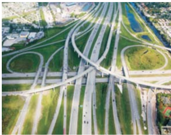
I-595 Managed Lanes, Florida (DBFO with availability payments). This project is expected to reconstruct and widen 10.5 miles of the I-595 corridor and add three reversible, dynamically tolled lanes by 2014. It is the first highway PPP in the United States to use availability payments. (Photo: Corradino Group)
