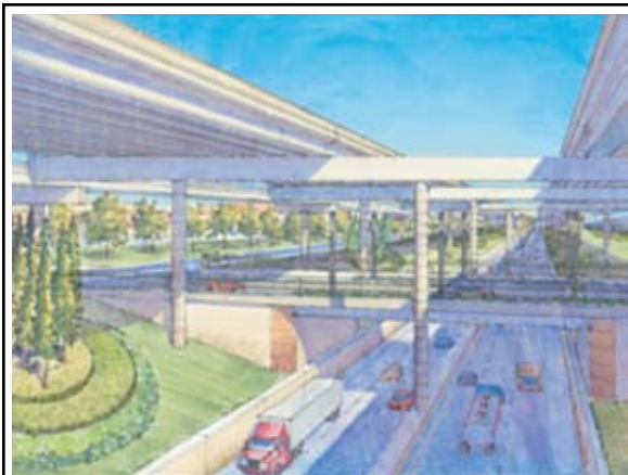
I-635 (LBJ Freeway) Managed Lanes Project, Texas (DBFOM). Expected to open in 2016, this project will add six managed lanes along I-635 (subsurface) and I-35E (elevated), besides reconstructing the main lanes and frontage roads. The private partner is under contract to operate and maintain the facility for 52 years. (Photo: Texas DOT)
