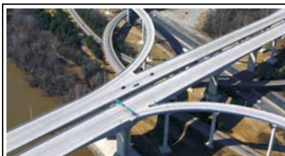
Pocahontas Parkway, Virginia (99-year lease with revenue sharing). This $354 million transportation project was the first to be implemented under Virginia's Public-Private Transportation Act of 1995. (Photo: FHWA)
