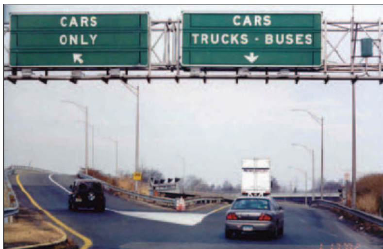
Figure 2-3. New Jersey Turnpike truck/bus lane (Collier and Goodin 2004)
