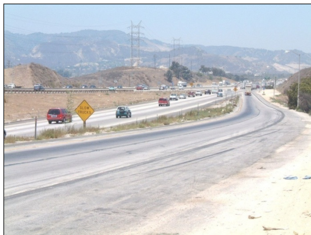
Figure 2-35. Truck bypass lanes on I-5 at I-405 north of LA (Middleton, et al. 2003)
