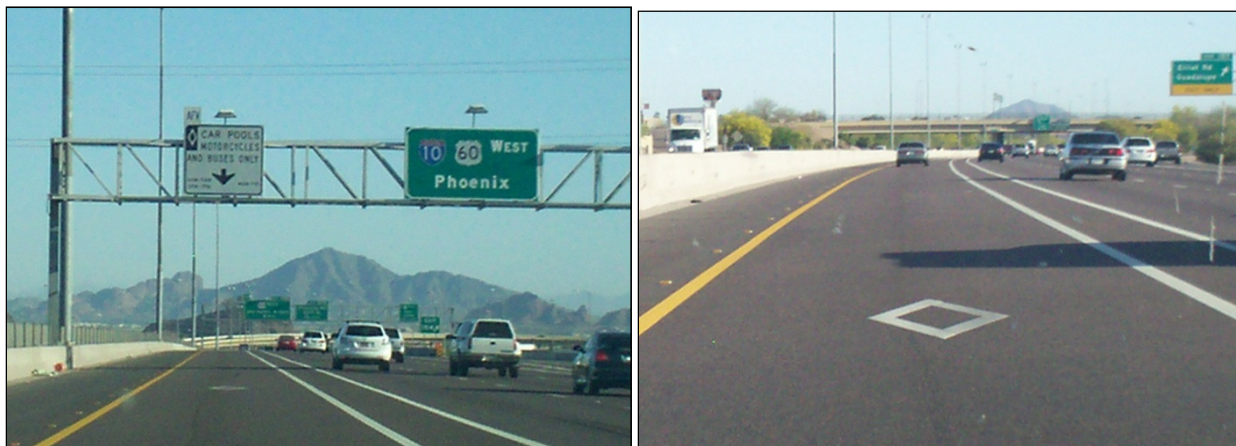
Figure 2-14. HOV signage and pavement markings, Phoenix, AZ
