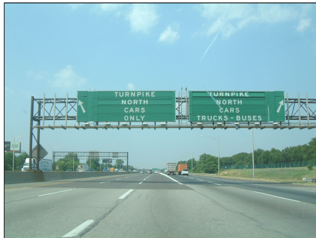
Figure 2-28. Overhead truck sign on New Jersey Turnpike (Middleton, et al. 2003)
