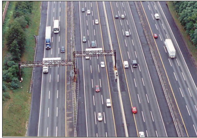
Figure 2-33. New Jersey Turnpike dual facility (Middleton, et al. 2003)
