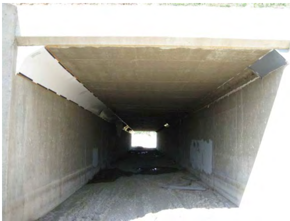
Figure 20. Looking west down CBC 4 from the CBC entrance on August 18, 2009.
