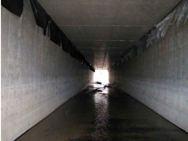
Figure 19. Status of plastic strip deterrents after December 2008 wind storm.
