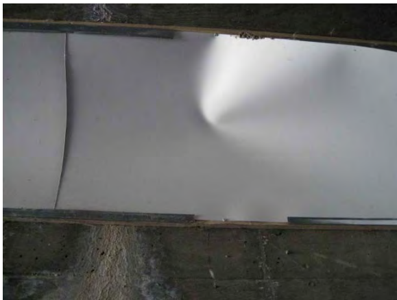
Figure 22. The two screws that kept the white plastic panel in CBC 4 from falling out completely.
