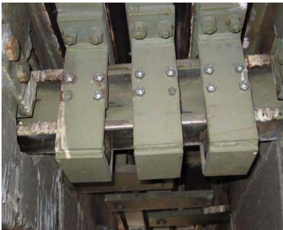
Figure 1. Pier 4 joint support beam at girder A (E16ND).
