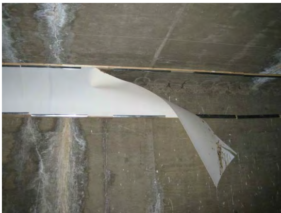
Figure 22. The two screws that kept the white plastic panel in CBC 4 from falling out completely.
