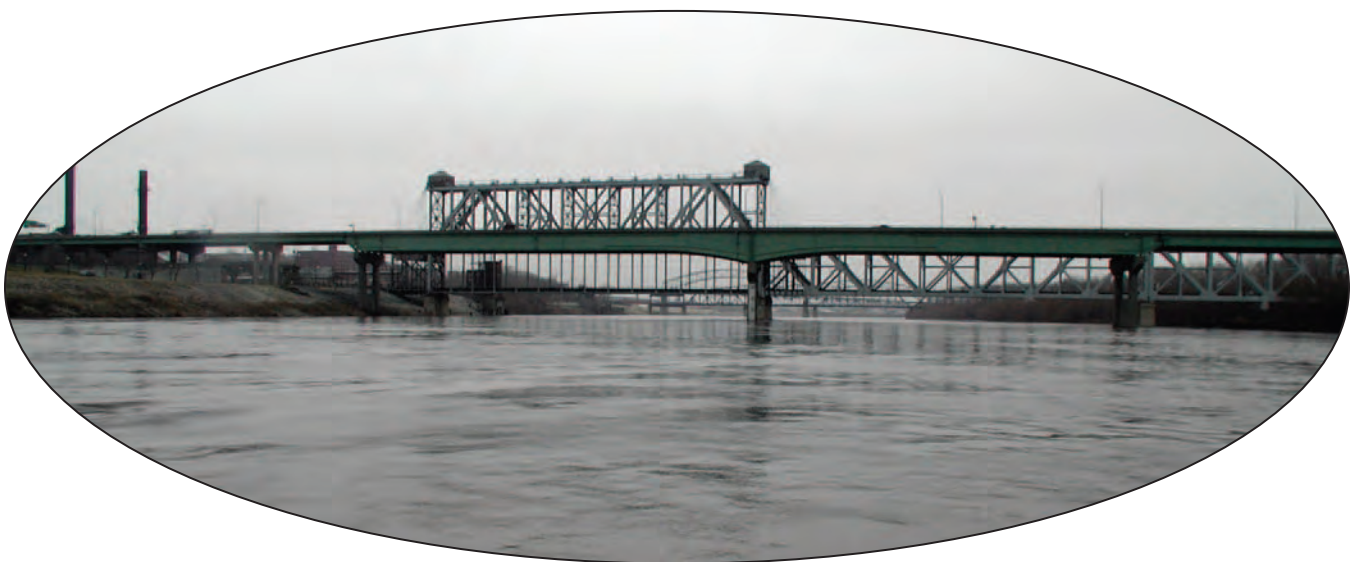
Structure A4060 on State Highway 9.
