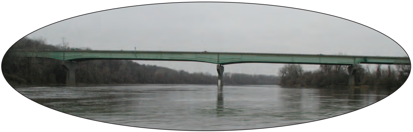
Structure A1800 on Interstate 635.
