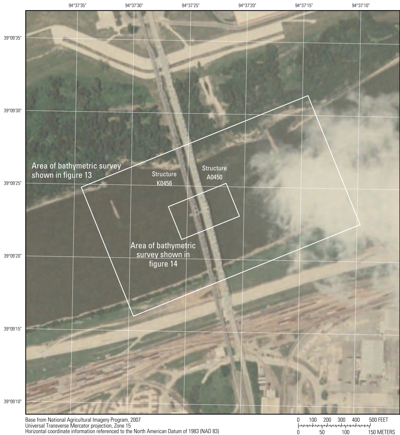
Figure 12. Location of the bathymetric survey area on the Missouri River near structures K0456 and A0450 on U.S. Highway 69 in Kansas City, Missouri.
