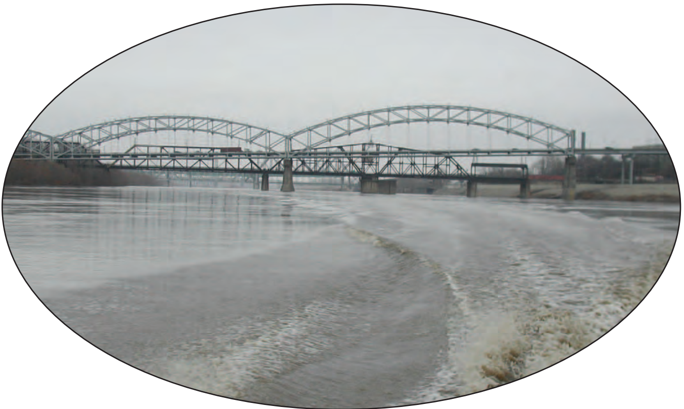
Structure A4649 on U.S. Highway 169.
