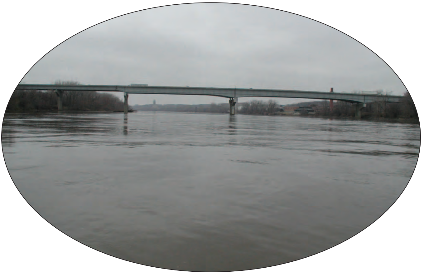
Structure A0767 on Interstate 435.
