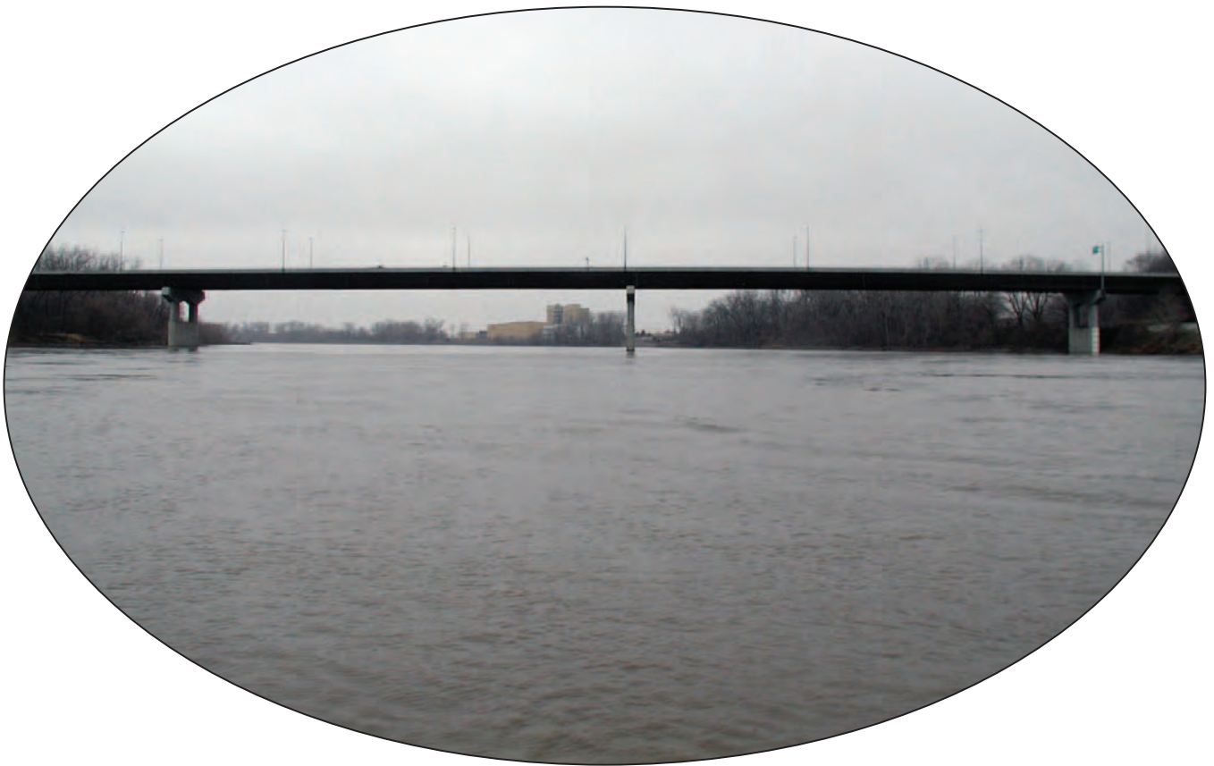
Structure A5817 on State Highway 269.
