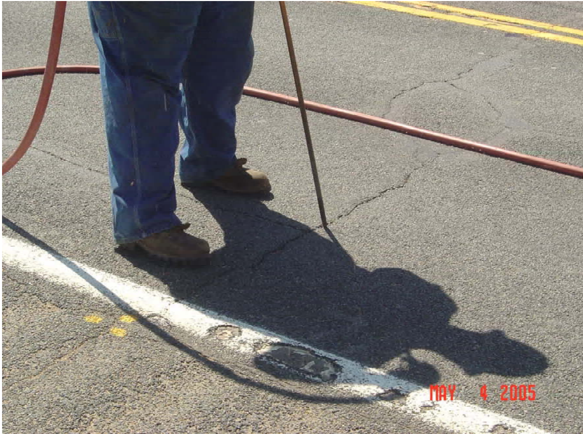
Figure A4 – Cleaning Crack with Compressed Air
