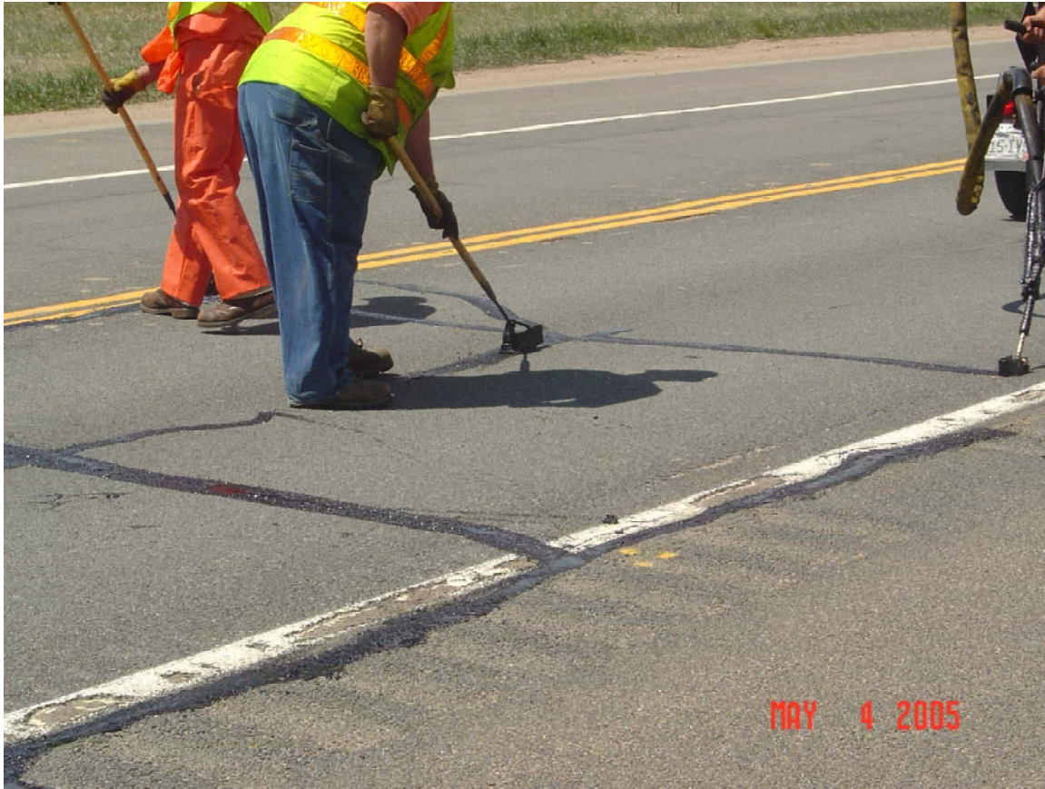
Figure A7 – Squeegee Application After Crack Pouring
