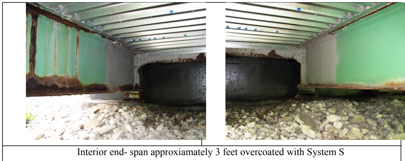
Figure 4.3 Example of a System S End-span Recoating at the Bearing Area with Early Failure.
