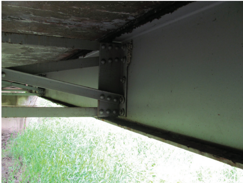
Poor Condition – Interior Beam Mid-Span
