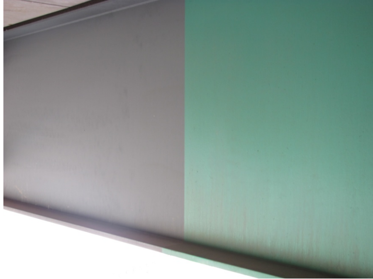
Figure 4.6 Example of 14-year-old System G Coating.
