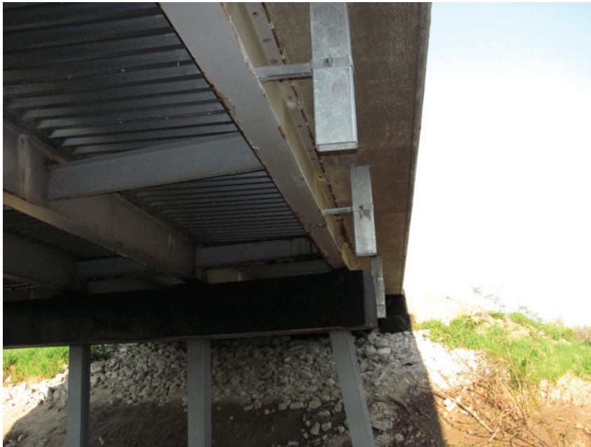
Poor Condition – Interior Beam Mid-Span
