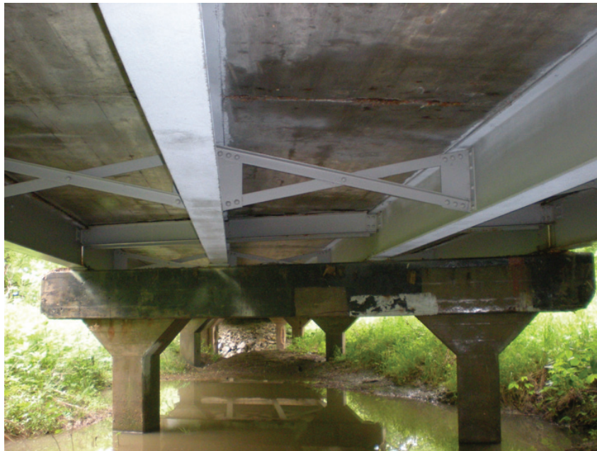
Good Condition – Interior Beam Mid-Span
