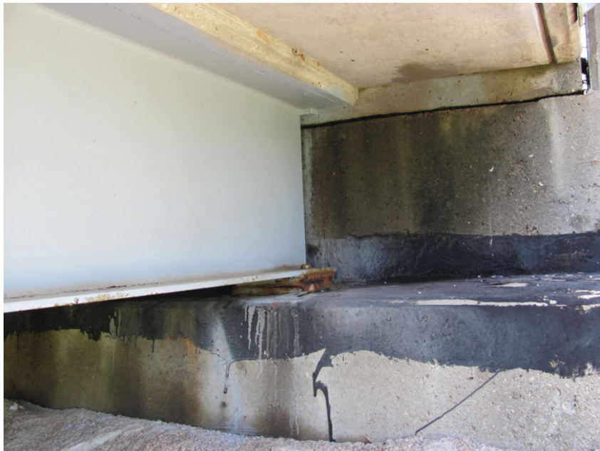
Good Condition – Exterior Beam End-Span
