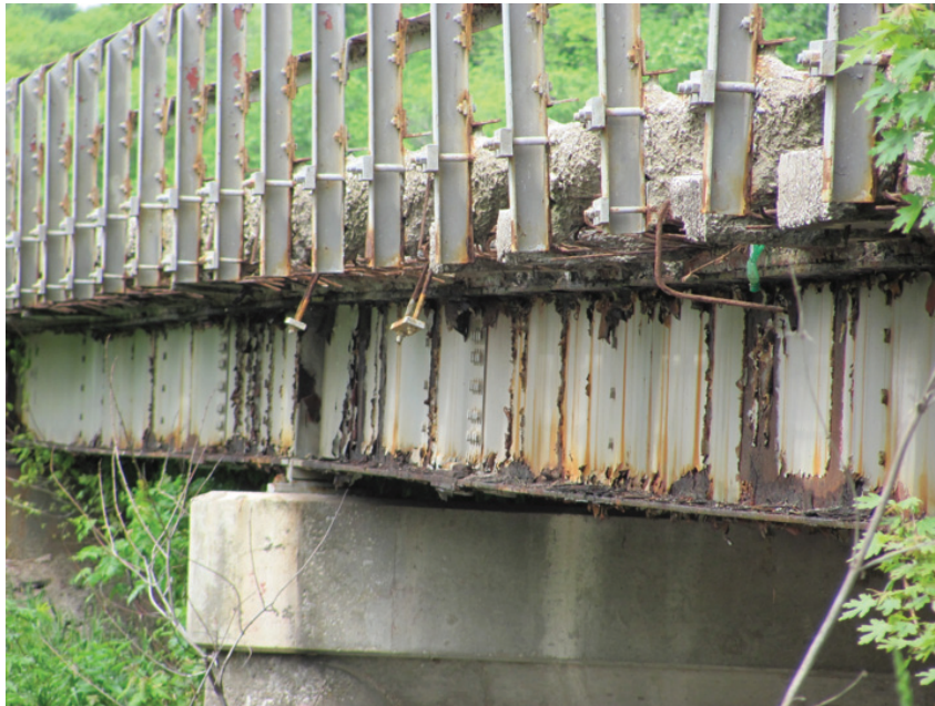
Very Poor Condition – Facia Girder Mid-Span
