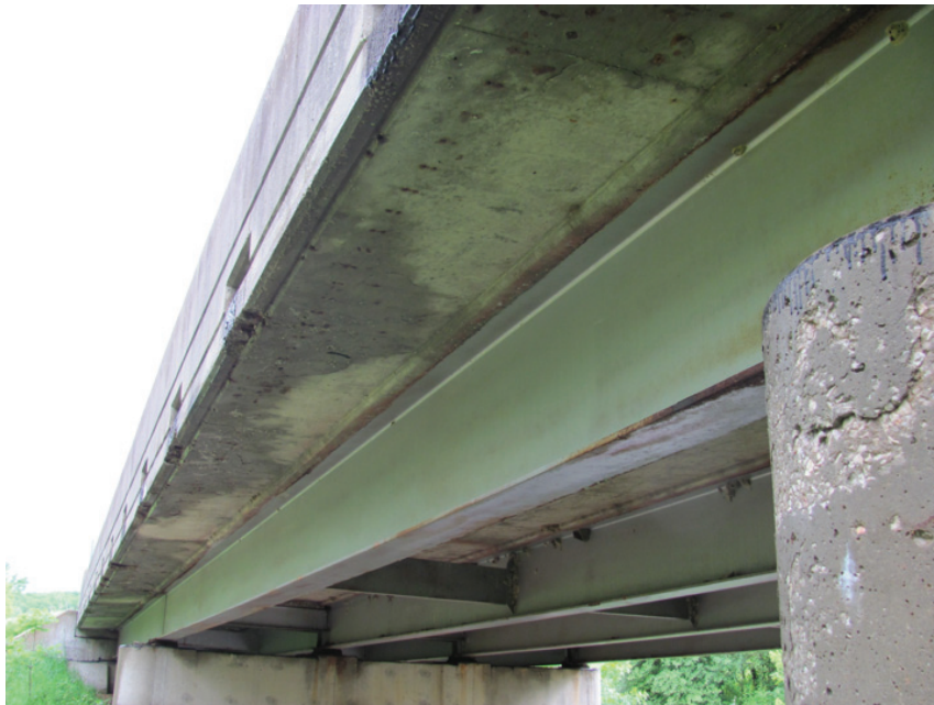
Poor Condition – Facia Girder Mid-Span
