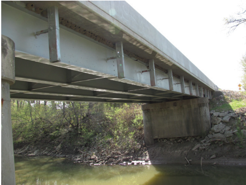
Good Condition – Facia Girder Mid-Span
