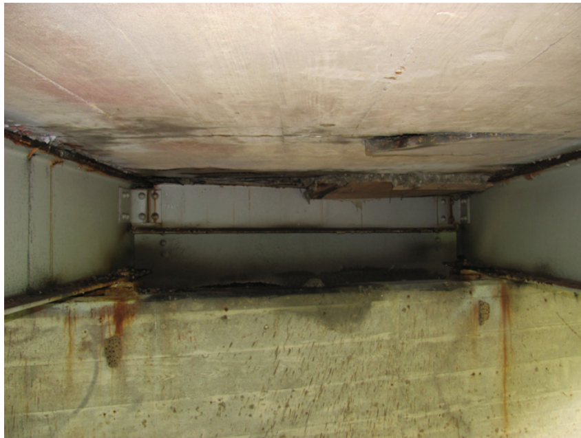
Poor Condition – Interior Beam End-Span
