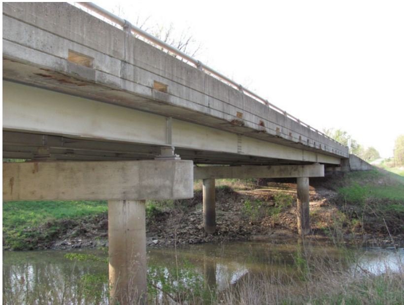
Good Condition – Facia Girder Mid-Span
