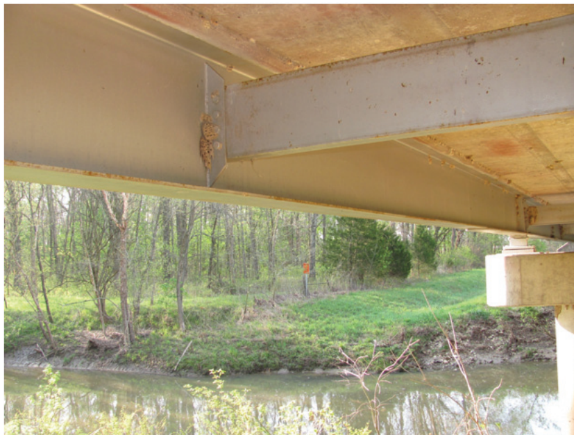
Fair Condition – Interior Beam Mid-Span
