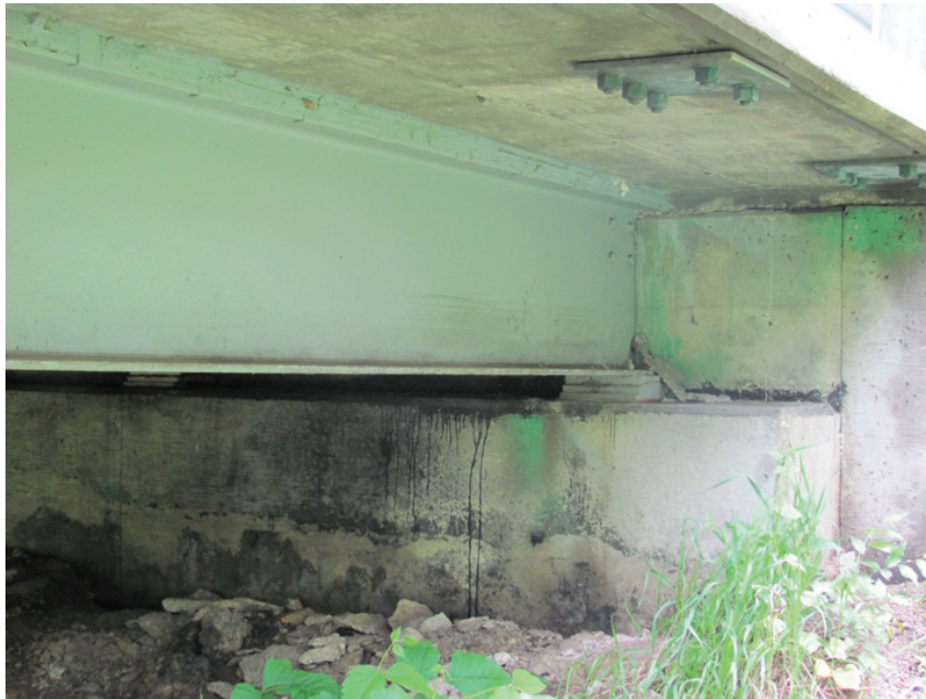
Good Condition – Exterior Beam End-Span
