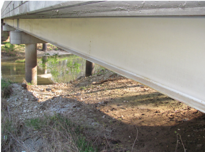
Fair Condition – Fascia Girder Mid-Span
