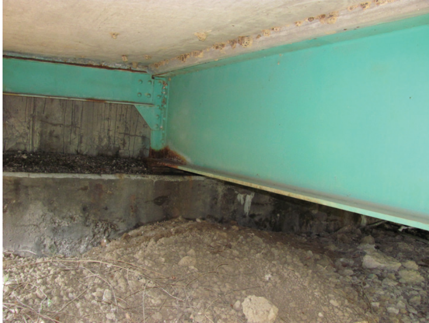
Poor Condition – Interior Beam End-Span
