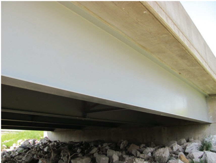
Very Good Condition – Exterior Beam End-Span
