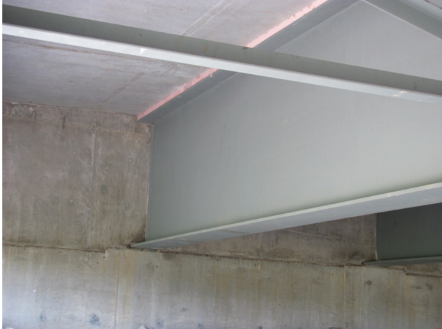
Very Good Condition – Interior Beam End-Span
