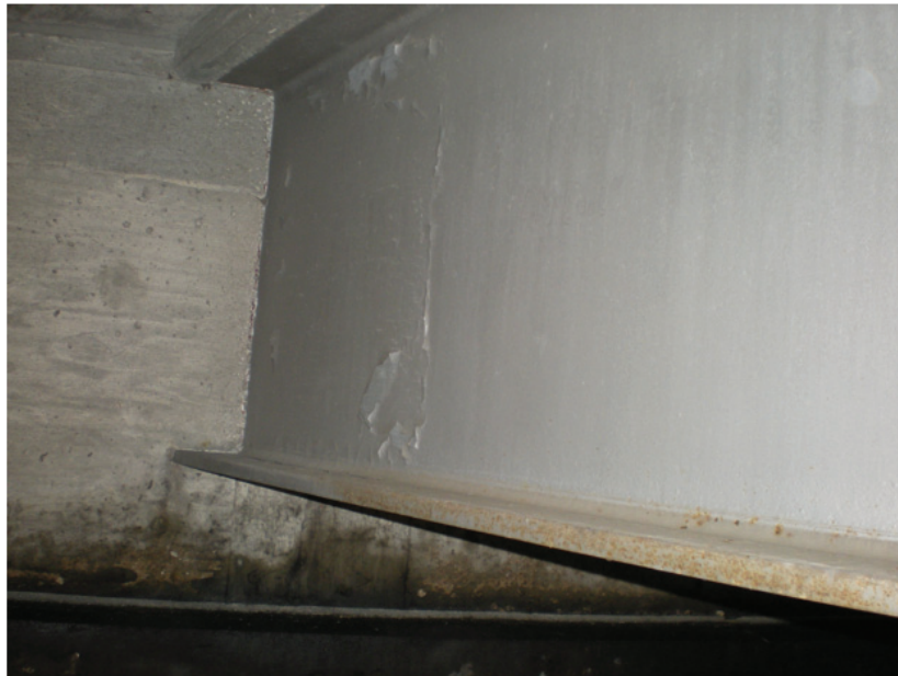
Fair Condition – Interior Beam End-Span
