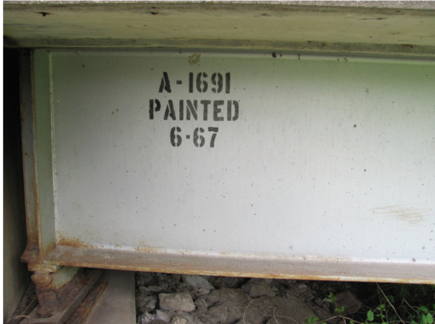
Fair Condition – Exterior Beam End-Span
