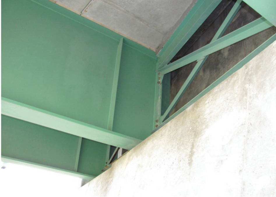
Very Good Condition – Interior Beam End-Span
