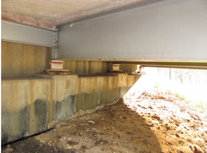
Fair Condition – Interior Beam End-Span
