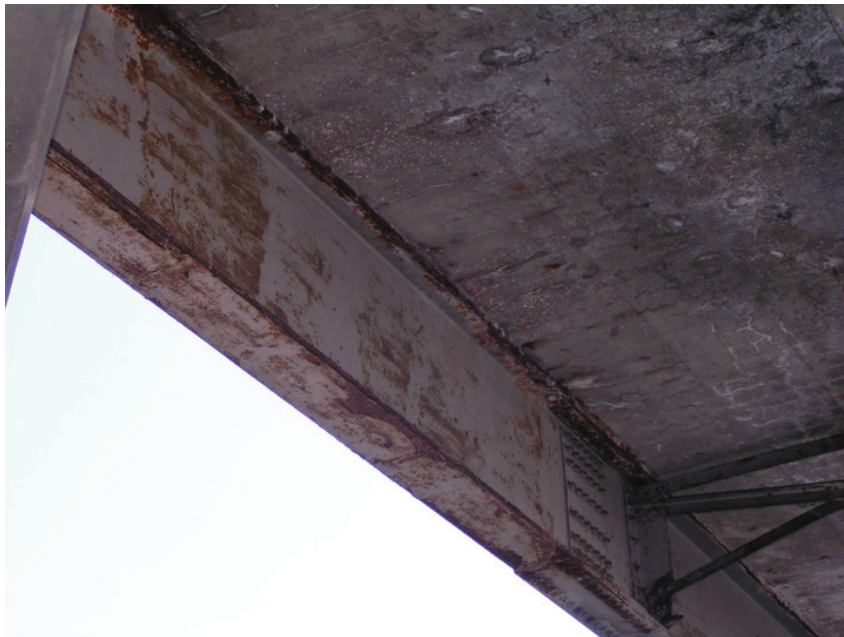
Very Poor Condition – Interior Beam Mid-Span
