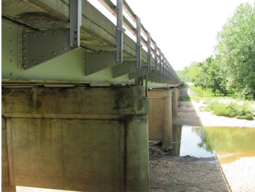
Fair Condition – Fascia Girder Mid-Span
