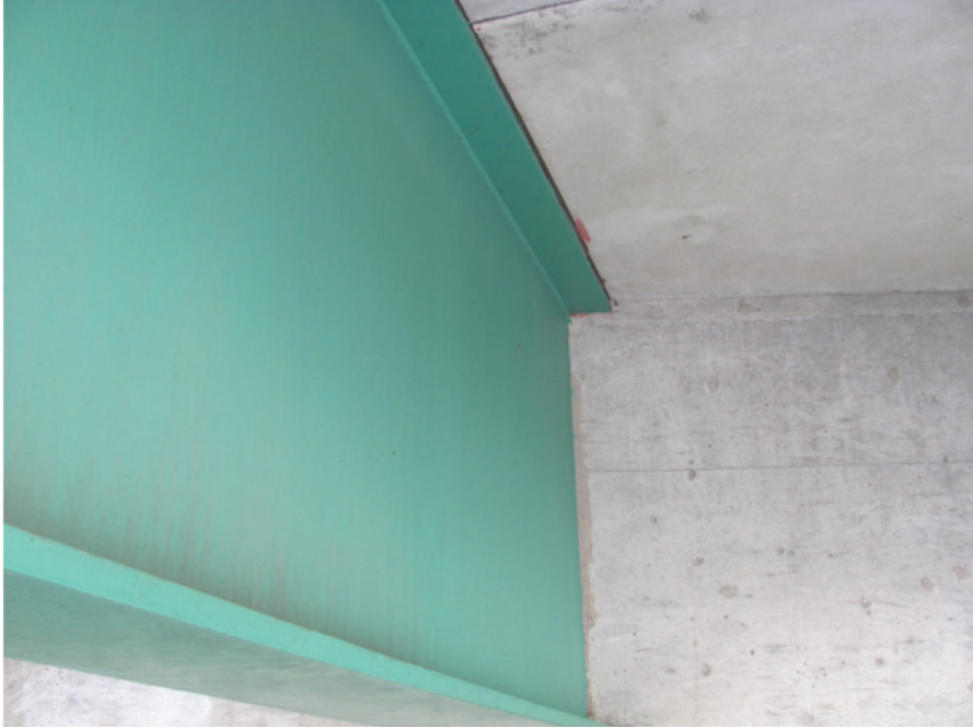
Very Good Condition – Exterior Beam End-Span
