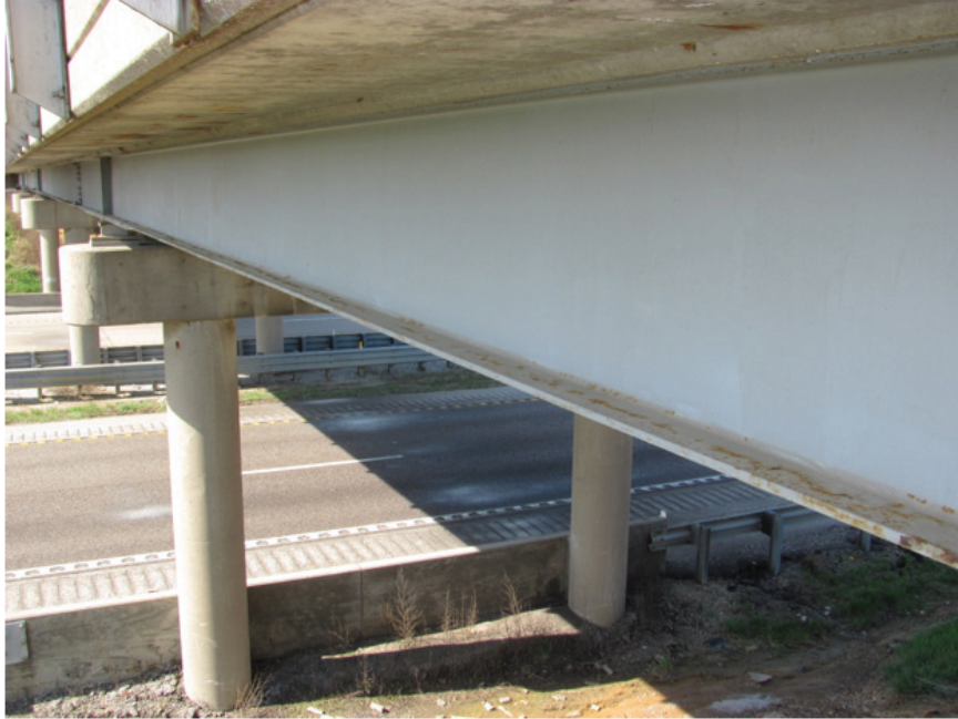
Fair Condition – Facia Girder Mid-Span
