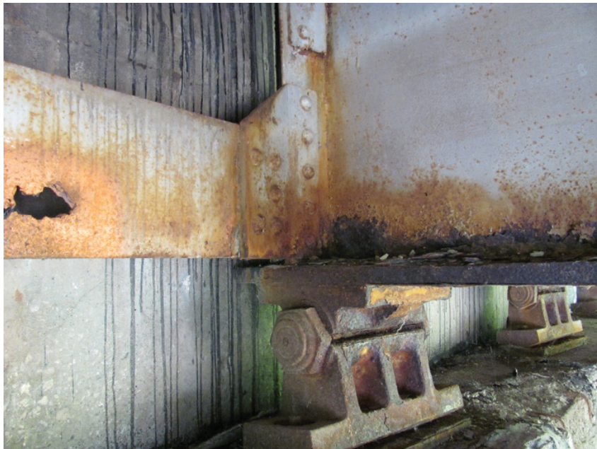
Very Poor Condition – Exterior Beam End-Span
