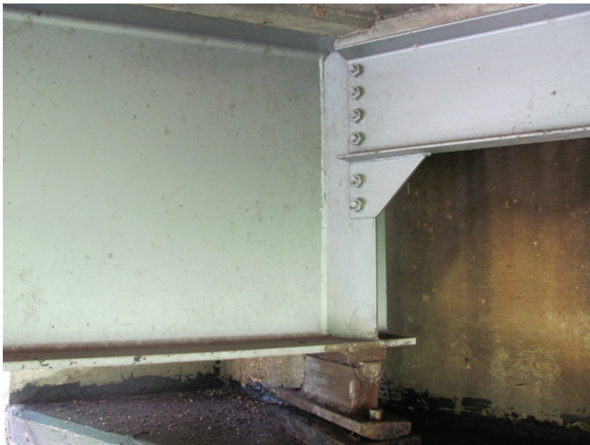
Good Condition – Interior Beam End-Span
