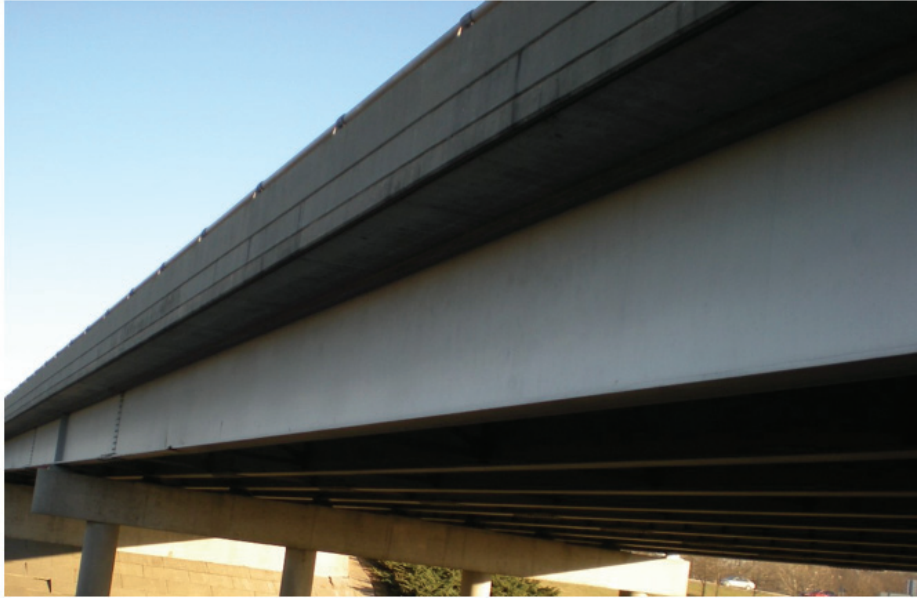
Very Good Condition – Facia Girder Mid-Span
