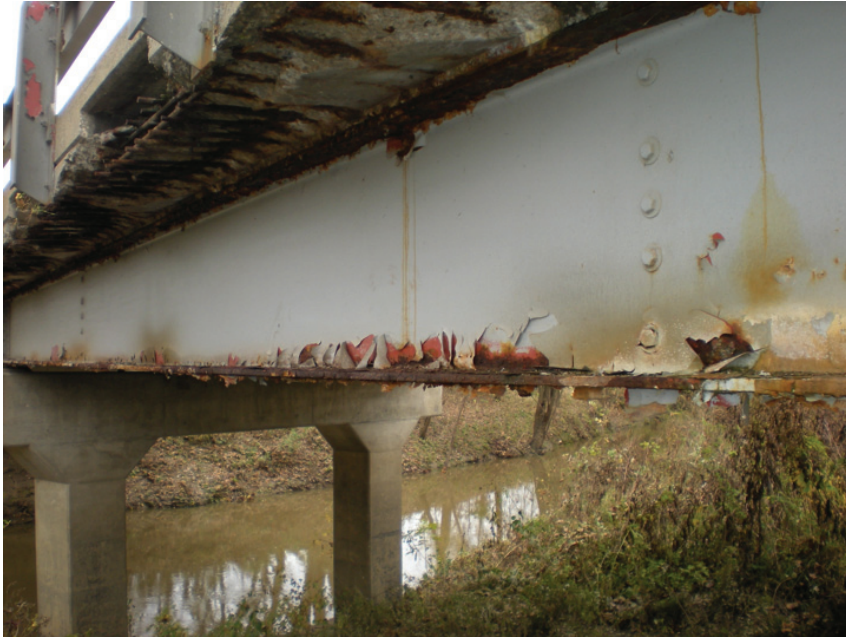
Very Poor Condition – Facia Girder Mid-Span
