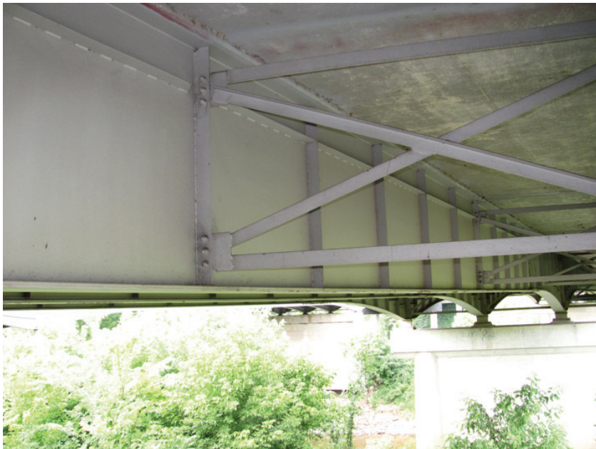
Good Condition – Interior Beam Mid-Span
