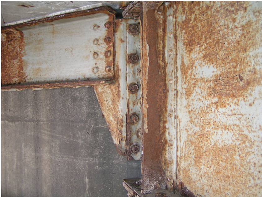
Very Poor Condition – Interior Beam End-Span
