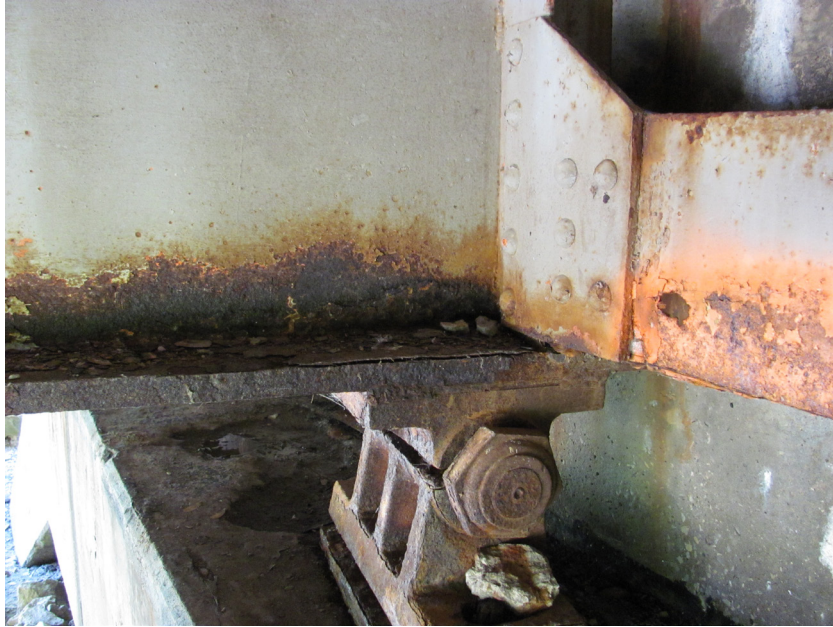
Very Poor Condition – Interior Beam End-Span
