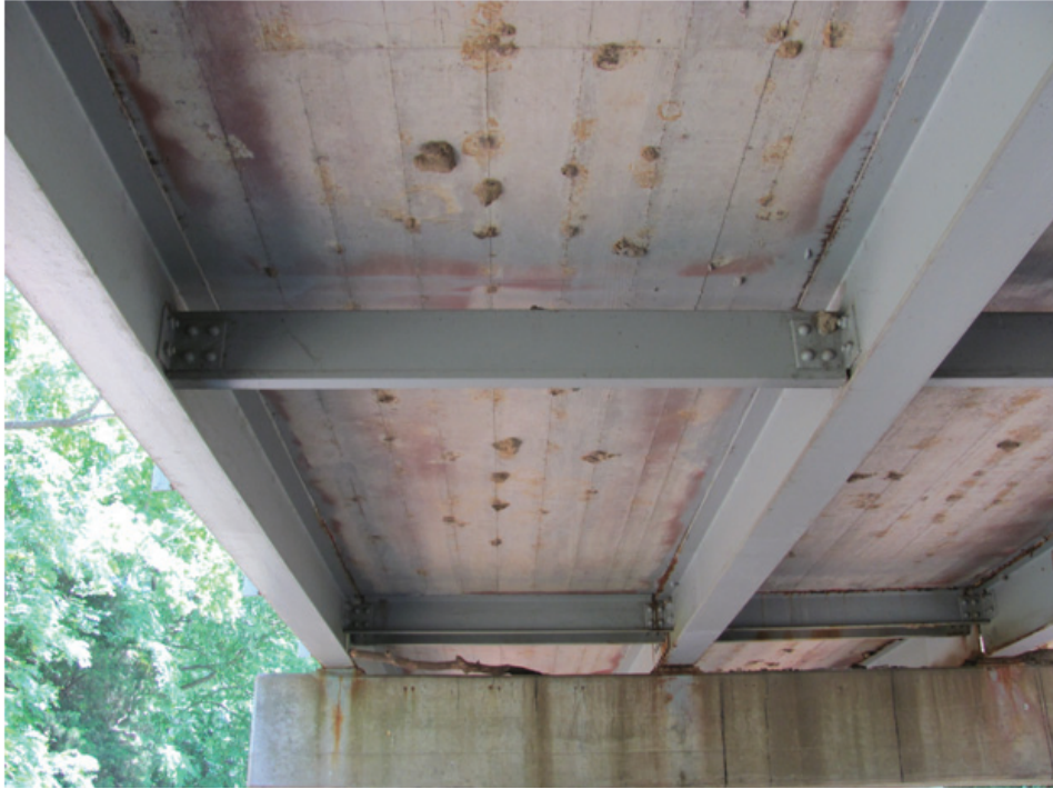
Fair Condition – Interior Beam Mid-Span
