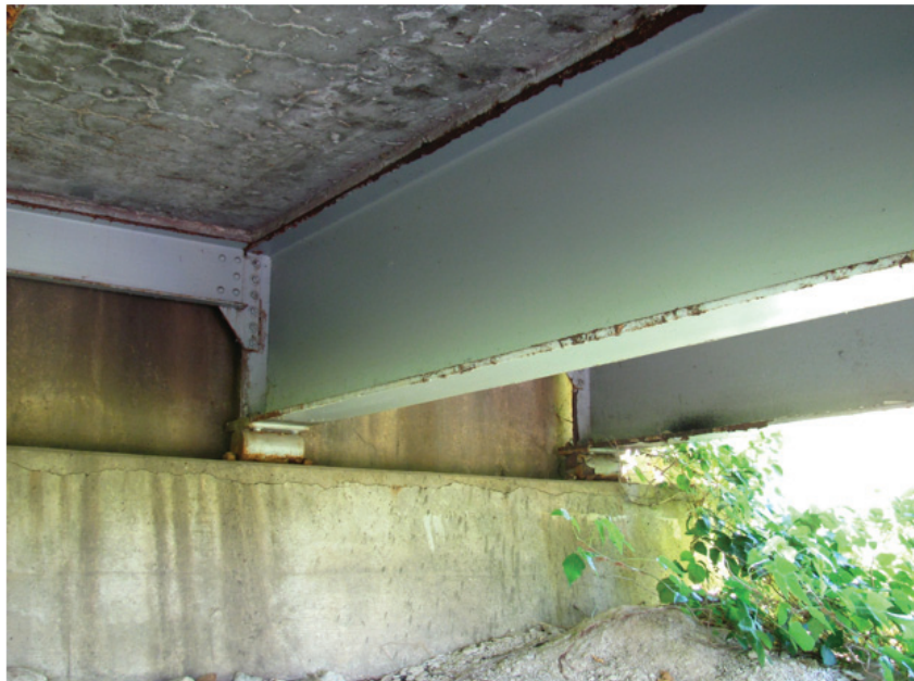
Fair Condition – Interior Beam End-Span
