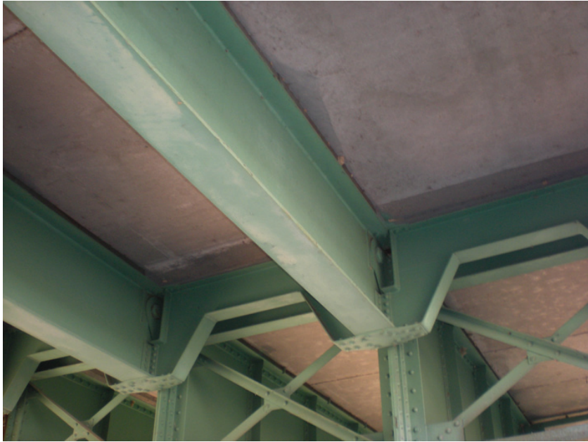
Good Condition – Interior Beam Mid-Span
