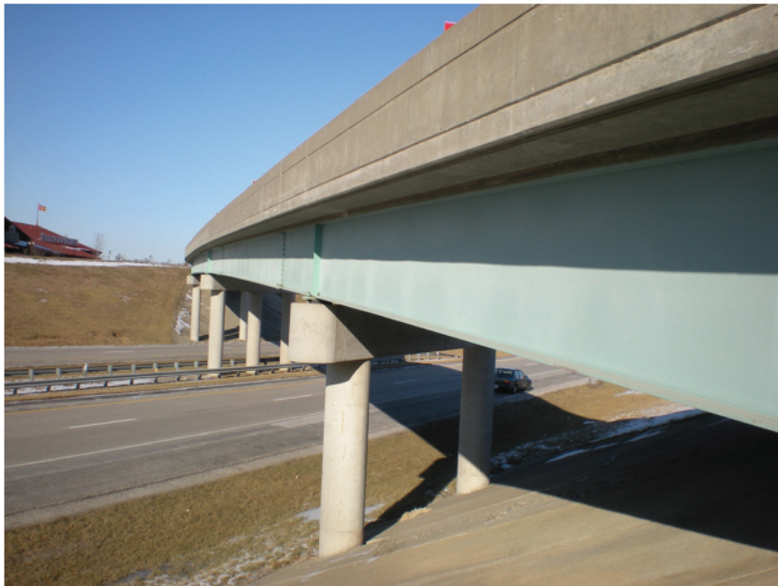
Very Good Condition – Facia Girder Mid-Span
