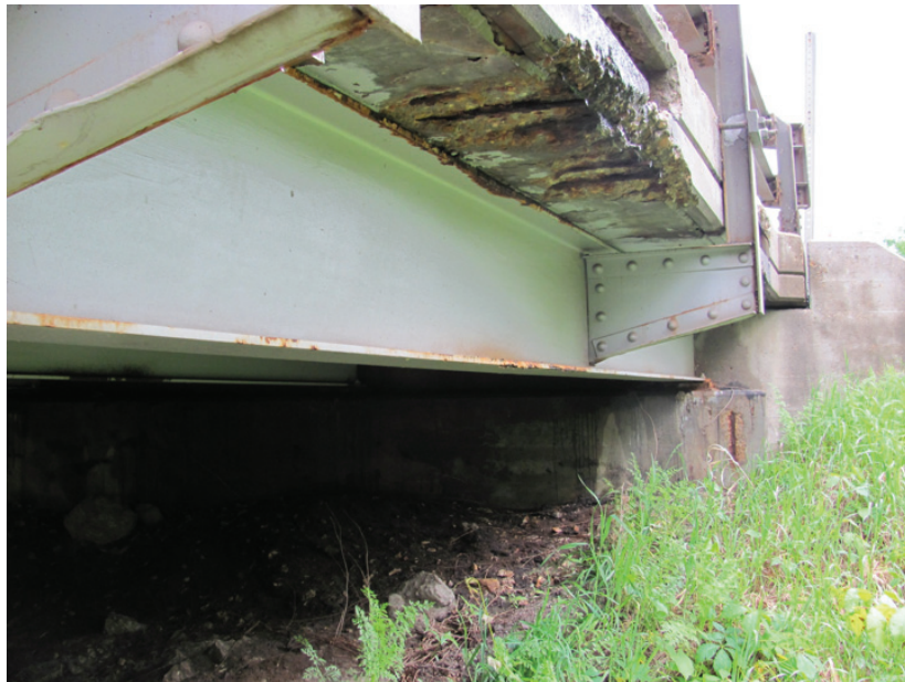
Poor Condition – Exterior Beam End-Span
