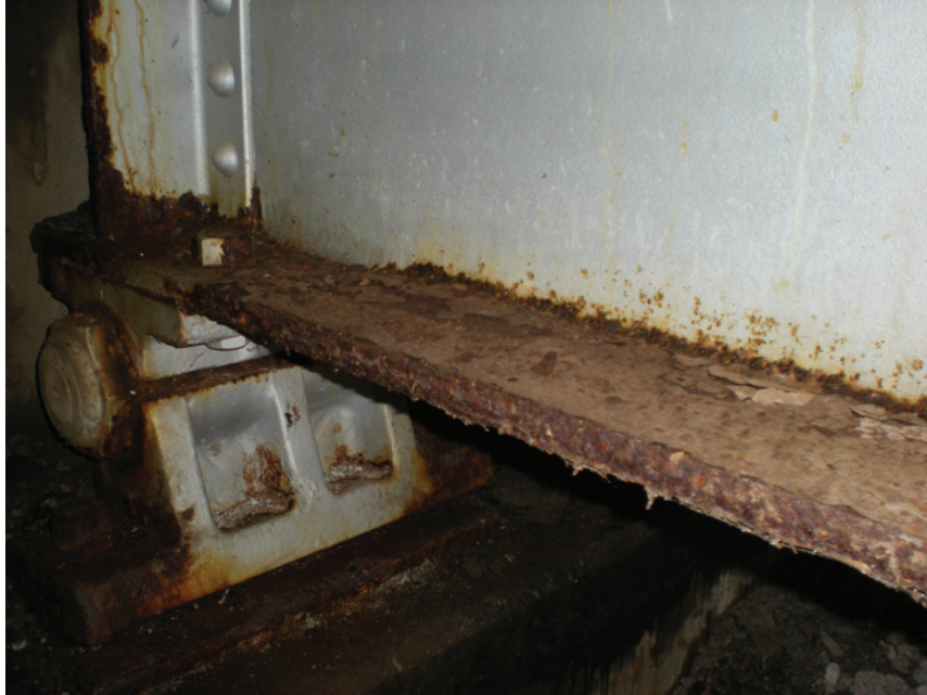
Very Poor Condition – Exterior Beam End-Span
