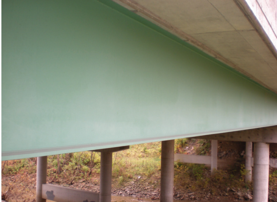
Very Good Condition – Facia Girder Mid-Span
