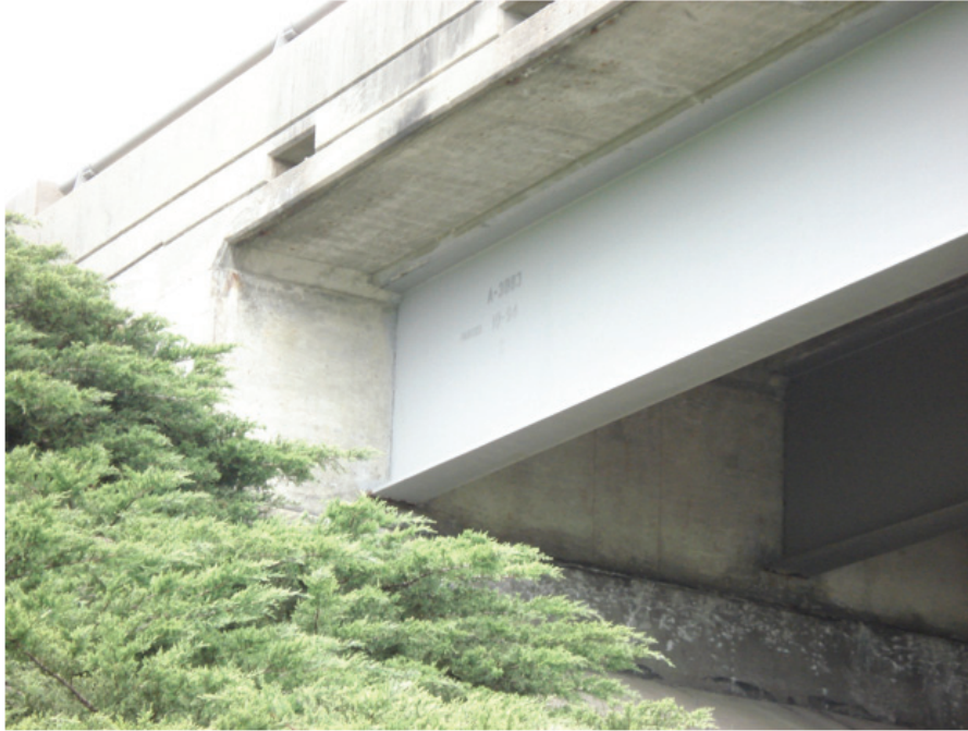
Very Good Condition – Exterior Beam End-Span
