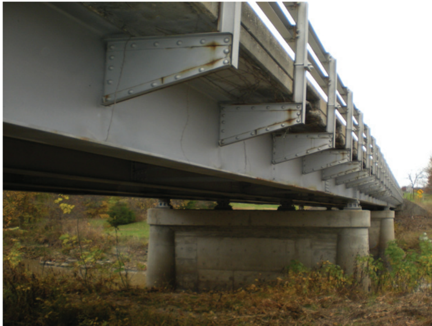
Fair Condition – Facia Girder Mid-Span
