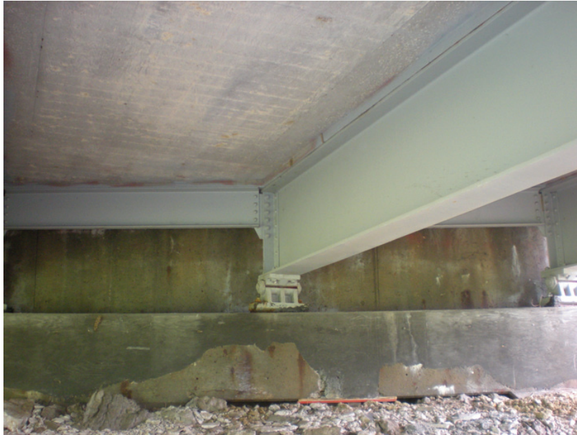
Good Condition – Interior Beam End-Span
