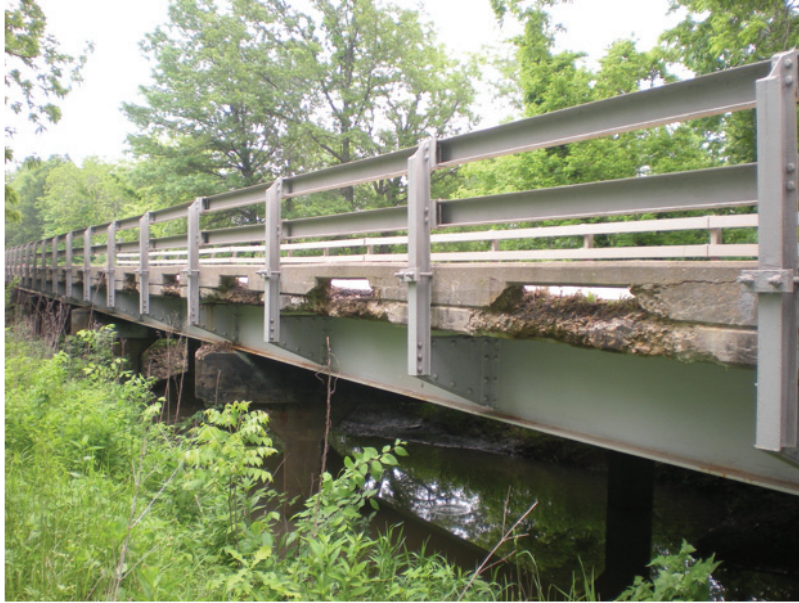
Fair Condition – Fascia Girder Mid-Span
