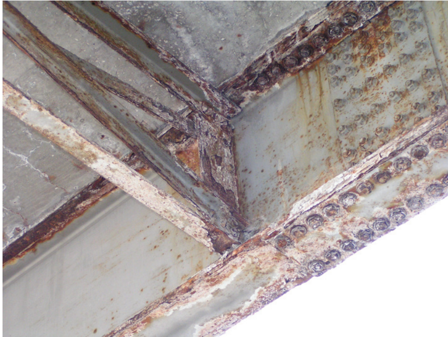
Very Poor Condition – Close-up
