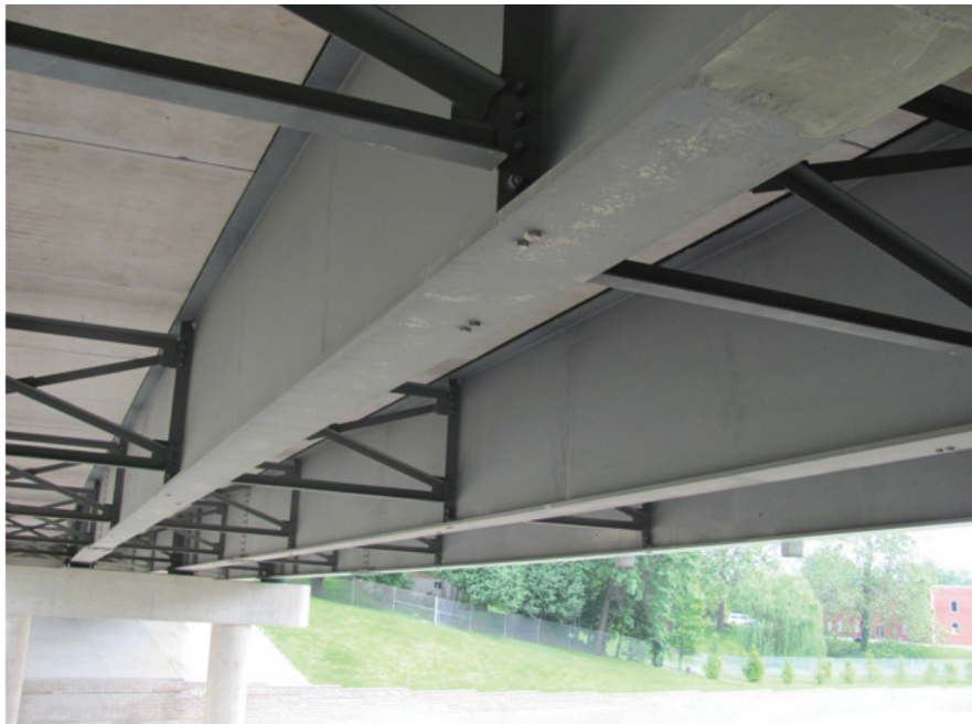
Very Good Condition – Interior Beam Mid-Span
