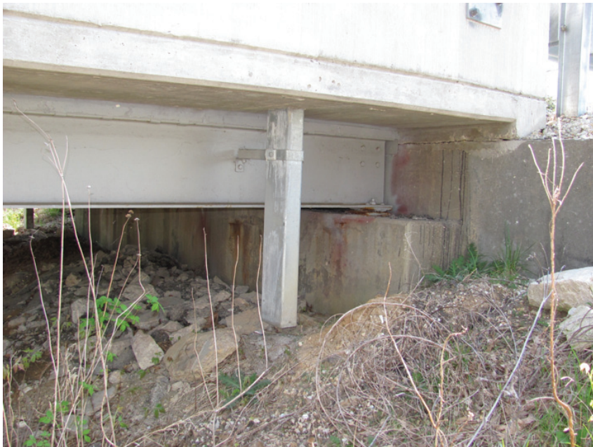
Good Condition – Exterior Beam End-Span
