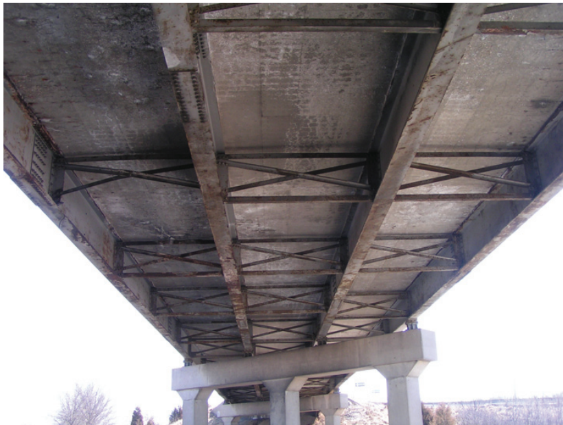
Very Poor Condition – Interior Beam Mid-Span
