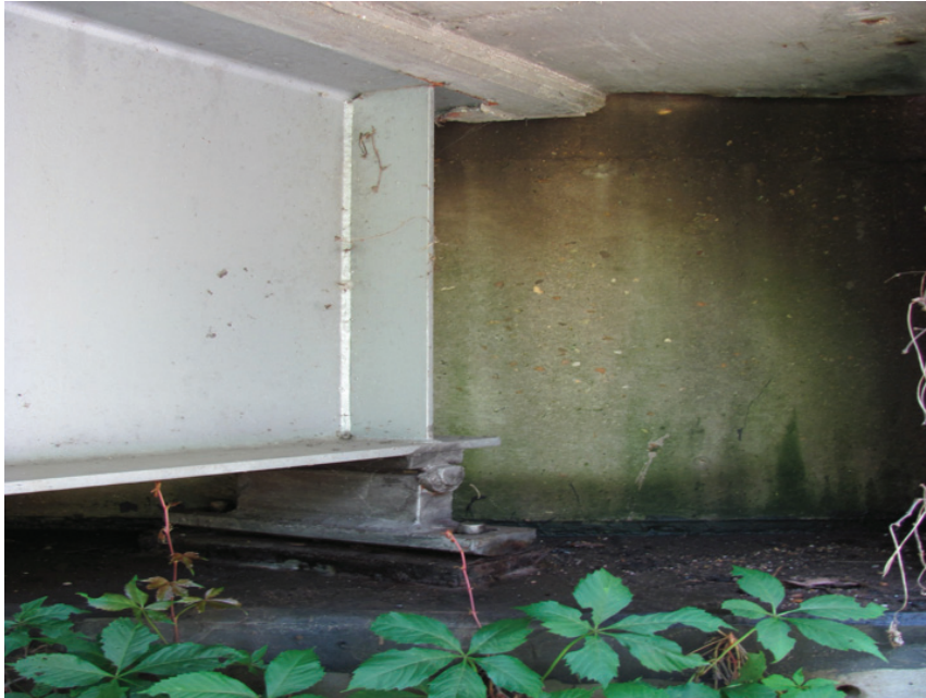
Good Condition – Exterior Beam End-Span
