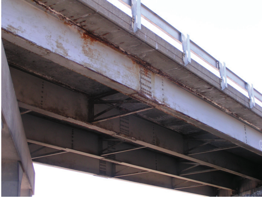
Very Poor Condition – Facia Girder Mid-Span
