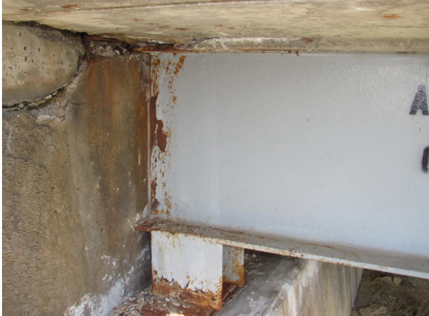
Poor Condition – Interior Beam End-Span
