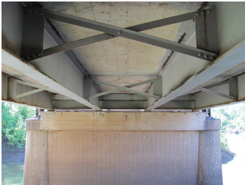
Poor Condition – Interior Beam Mid-Span
