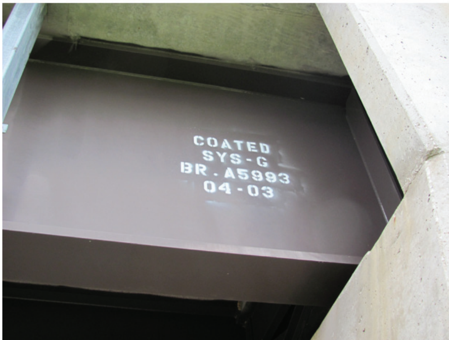
Very Good Condition – Exterior Beam End-Span
