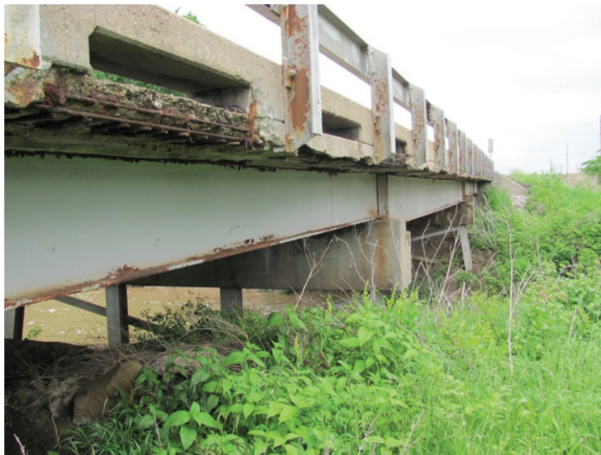
Poor Condition – Facia Girder Mid-Span
