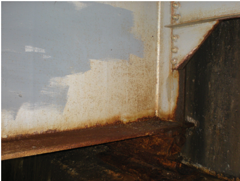
Very Poor Condition – Interior Beam End-Span
