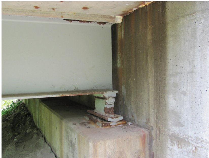
Fair Condition – Exterior Beam End-Span
