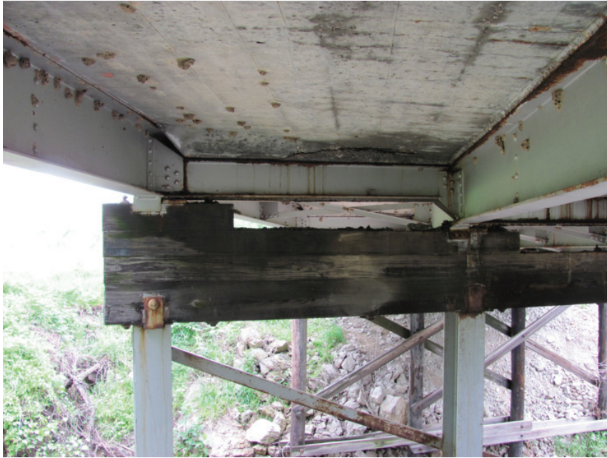
Poor Condition – Interior Beam Mid-Span
