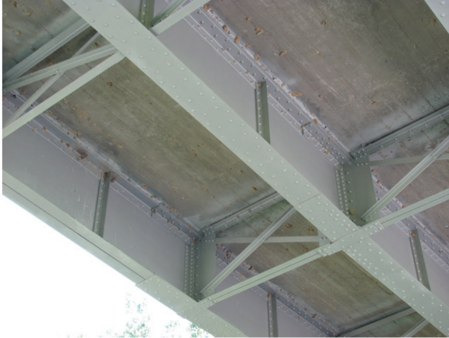
Very Good Condition – Interior Beam Mid-Span
