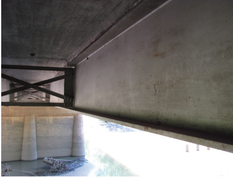
Fair Condition – Interior Beam Mid-Span
