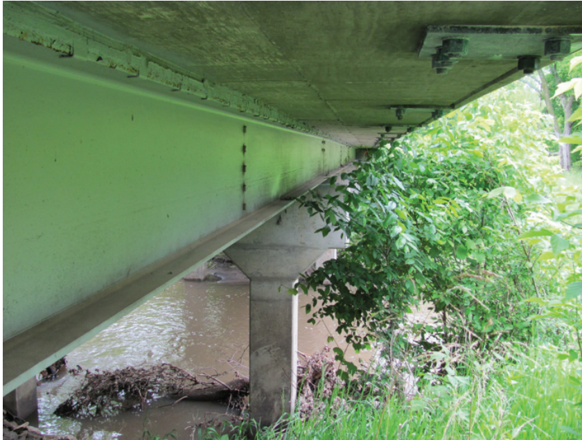
Good Condition – Facia Girder Mid-Span
