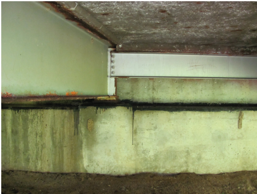
Poor Condition – Interior Beam End-Span
