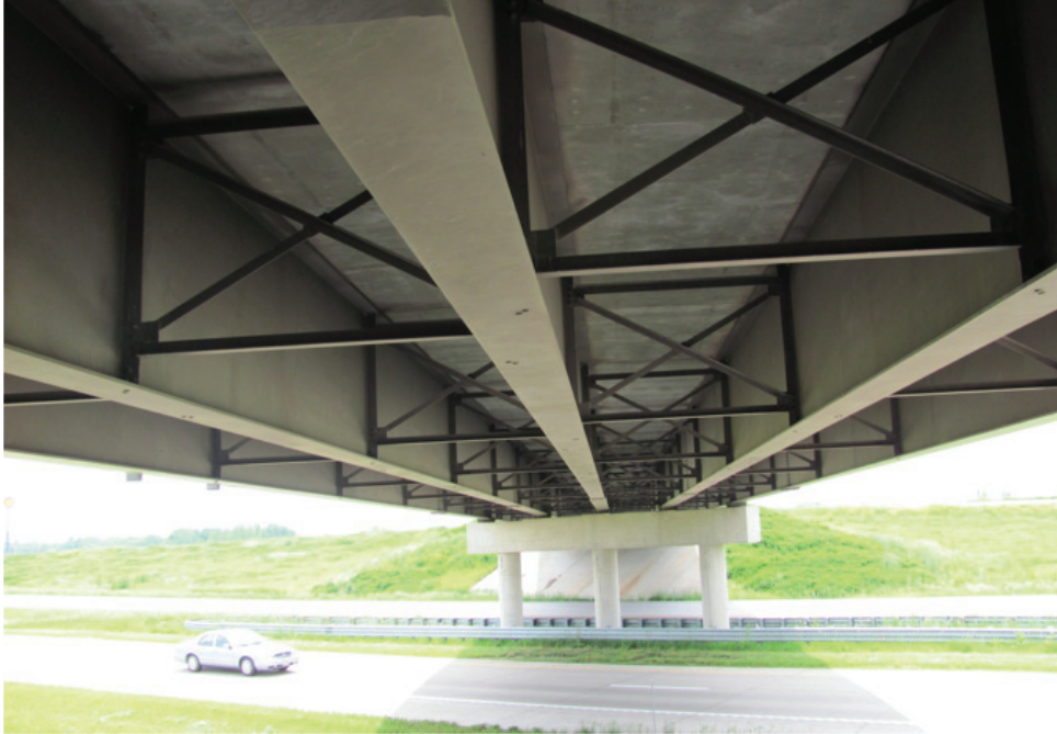
Very Good Condition – Interior Beam Mid-Span
