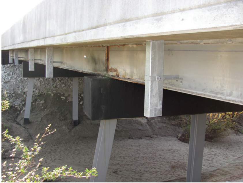
Poor Condition – Facia Girder Mid-Span
