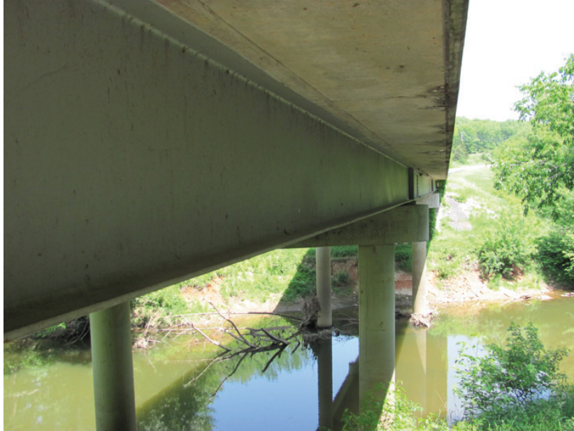
Good Condition – Facia Girder Mid-Span
