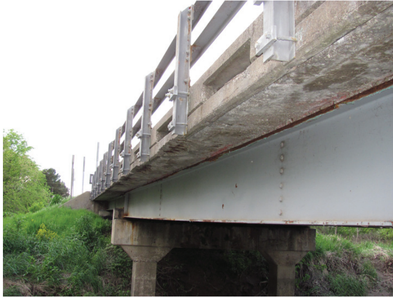
Poor Condition – Facia Girder Mid-Span
