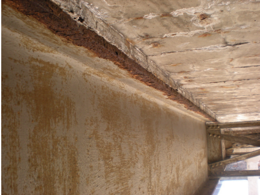
Very Poor Condition – Interior Beam Mid-Span
