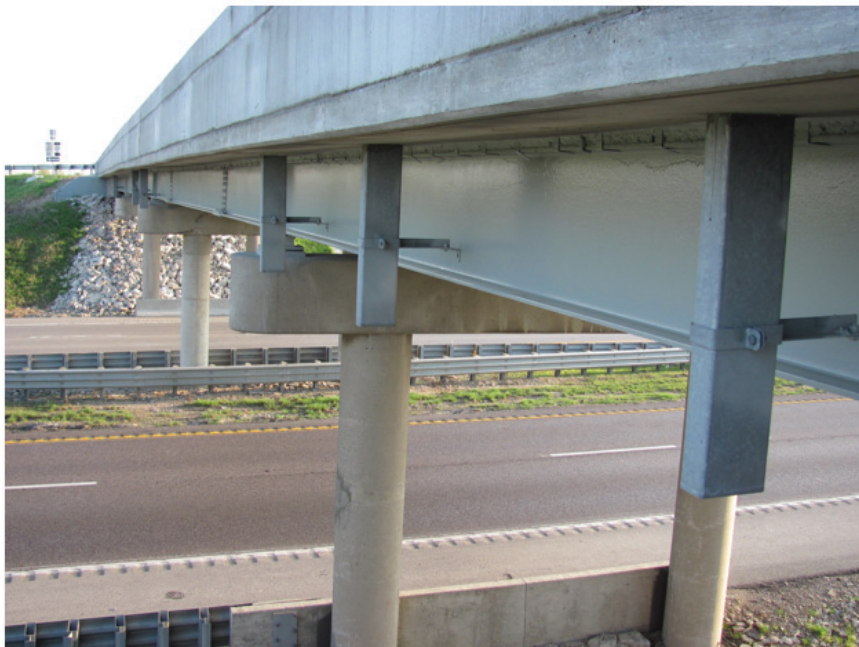
Very Good Condition – Facia Girder Mid-Span
