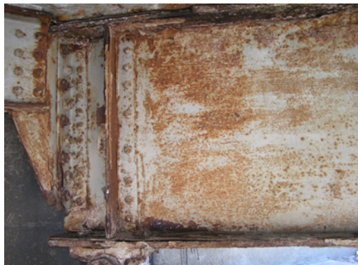
Figure 3.5 Example Photograph for Interior Sections of a Bridge with Coatings in Very Poor Condition.
