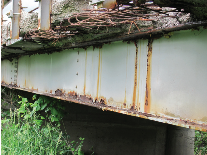
Very Poor Condition – Fascia Girder Mid-Span
