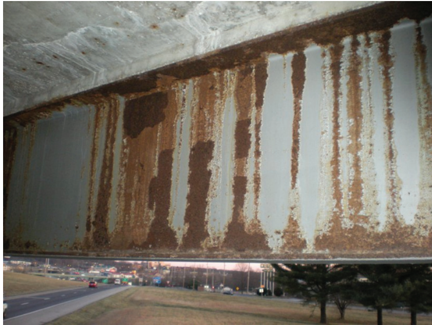
Very Poor Condition – Interior Beam Mid-Span
