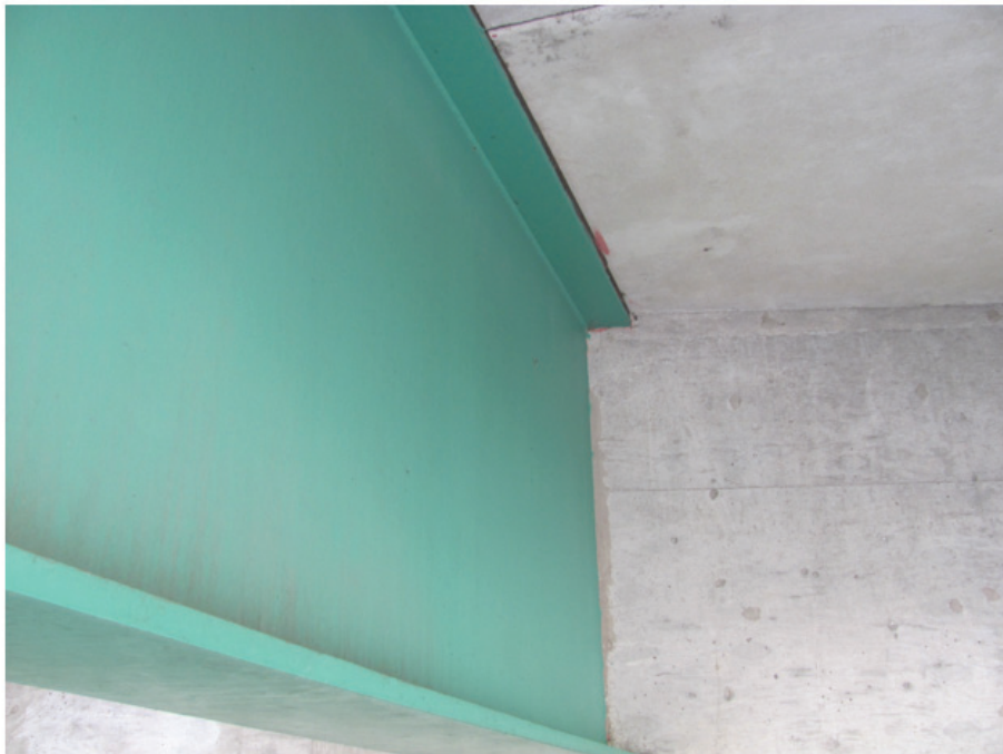
Very Good Condition – Interior Beam End-Span
