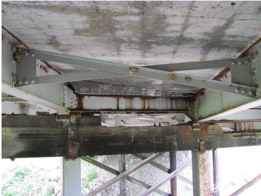
Very Poor Condition – Interior Beam Mid-Span
