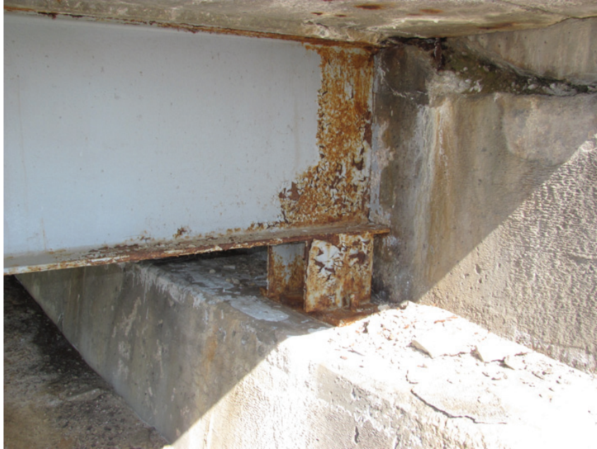
Poor Condition – Exterior Beam End-Span
