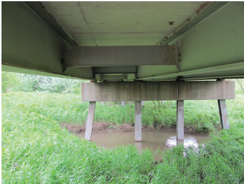
Fair Condition – Interior Beam Mid-Span
