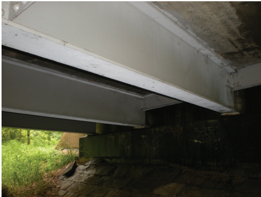
Good Condition – Interior Beam End-Span
