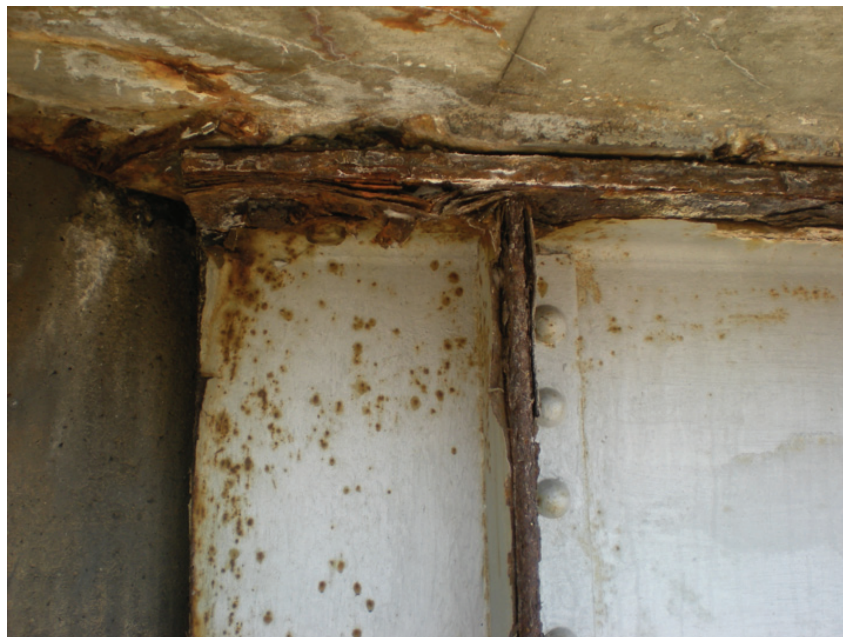
Very Poor Condition – Exterior Beam End-Span
