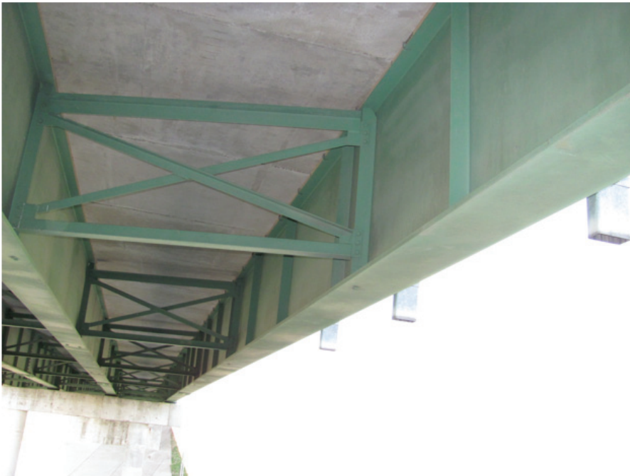
Very Good Condition – Interior Beam Mid-Span
