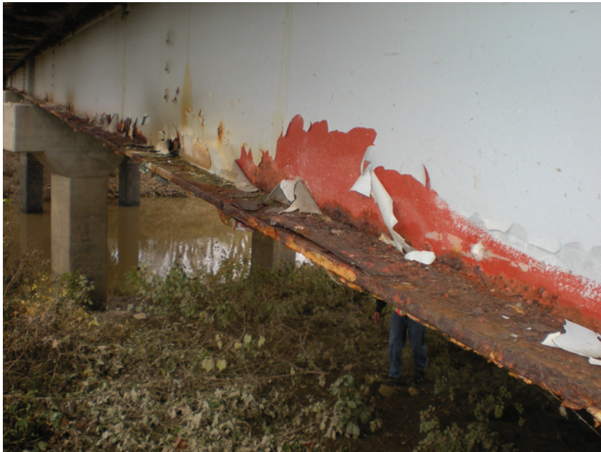
Very Poor Condition – Facia Girder Mid-Span
