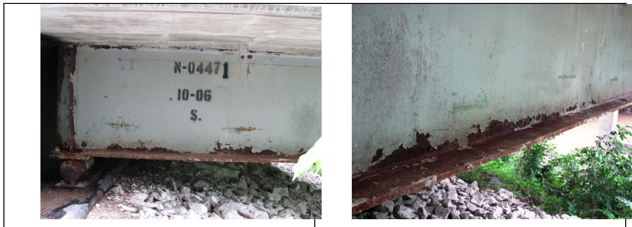
Figure 4.2 Example of System S Coating with Early Failure, End-span of Fascia Girder.
