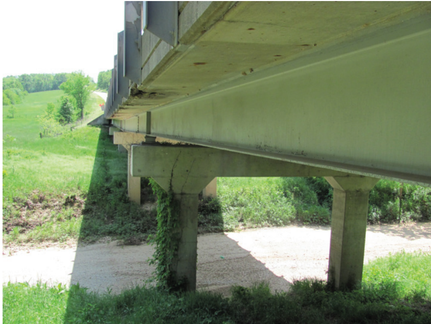
Good Condition – Facia Girder Mid-Span
