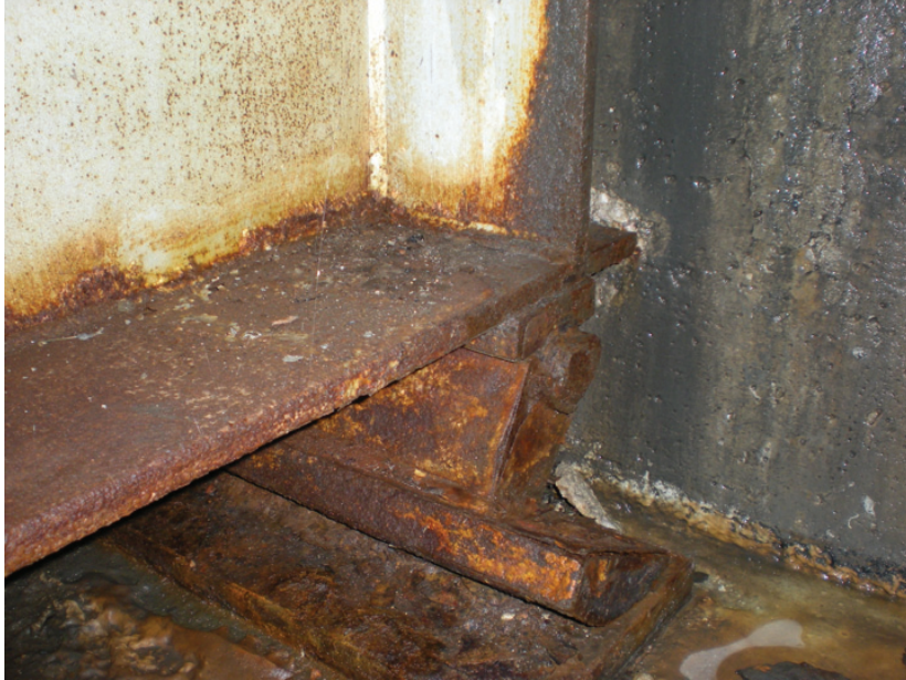
Very Poor Condition – Interior Beam End-Span
