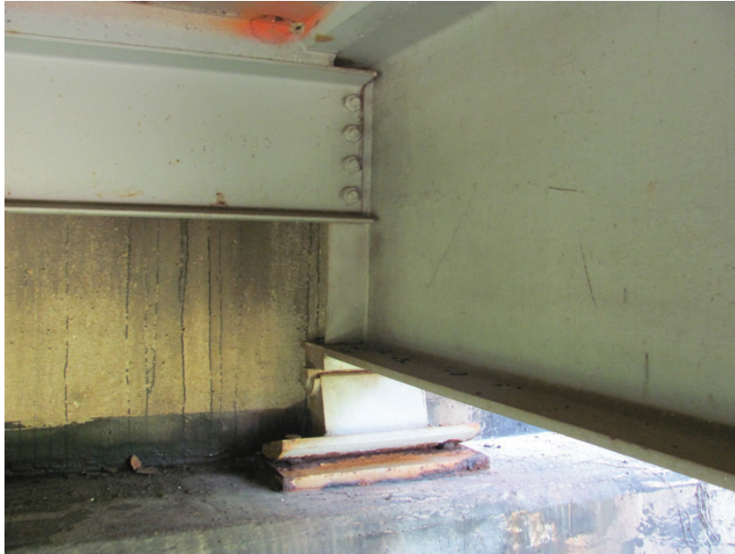
Good Condition – Interior Beam End-Span
