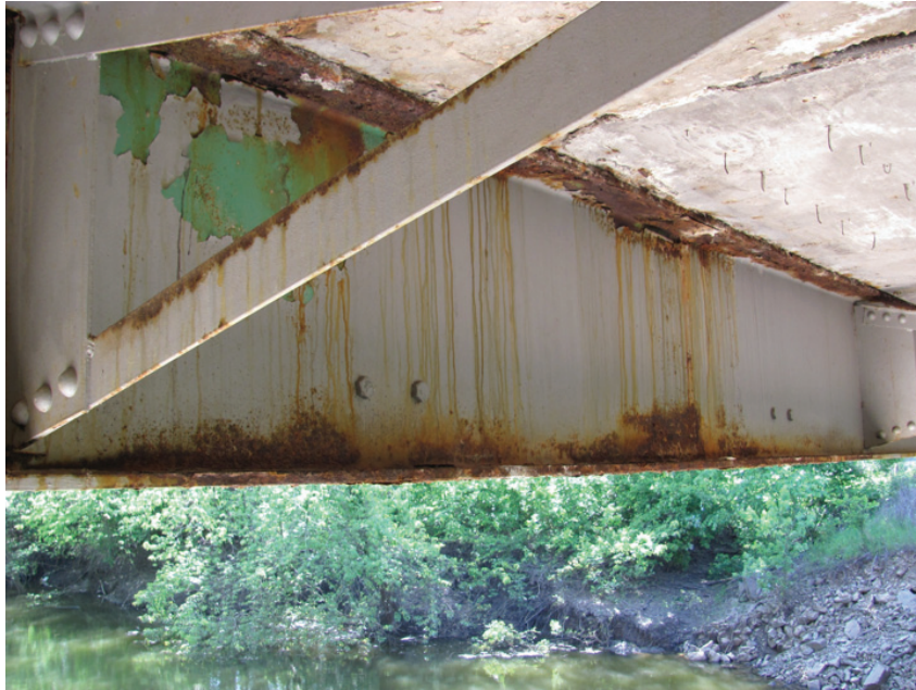
Very Poor Condition – Interior Beam Mid-Span
