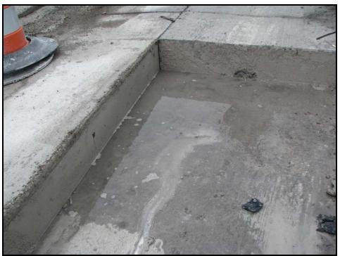
FIGURE 10 Exposed Lean Concrete Base of Euro-Pavement (Note Standing Water)
