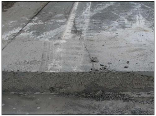
FIGURE 5 Typical Longitudinal Crack with Euro-Pavement
