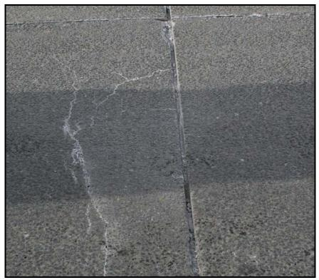
FIGURE 7 Beginning Spall of Euro-Pavement Note: White substance in crack is salt (de-icing) residue.
