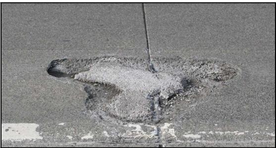
FIGURE 9 High Severity Spall/Delamination of Euro-Pavement
