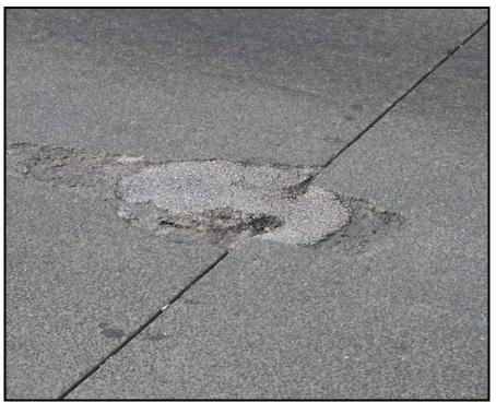
FIGURE 8 Spall on Both Sides of Transverse Joint of Euro-Pavement
