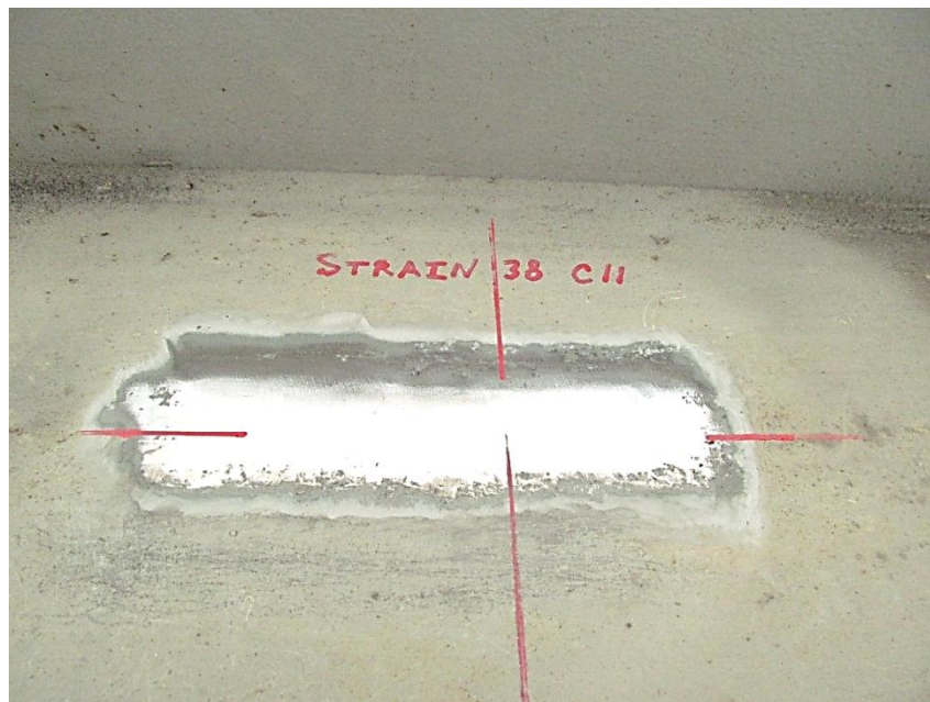
Figure 13. Metal Preparation: Grind and Mark the Sensor Location
