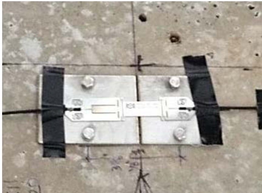
Figure 19. Spot Welded Strain Sensor on Steel Plate
