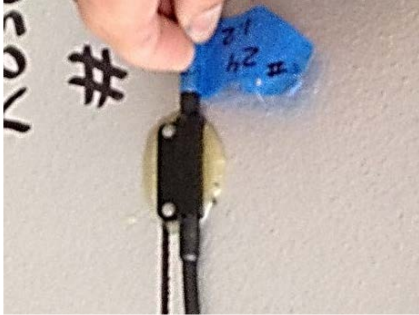
Figure 24. Using Epoxy to mount Temperature Sensor
