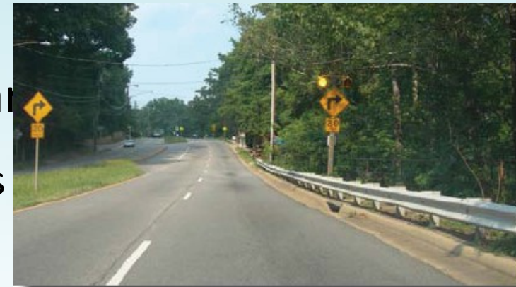
Doubling-up of the sign proved effective at this site because tree limbs partially blocked the right side sign.
