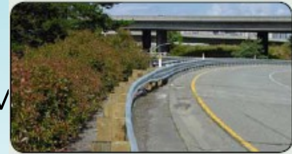
After: The replacement guardrail meets current safety standards, and creates a continuous transition to the bridge rail, removing the blunt end that had existed previously.
