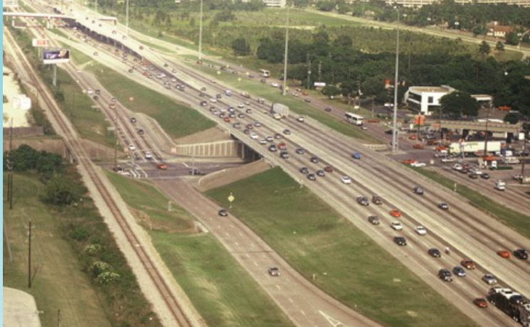
IH10 at SH 6, Before Construction
