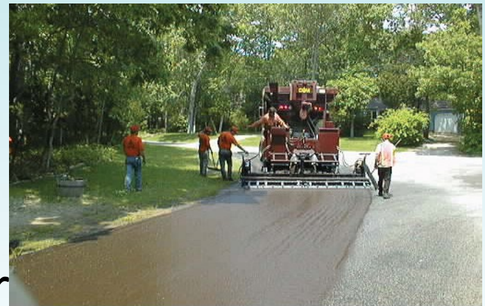
Application of skid-resistant pavement surface in curve.
