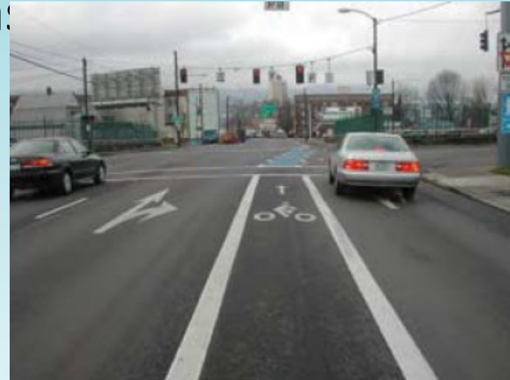
Example of blue bike lane between right turn lane and shared right-through lane (Portland, OR)
