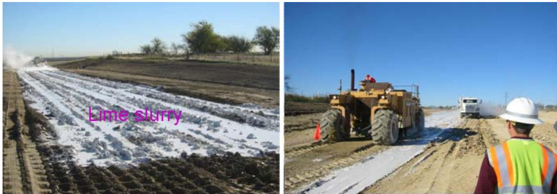
Figure 3-1. Lime Treatment Process on SH 114.
