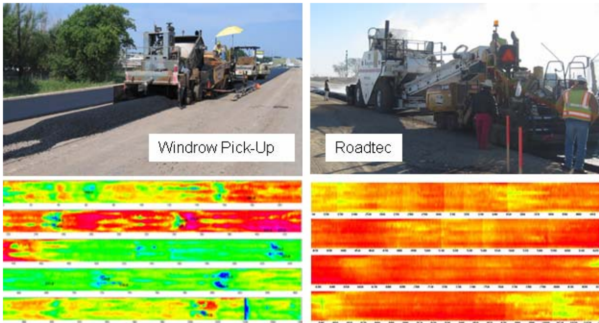
Figure 3-3. Comparison of MTDs and HMA Mat Temperature Profiles on SH 114 (Red \cong 300 °F [Good], 235 °F \leq Green \leq 270 °F, Blue \cong 220 °F [Thermal Segregation]).
