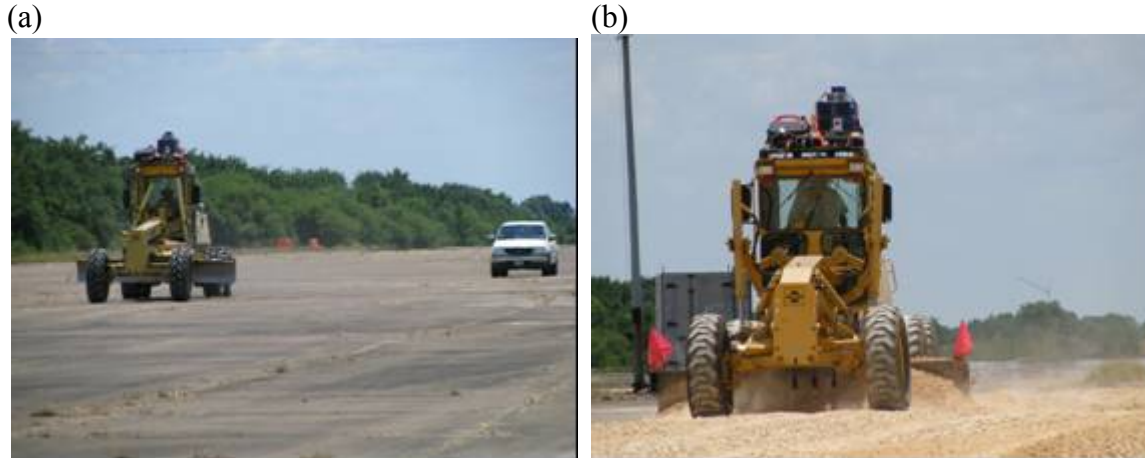
Figure 15. Pictures of (a) Driving Testing and (b) Leveling Testing.
