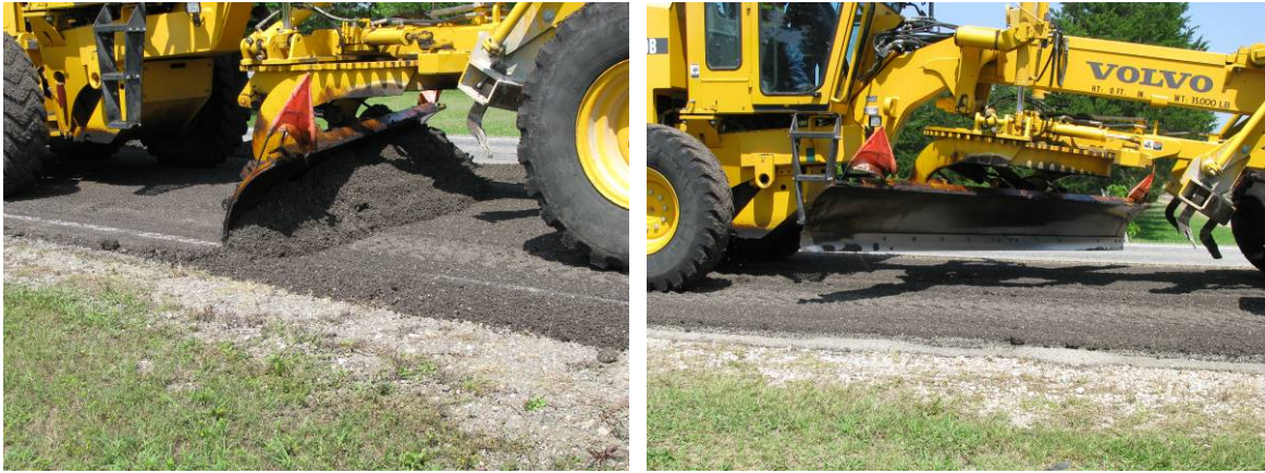
Figure 4. Grader Blade Position in Forward (Left) and Backward (Right) Movements.
