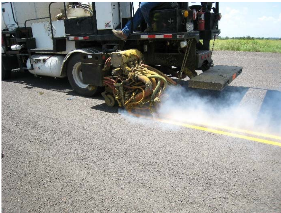
Figure 24. SH 21 Lead-Free Thermoplastic Installation.
