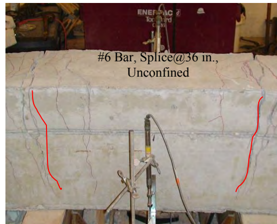
(j) Flexural failure of B-6-8
