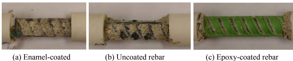
Figure 4.19 Details of concrete-rebar interfaces (#4 rebar).
