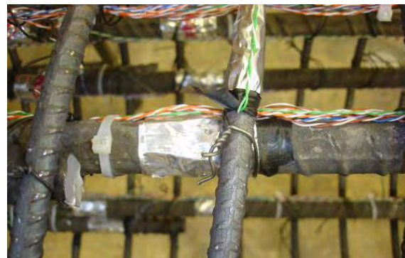
(b) Gauges on main and spiral reinforcement
