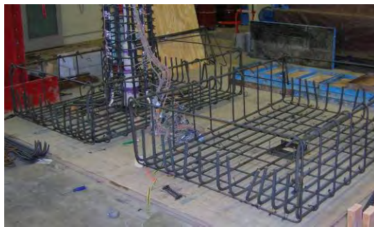
(a) Footing reinforcement cage
