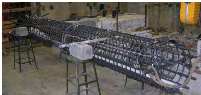
(b) Column reinforcement cage
