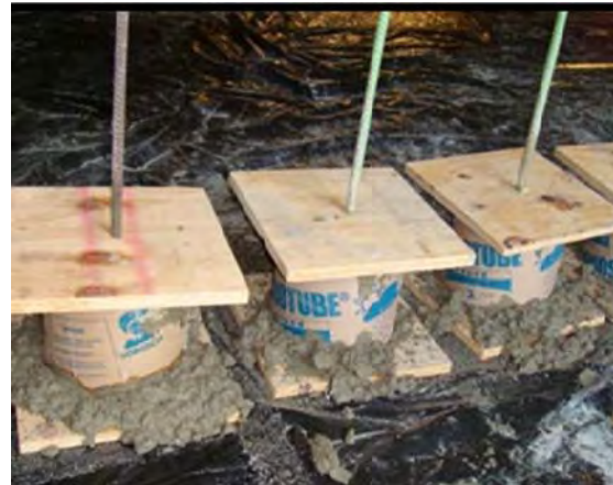
(b) Completion of casting
