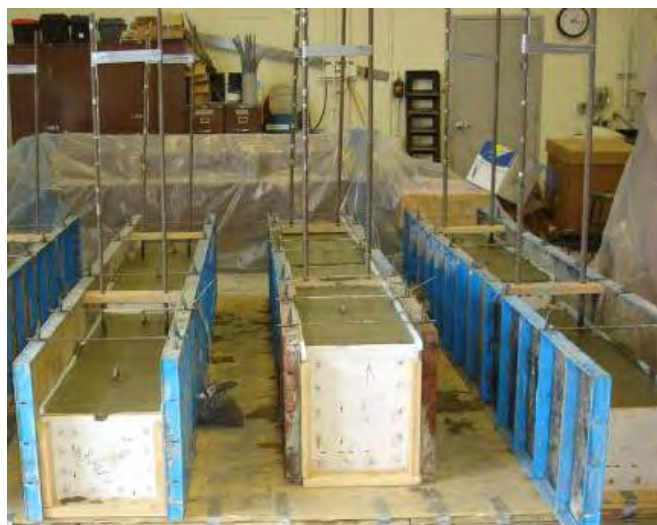
(b) Steel formwork and concrete casting
