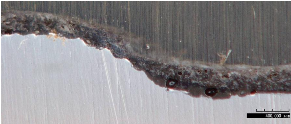
(c) Thin portion of double coating on a deformed rebar showing no distinct boundary
