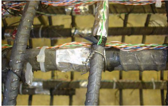
(b) Gauges on main and spiral reinforcement
