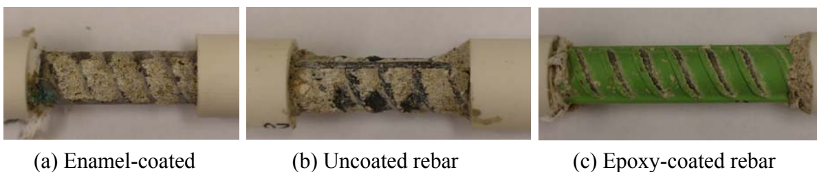
Figure 4.19 Details of concrete-rebar interfaces (#4 rebar).
