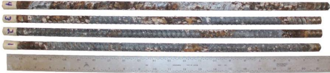
Figure 6.45 Uncoated reinforcing bars after removal from a ponding specimen.
