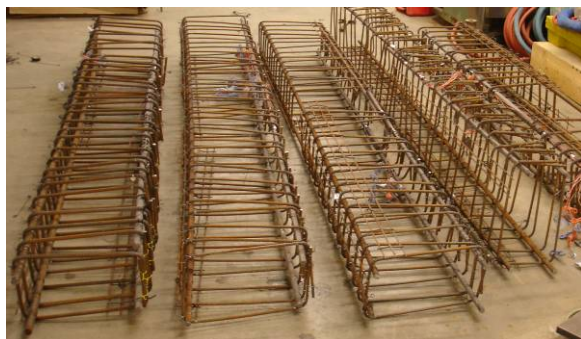
(a) Rebar cage of beams
