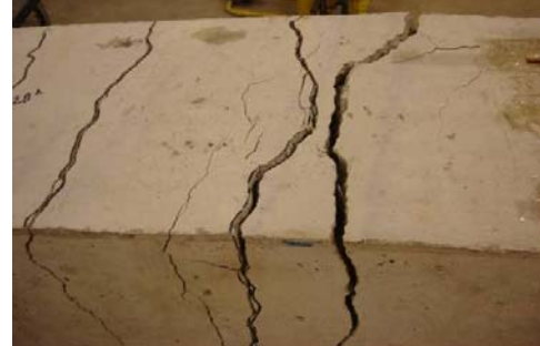
(c) Cracks at failure
