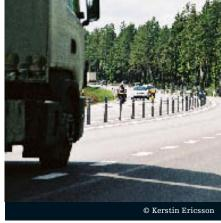
• A new and widely discussed innovation is the **2+1 lane highway with a median barrier,** a road type developed in Sweden.
