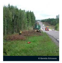
• Major investments have been made to **minimise the damage** ensuing from cars veering off the road. Guard rails have been erected, and potentially dangerous objects such as trees and boulders have been cleared away from roadside areas.
