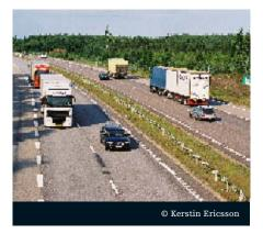
• **Speed limits** on parts of the road network have been reviewed in order to ensure that they reflect the safety standard of the road. For example, it is now quite unusual to find a road with a speed of 110 km/h without a median barrier.
