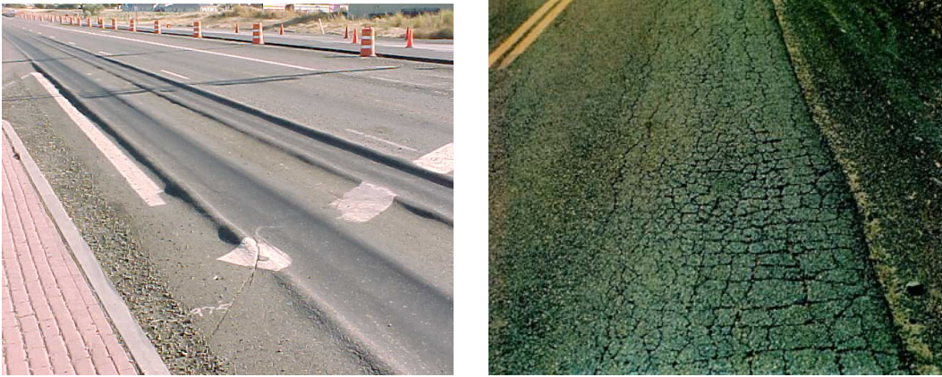
Figure 1 Distresses in flexible pavements (a) rutting (b) fatigue cracking
