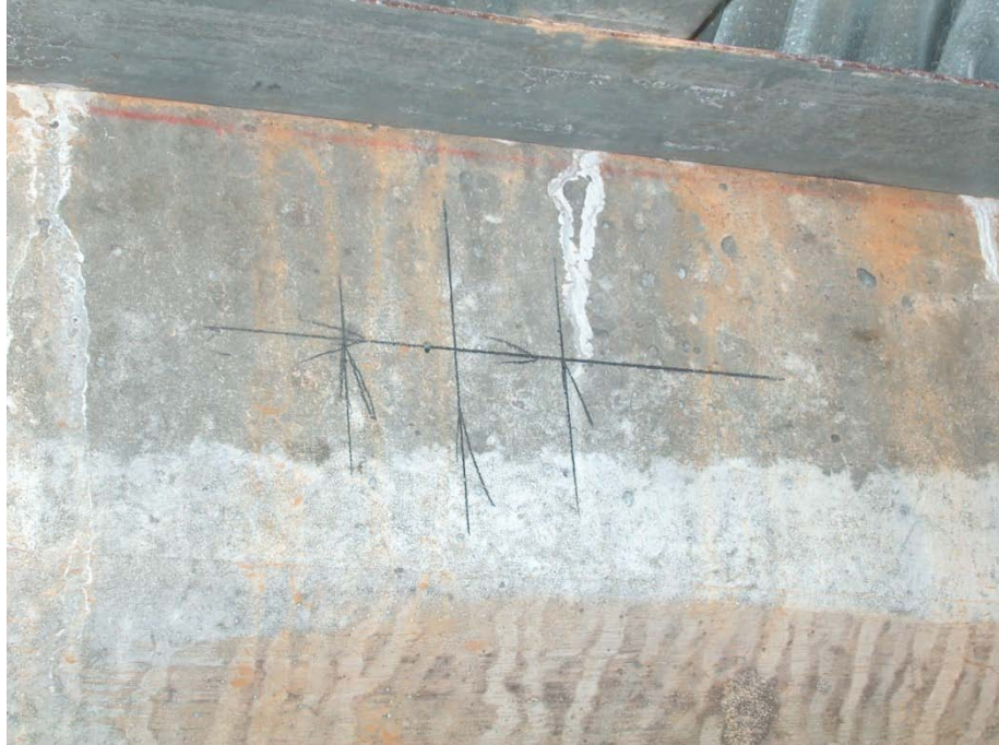
Figure 177 Initial marking on the girder for placing transducer
