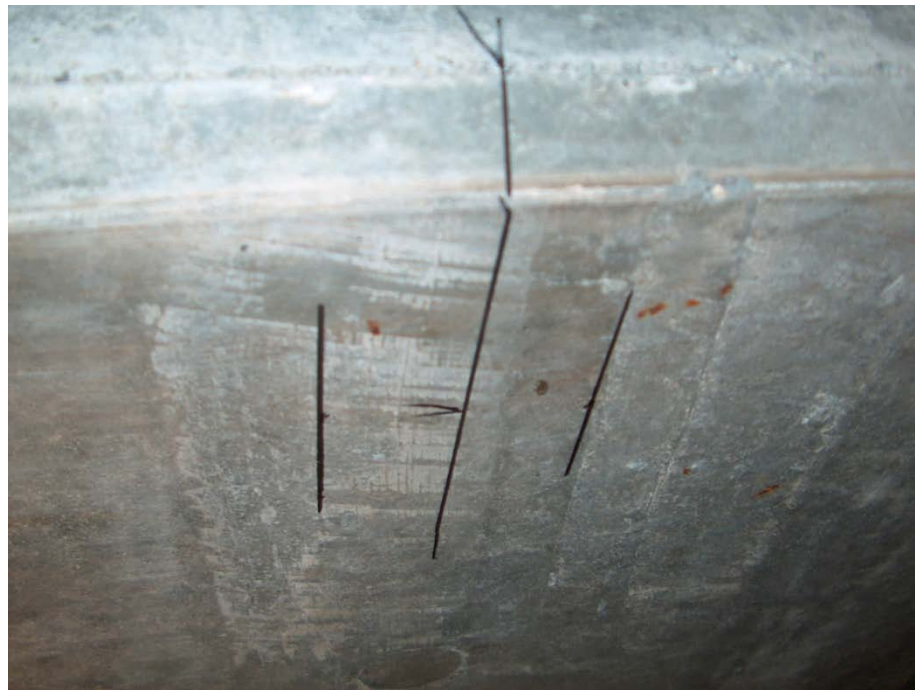
Figure 174 Initial marking on the girder for placing transducer
