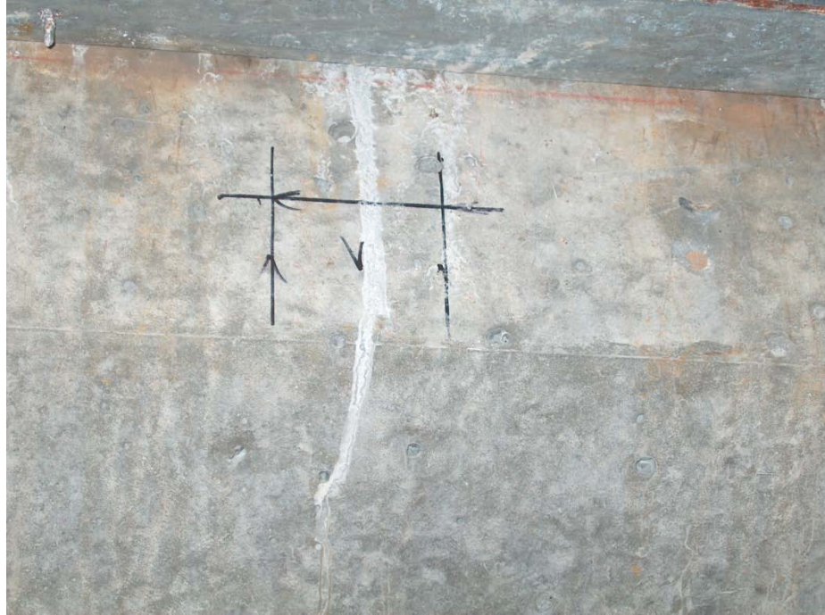
Figure 165 Initial marking on the girder for placing transducer
