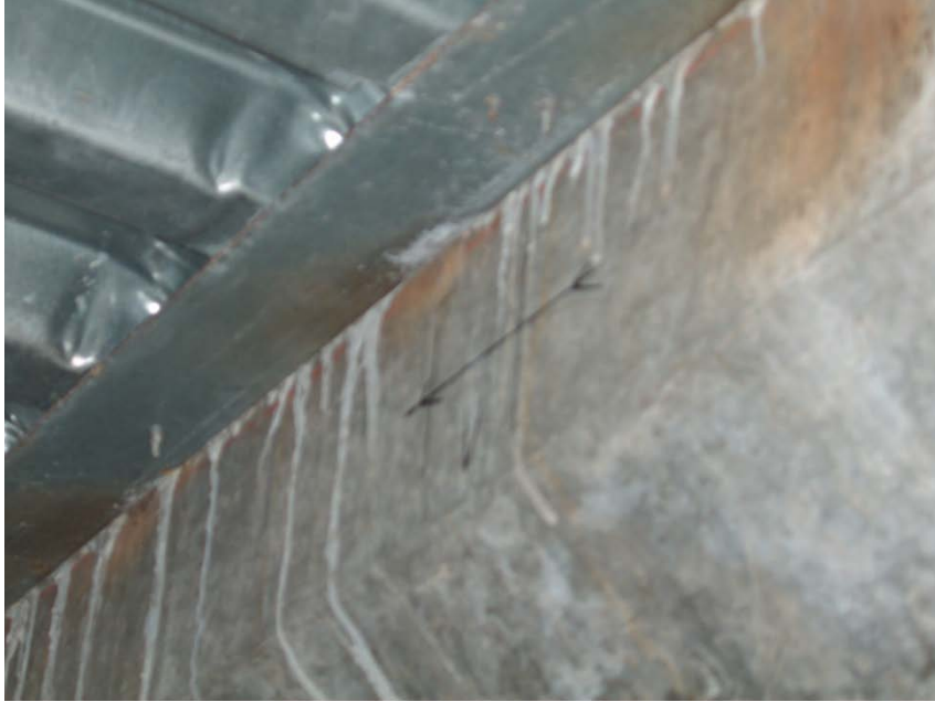
Figure 143 Initial marking on the girder for placing transducer
