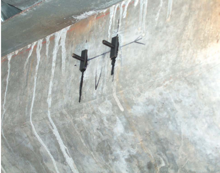
Figure 145 Tabs on the Girder 1 after removing the transducer
