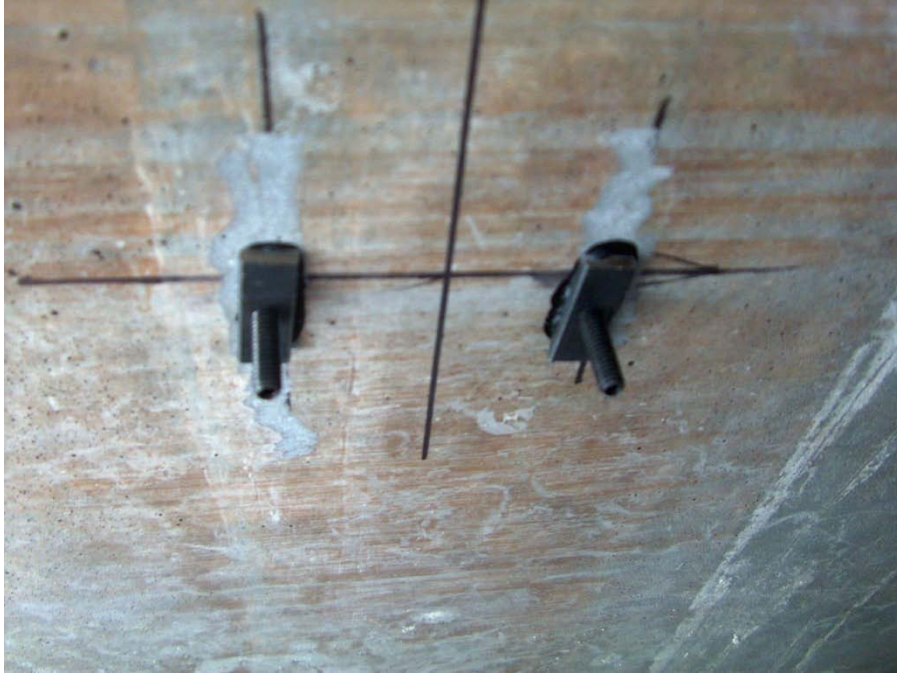
Figure 159 Tabs on the Girder 2 after removing the transducer
