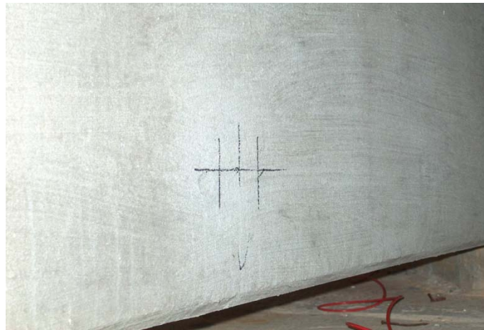
Figure 11 Marking on girder for placing of transducers
