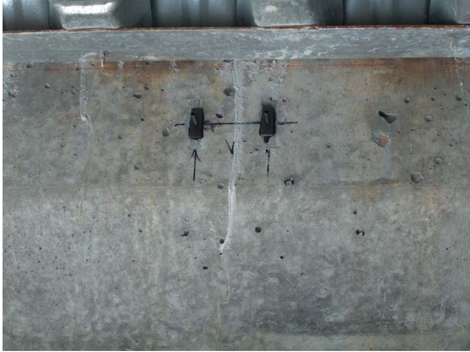
Figure 167 Tabs on the Girder 3 after removing the transducer
