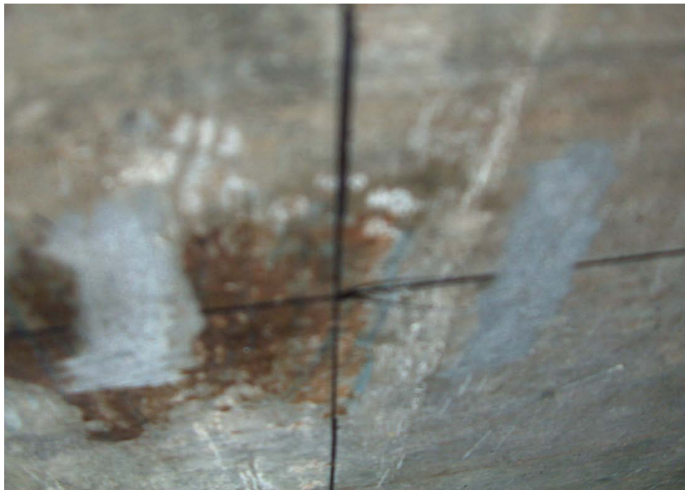
Figure 180 Initial marking on the girder for placing transducer
