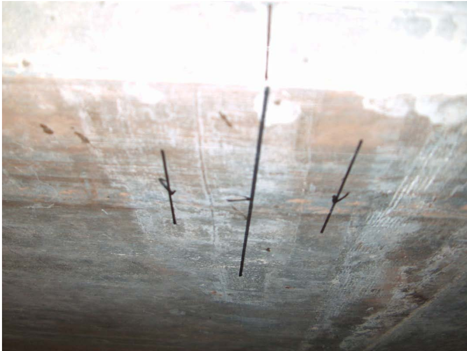
Figure 168 Initial marking on the girder for placing transducer
