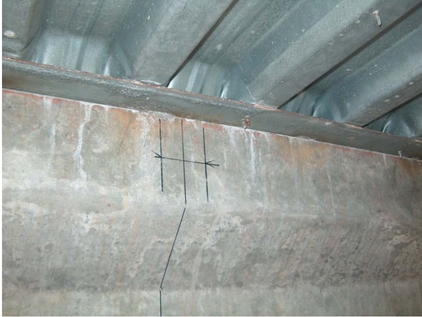
Figure 149 Initial marking on the girder for placing transducer
