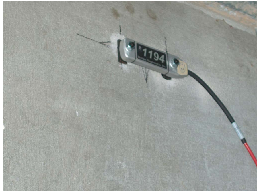
Figure 196 Gauge located on the continuity diaphragm of support Span 7-8
