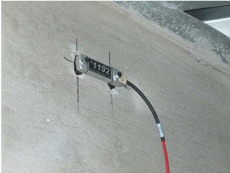
Figure 188 Gauge located on the continuity diaphragm of support Span 7-8
