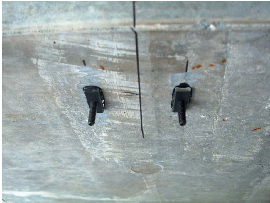
Figure 176 Tabs on the Girder 4 after removing the transducer
