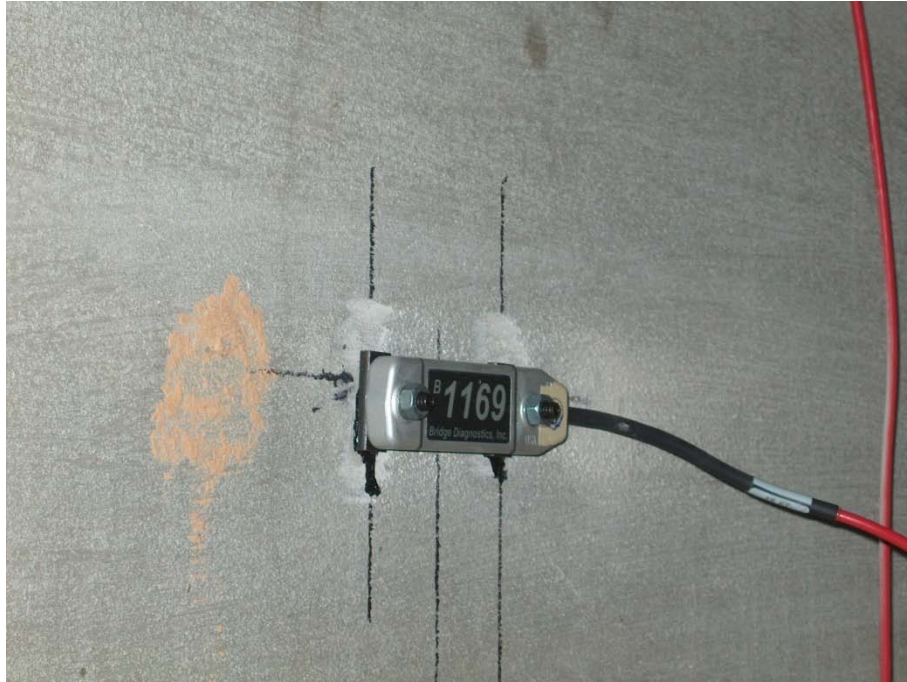
Figure 193 Gauge located on the continuity diaphragm of support Span 7-8
