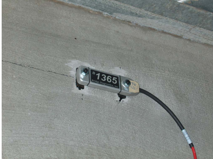
Figure 197 Gauge located on the continuity diaphragm of support Span 7-8
