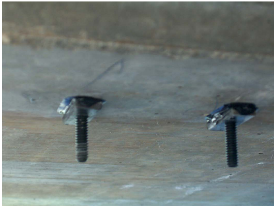
Figure 186 Tabs on the Girder 6 after removing the transducer
