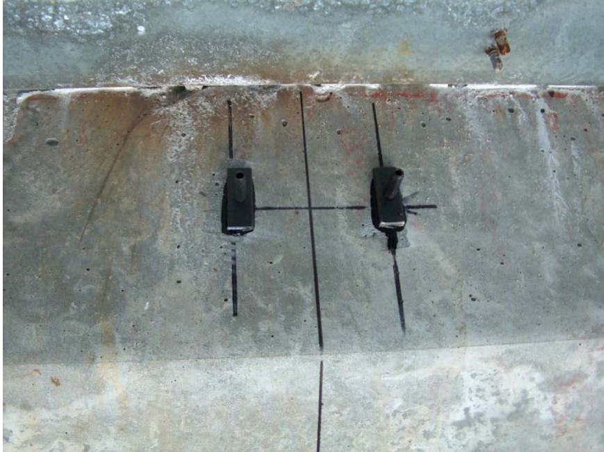
Figure 151 Tabs on the Girder 1 after removing the transducer
