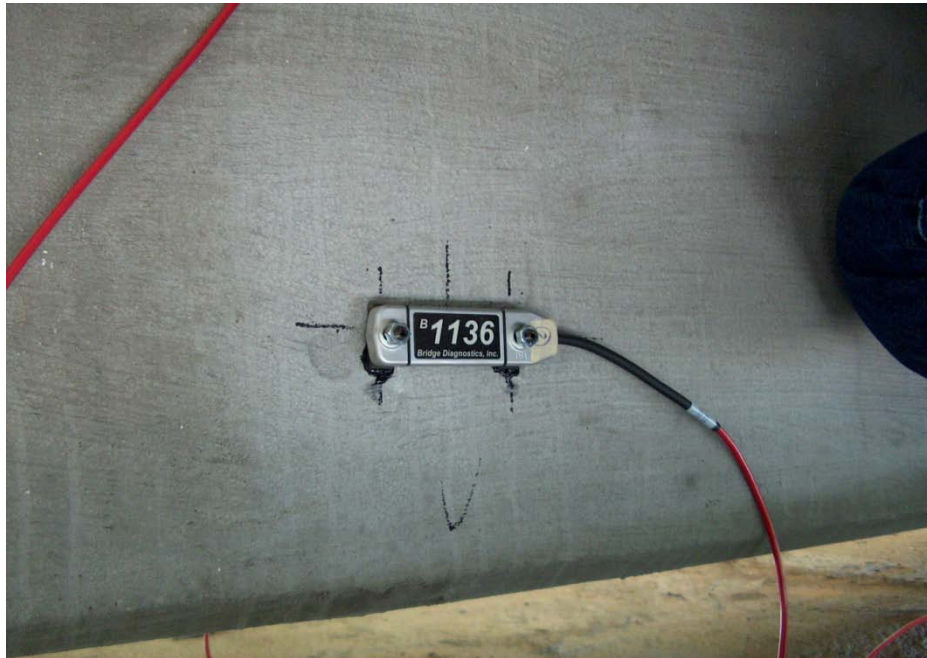
Figure 190 Gauge located on the continuity diaphragm of support Span 7-8
