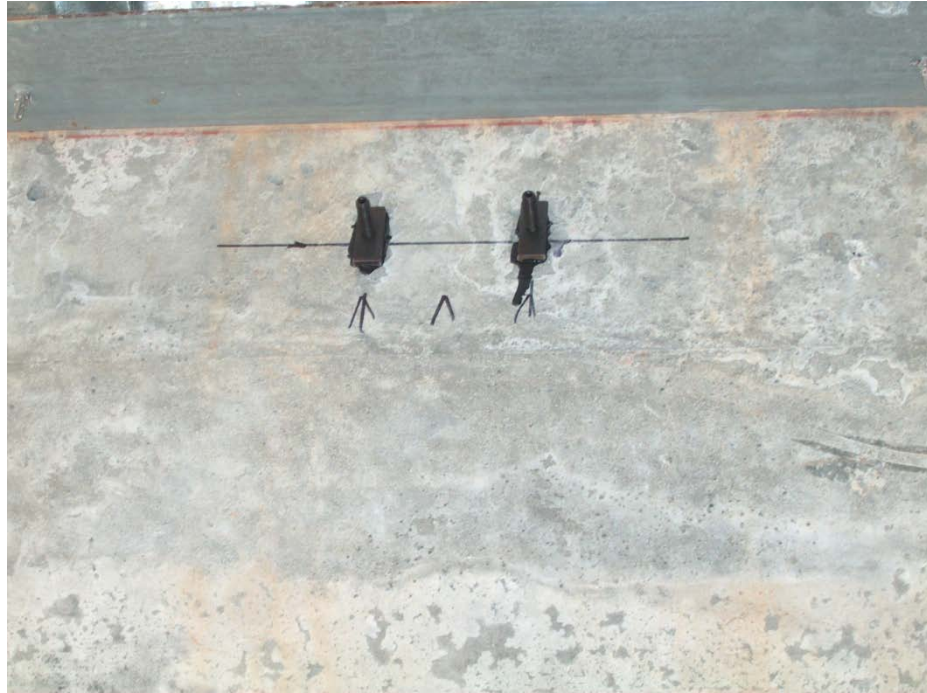
Figure 173 Tabs on the Girder 4 after removing the transducer
