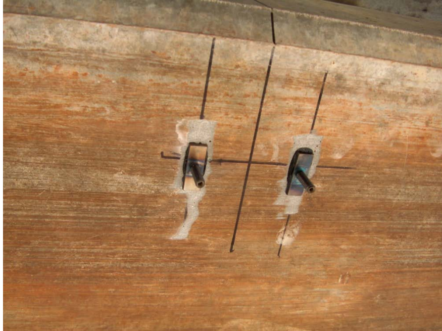
Figure 153 Tabs on the Girder 1 after removing the transducer
