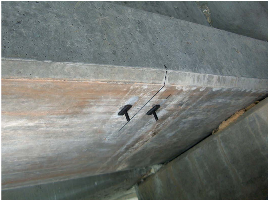
Figure 170 Tabs on the Girder 3 after removing the transducer
