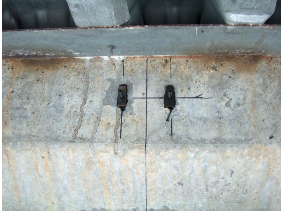
Figure 161 Tabs on the Girder 2 after removing the transducer
