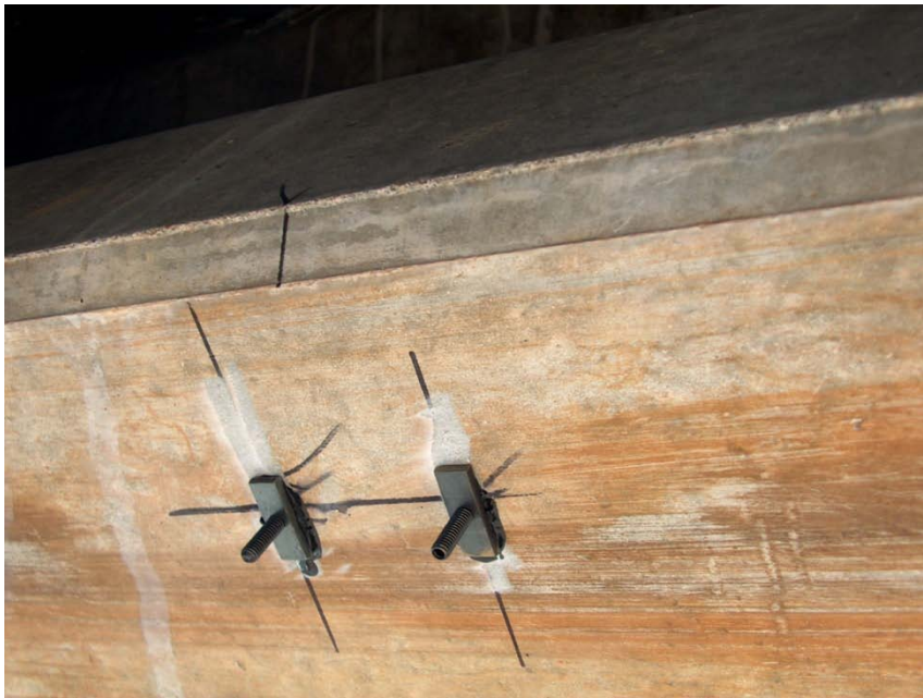
Figure 148 Tabs on the Girder 1 after removing the transducer
