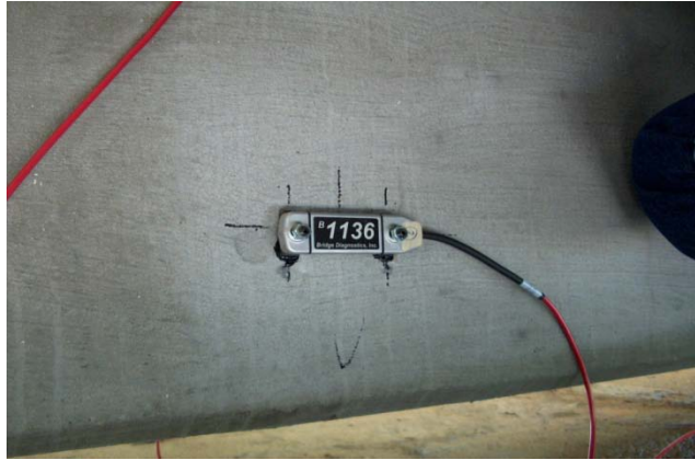
Figure 12 Fixing of transducers
