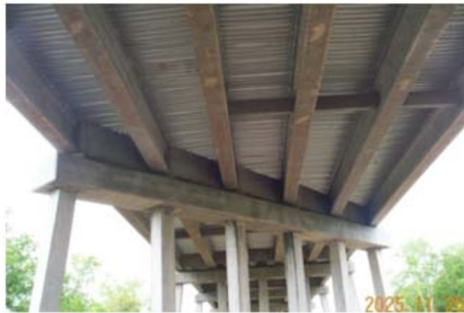
Figure 5 View of BNSF overpass
