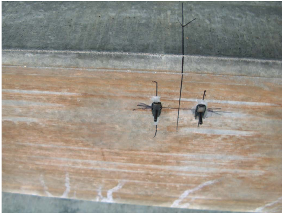
Figure 164 Tabs on the Girder 2 after removing the transducer
