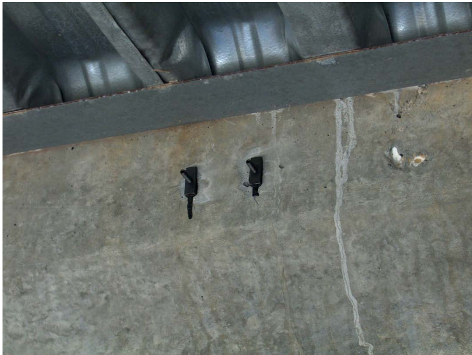
Figure 184 Tabs on the Girder 6 after removing the transducer
