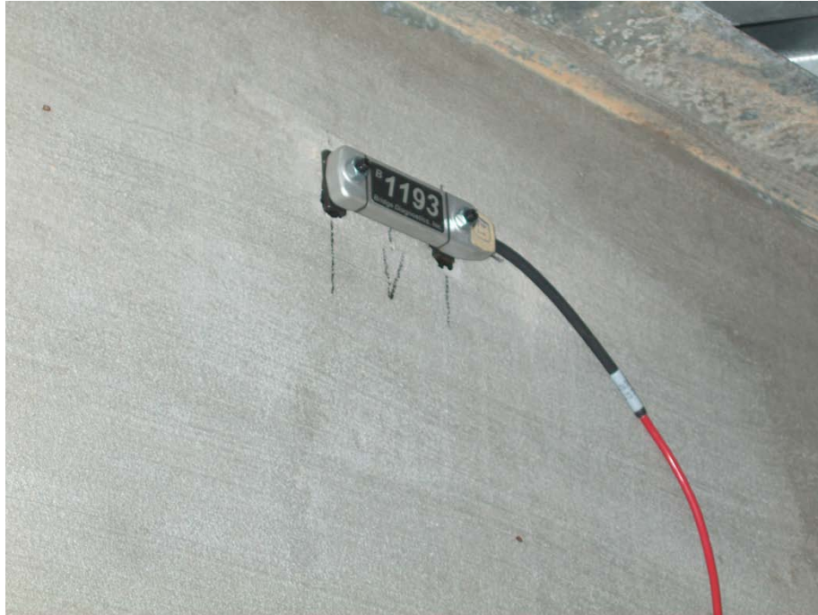
Figure 191 Gauge located on the continuity diaphragm of support Span 7-8
