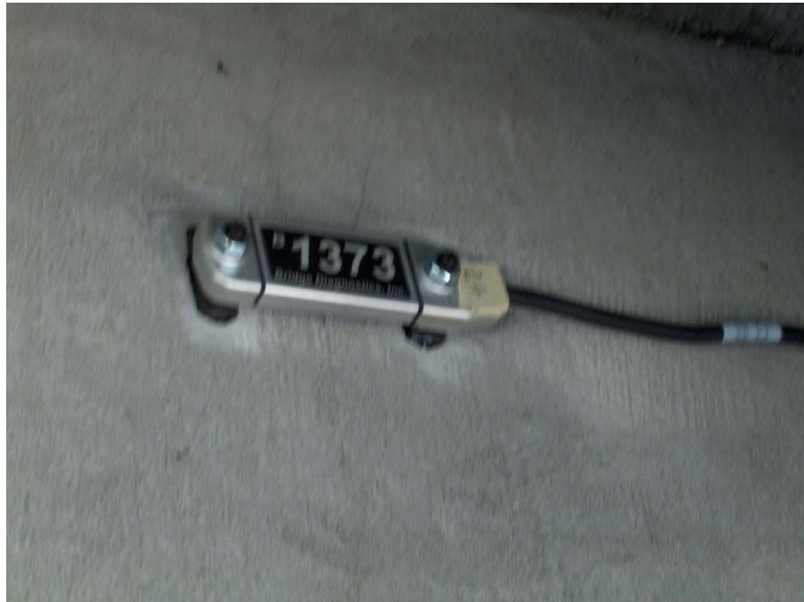
Figure 198 Gauge located on the continuity diaphragm of support Span 7-8
