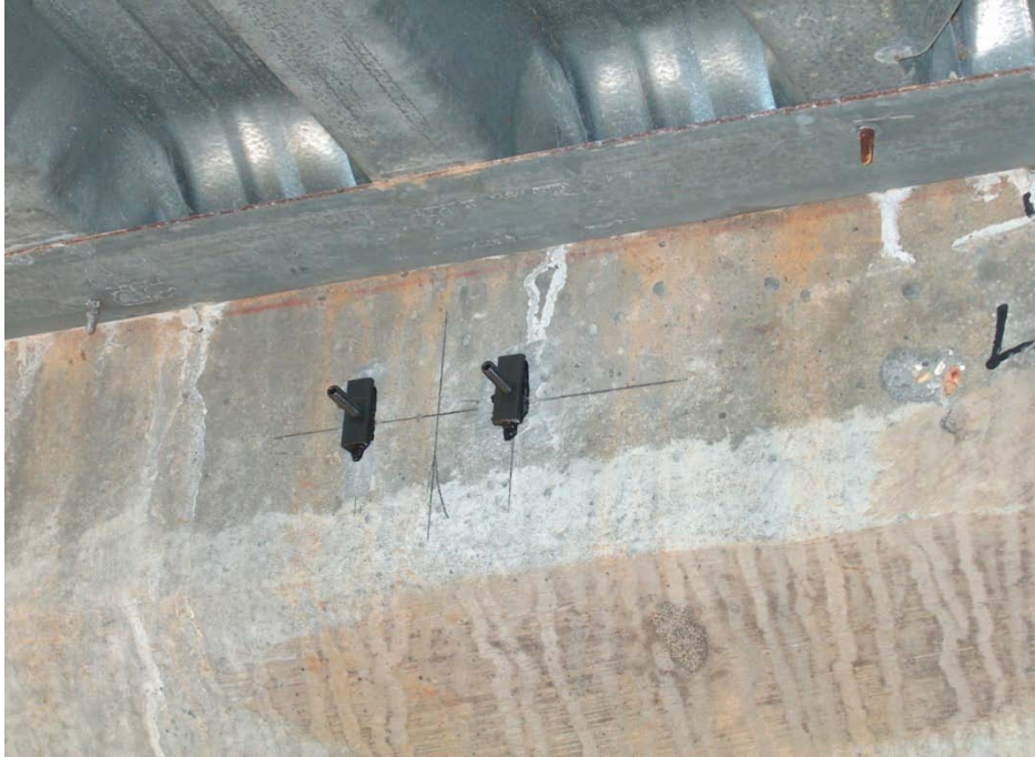
Figure 179 Tabs on the Girder 4 after removing the transducer
