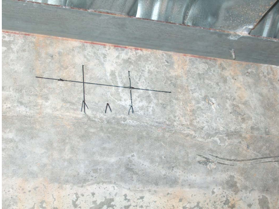
Figure 171 Initial marking on the girder for placing transducer
