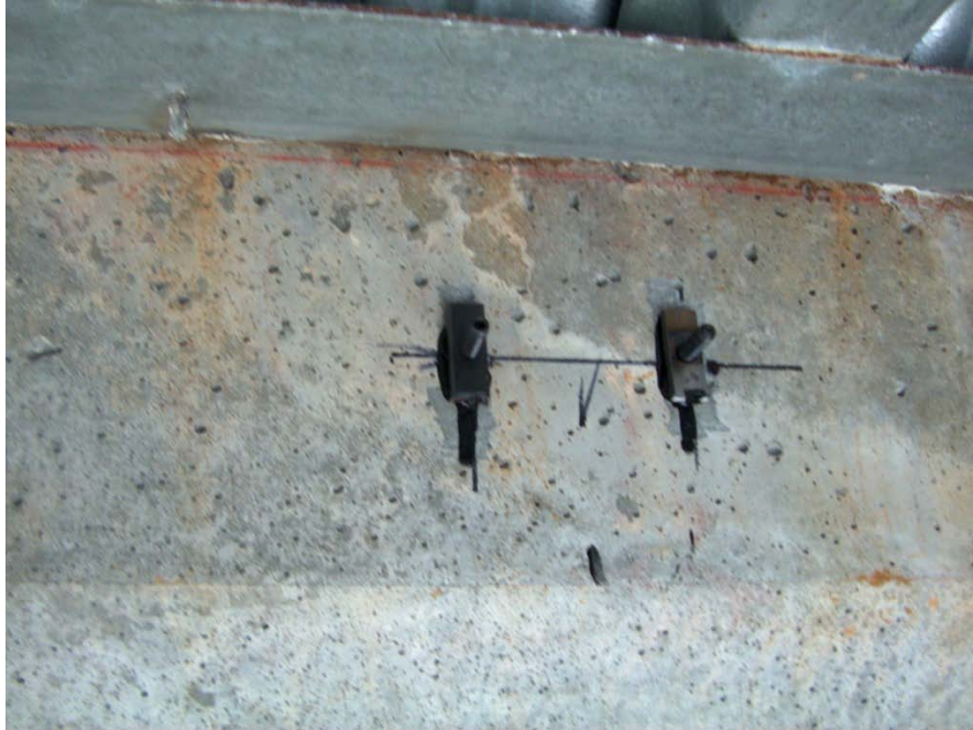
Figure 157 Tabs on the Girder 2 after removing the transducer
