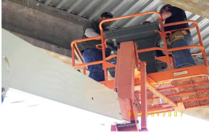
Figure 9 Superstructure accessed by JLG lift
