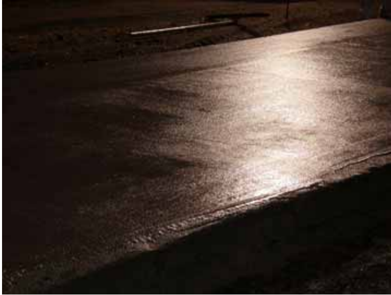
Figure B7. Concrete is eventually finished well
