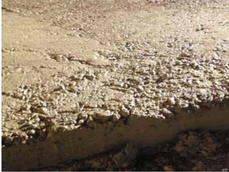
Figure B5. Dry mixture is hardly compacted behind the paving machine
